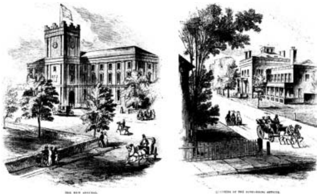
Figure 13. Left: The Main Arsenal (Building 13) as viewed from the northwest corner of the Green, 1852. (Abbott, 1852, p. 159) Right: Front façade of Commanding Officer's Quarters (Building 1), 1852. (Abbott, 1852, p. 160)
