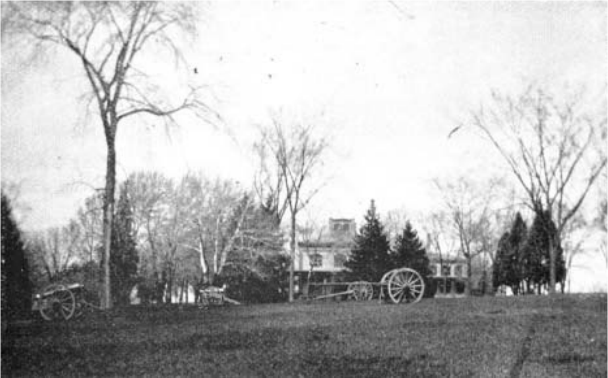
Figure 22. Lawn in front of the Commanding Officer's Quarters (Building 1) showing cannons used as a landscape feature, 1891 (Warner, 1891, p.39).
