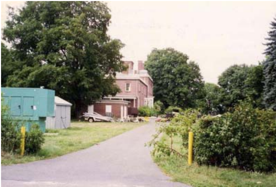
Figure 70. Small-scale maintenance related contemporary features near the driveway behind the Commanding Officer's Quarters (Building 1). To the left are the electric shed and a small storage shed. National Park Service, 2003.
