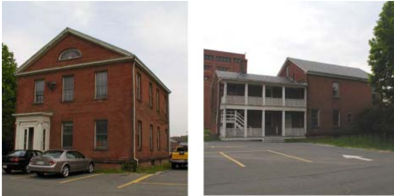
Figure 54. The west (left) and the north (right) facades of the Master Armorer's Quarters (Building 10) on the STCC property. National Park Service, 2002.
