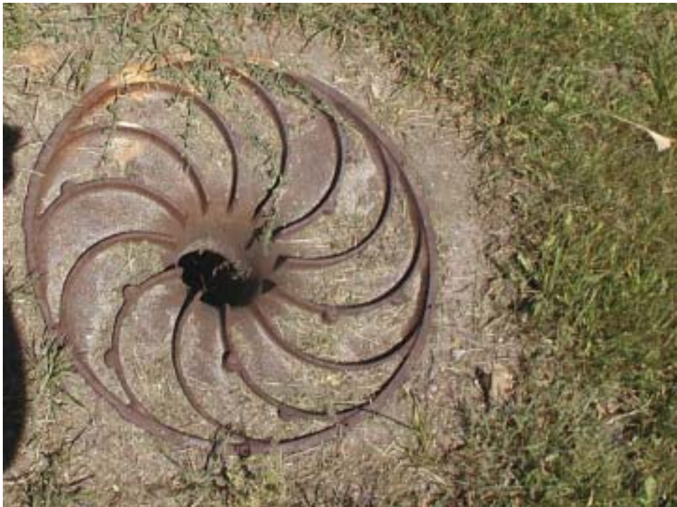
Figure 68. One type of drain inlet on the historic site. It is located on the southwest corner of the Green. National Park Service, 2003.
