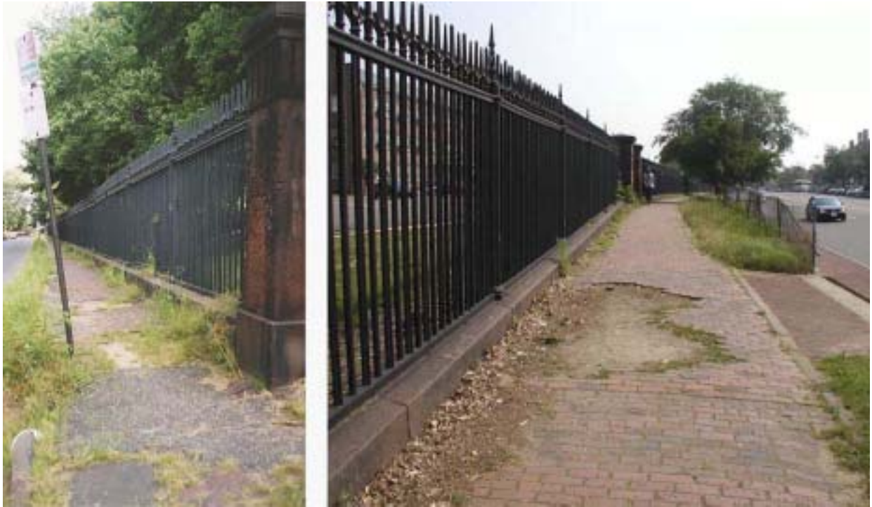
Figure 47. The brick perimeter sidewalk and fence. The sidewalks on Byers Street (left) and State Street (right) are on the city owned portion of the historic site and require stabilization and rehabilitation or restoration. National Park Service, 2002.
