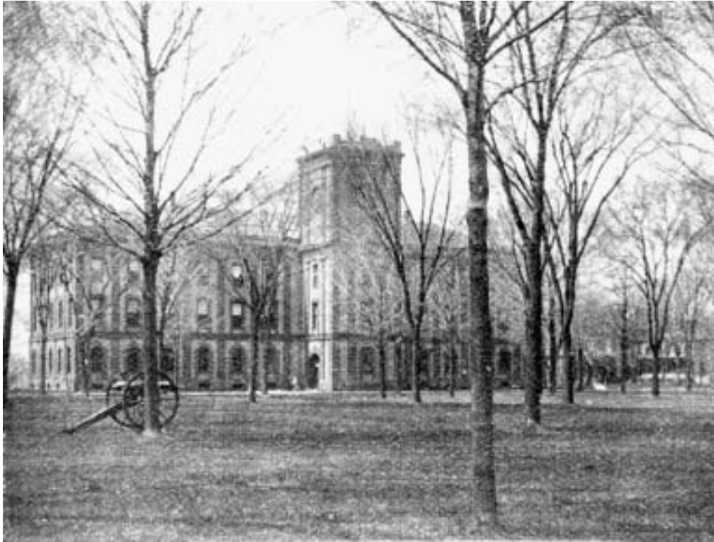
Figure 24. East façade of the Main Arsenal (Building 13) viewed across the Green showing the campus-like landscape, 1891 (Warner, 1891, p.39).
