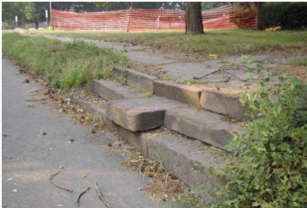
Figure 67. A mounting stone that is built into the steps between the road and the walk in front of the Officers' Quarters (Building 5 and 6, duplex). National Park Service, 2003.
