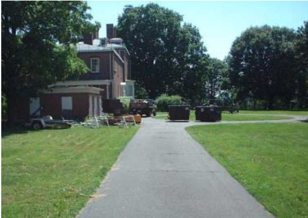
Figure 50. The driveway and circle behind the Commanding Officer's Quarters (Building 1). The Commanding Officer's Garage (Building 18) is on the left in front of the east side of the Commanding Officer's Quarters. National Park Service, 2002.
