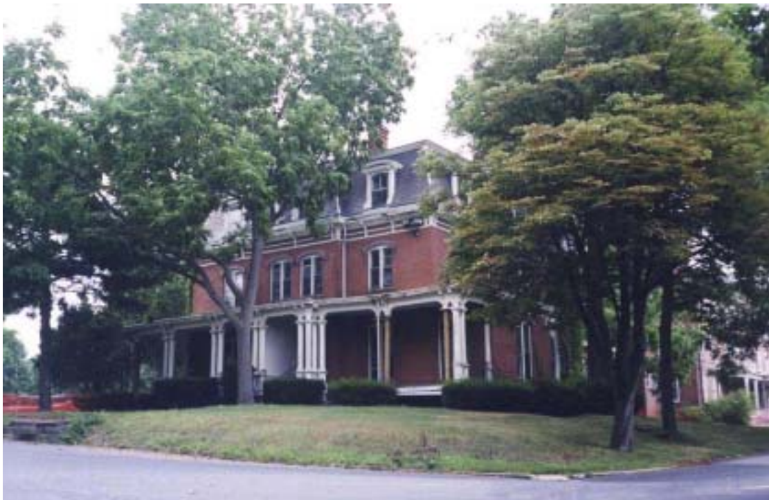
Figure 61. The Second Empire style duplex Officers' Quarters (Buildings 5 and 6) was built in 1870 and stands on the southwest corner of the Green. National Park Service, 2002.
