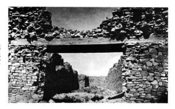
FIGURE 26 San Buenaventura in 1890 when the lintels remained over the entrance at the east, and one of the corbels under the choir loft was in place in the south wall. (Southwest Museum.)
