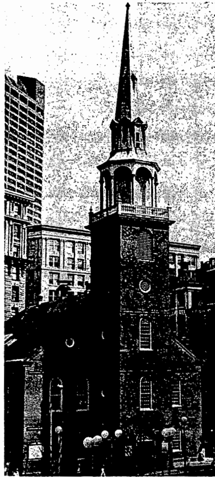
Old South Meeting House. Courtesy Massachusetts Department of Commerce and Development.
