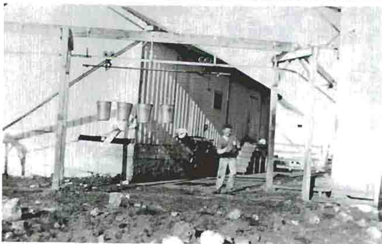
Jim McClure's tramway for hauling milk to the separator in the dairy building. Courtesy of the McClure Family.
