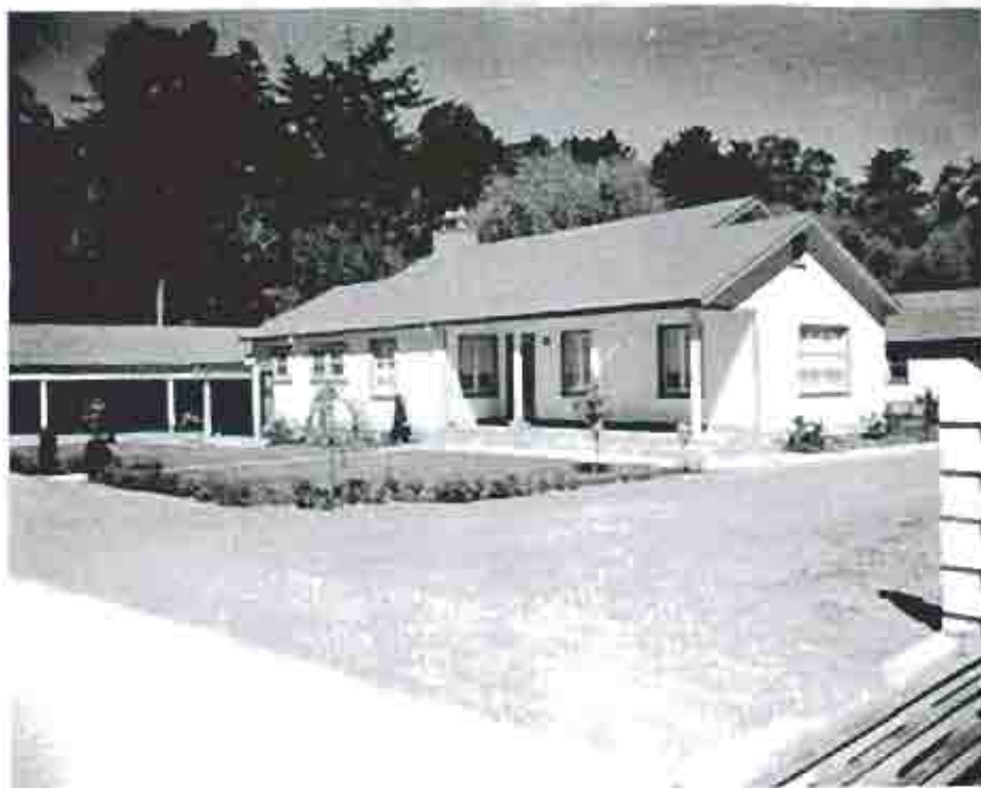
Above, the original ranch house at W Ranch in the early 1920s. Courtesy of Joan Rapp Mayhew. Left, Gene Compton built new ranch residences in the late 1940s. This is the foreman's house as it appeared when new; it is now the ranger building. Jack Mason Museum Collection.
