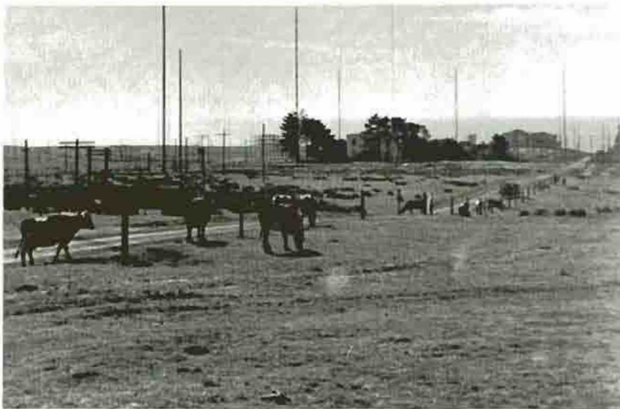
Marconi Wireless Company and RCA built this communications station on the old Nott and Ingermann Ranches early in the century. Photograph by D. M. Gunn;
