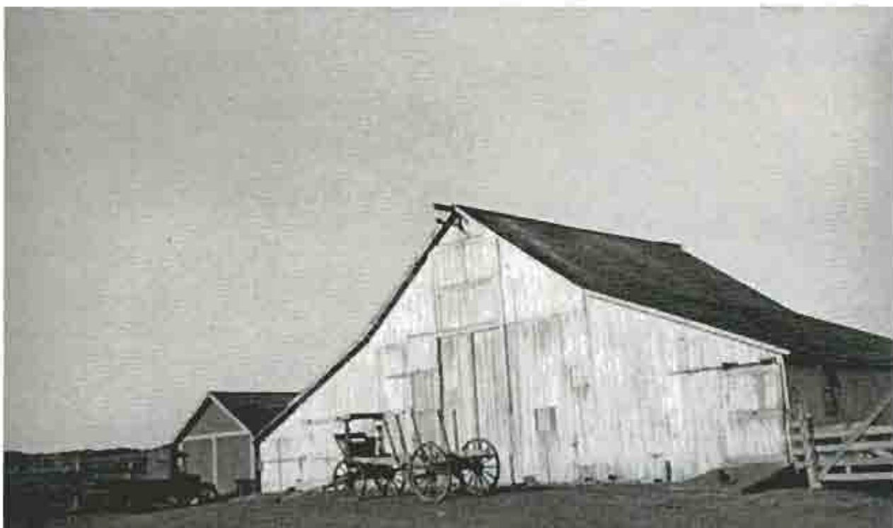
The horse barn at C Ranch, 1931, with what appears to be a wagon shed behind. Courtesy of Roy Farrington Jones.
