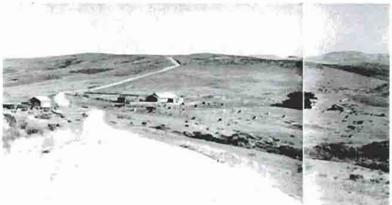
K Ranch in 1963; the large milking barn is gone, and the remaining buildings will soon be demolished by the National Park Service. Photo from an appraisal of the property.
