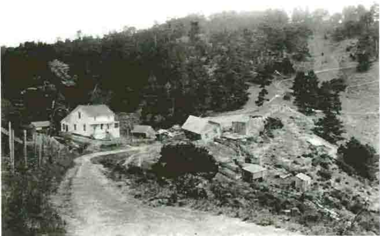
Sunnyside Ranch after the 1906 earthquake; the dairy house has fallen over. G. K. Gilbert photograph, courtesy of U. S. Geological Survey Library.
