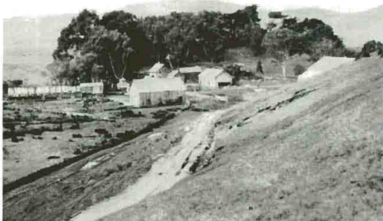
Home Ranch appears ramshackle during the waning years of Shafter ownership, in this photograph taken in 1923. The front porch of the dairy house has been altered, and a number of trees are missing. Point Reyes National Seashore Collection.
