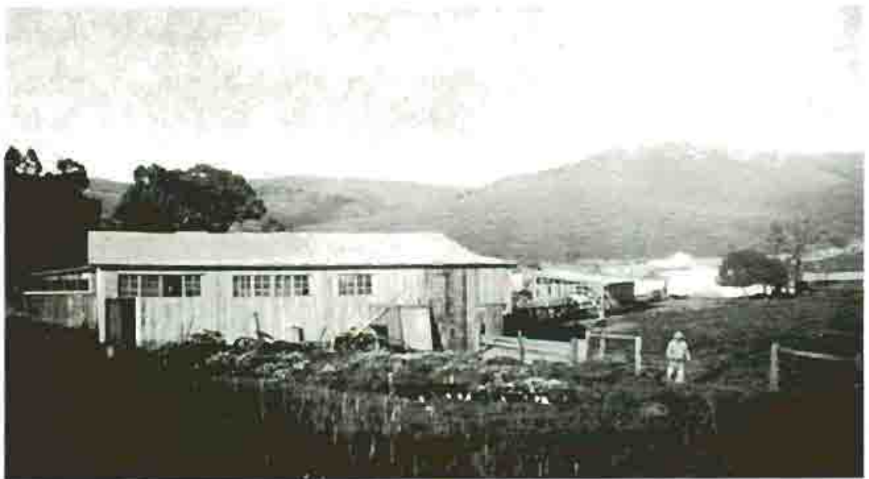
The Home Ranch shop appears in the foreground in this late 1930s photograph. The garage is under construction in the distance. Courtesy of Margaret Wosser Dowd.
