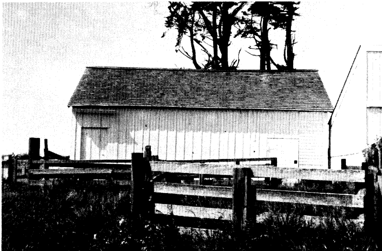
Figure 45. Looking west at the Calf Shed. This building was fully stabilized in 1984 after severe storm damage the previous winter.
