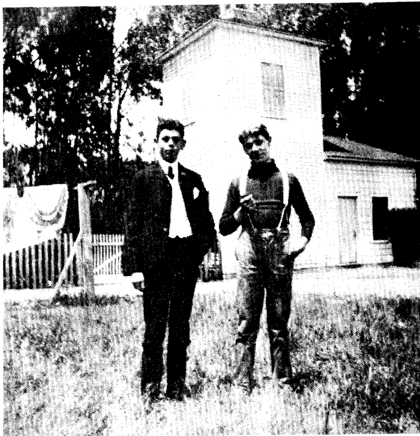
Figure 14 - The "Tank House" stands behind two unidentified young men, c. 1903. Today, the second story portion is gone, along with the cupola containing the bell. For details of the cupola, see Figures 5 and 16, and to compare with its present appearance, see Figure 37. Note fences, trees, grass, and clotheslines. Collection of Katie Bates.
