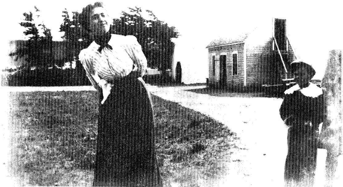
Figure 24 - Behind school teacher Martha Thompson and two of her students are the whitewashed Blacksmith Shop and the gable-roofed Carpenter Shop with the stairway at the end, and an unidentified building at right, west of it. Behind the trees at left is the Dairy (Cow) Barn, c. 1902. Collection of Katie Bates.
