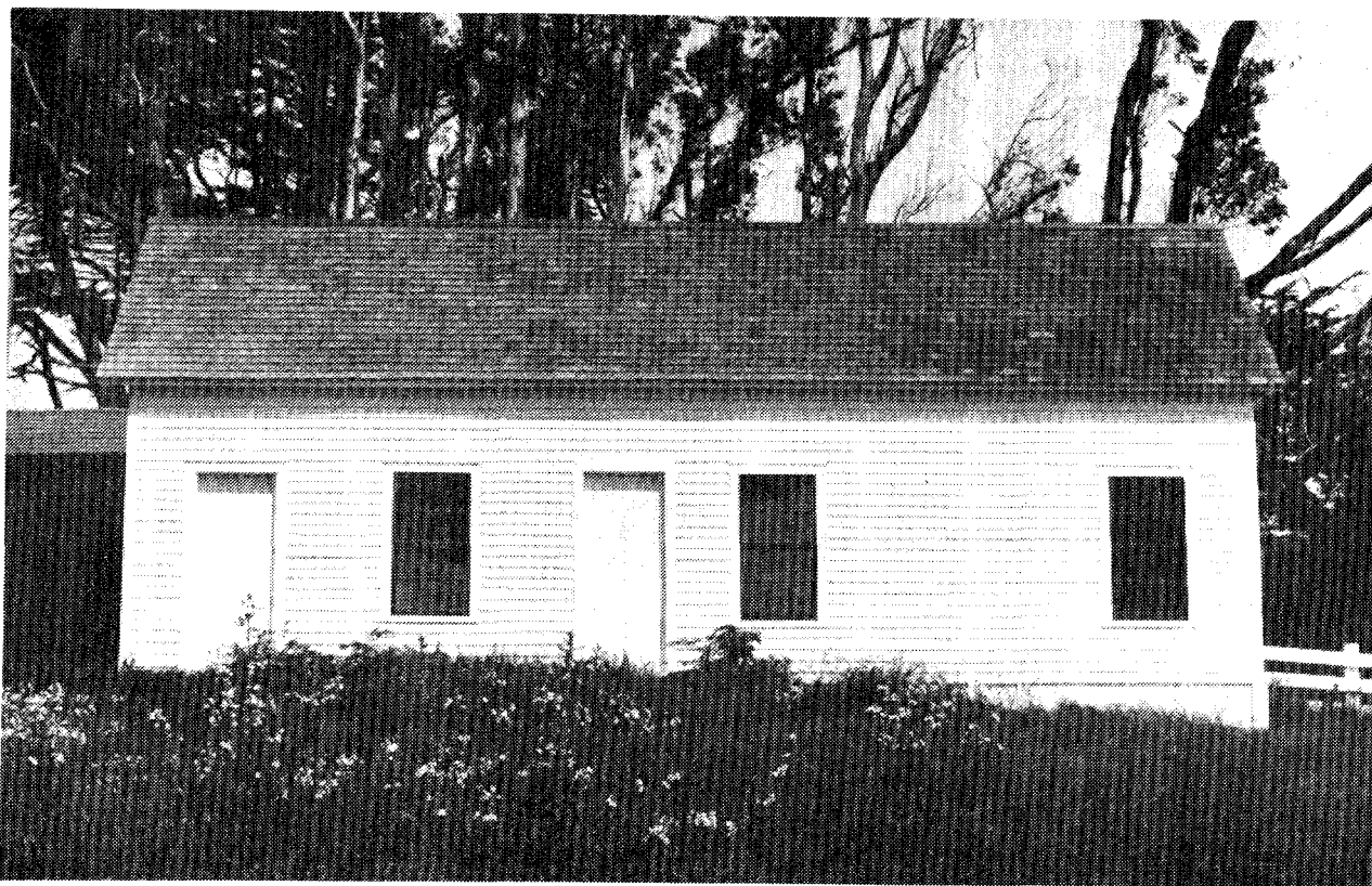
Figure 40. Looking north at the School House. Note: This building has been stabilized.
