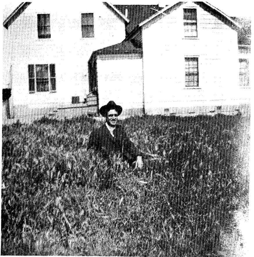
Figure 8 - The west side of Pierce Ranch House shows the contrast between the larger portion believed built in 1869, at left, and the much smaller residence believed to date from the 1850s and to have faced to the west. This latter became an annex to the 1869 house. This view dates from about 1903. Collection of Katie Bates.
