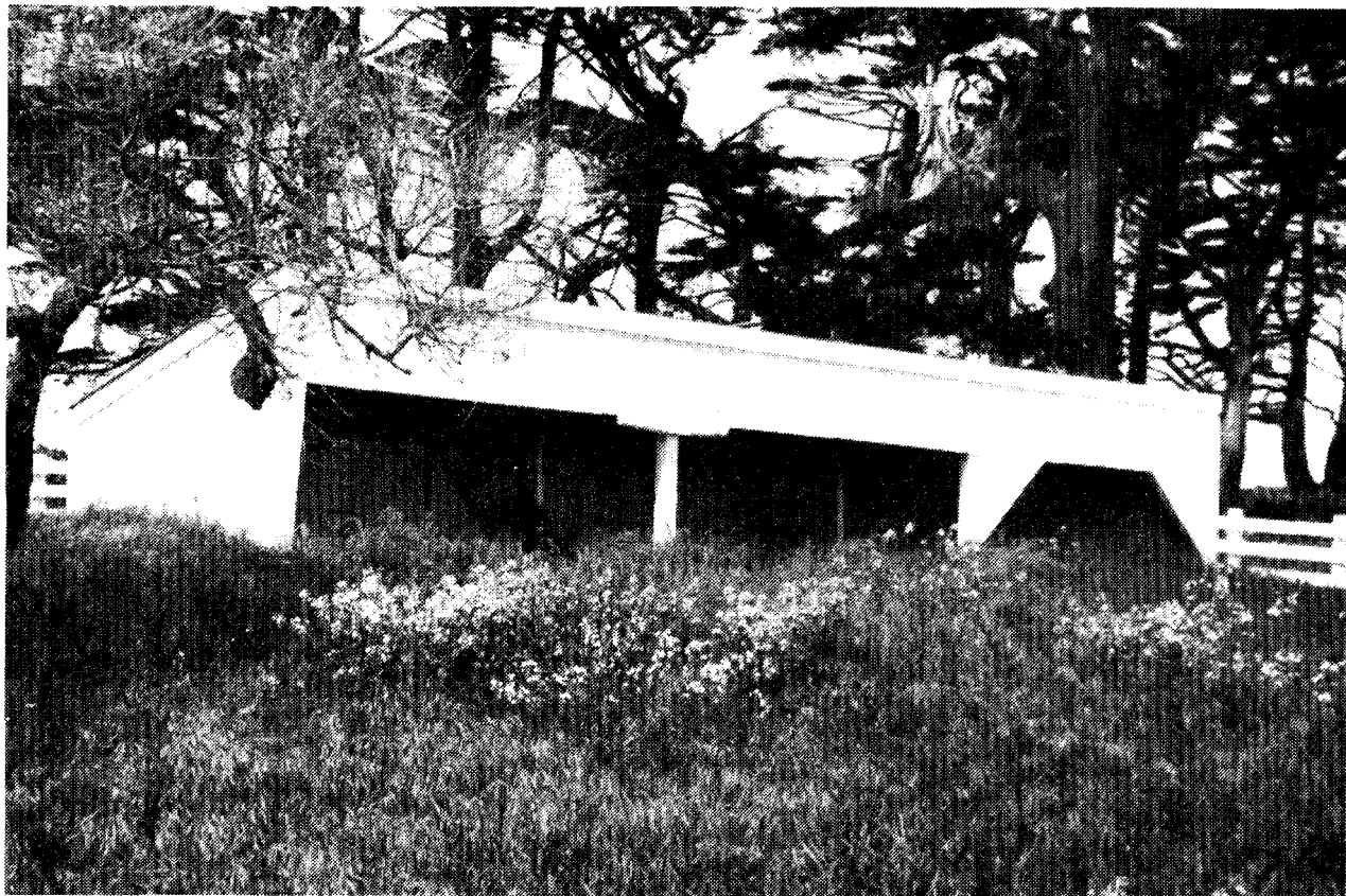
Figure 42. Looking northwest at the Open Front Shed. Note: This building was reconstructed using some of the original siding after severe storm damage in 1983.
