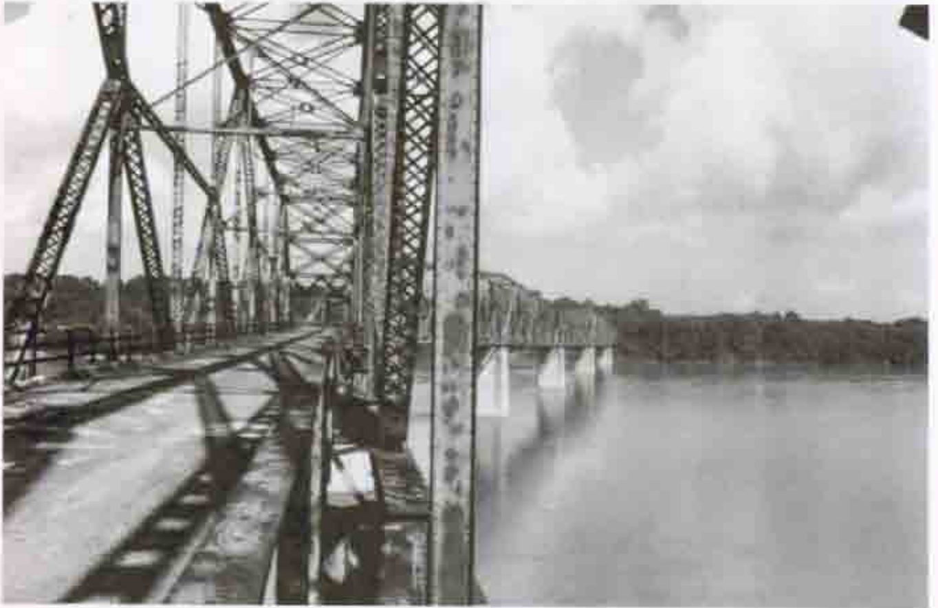
St. Louis, Missouri — Chain of Rocks Bridge
