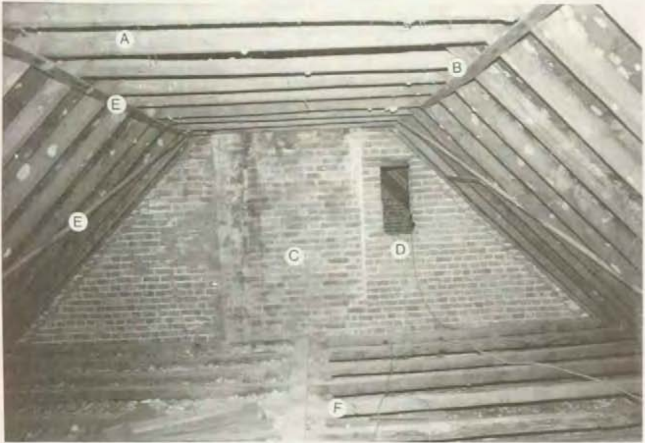
62 B ATTIC - NORTH ELEVATION OF CA. 1725 HOUSE
