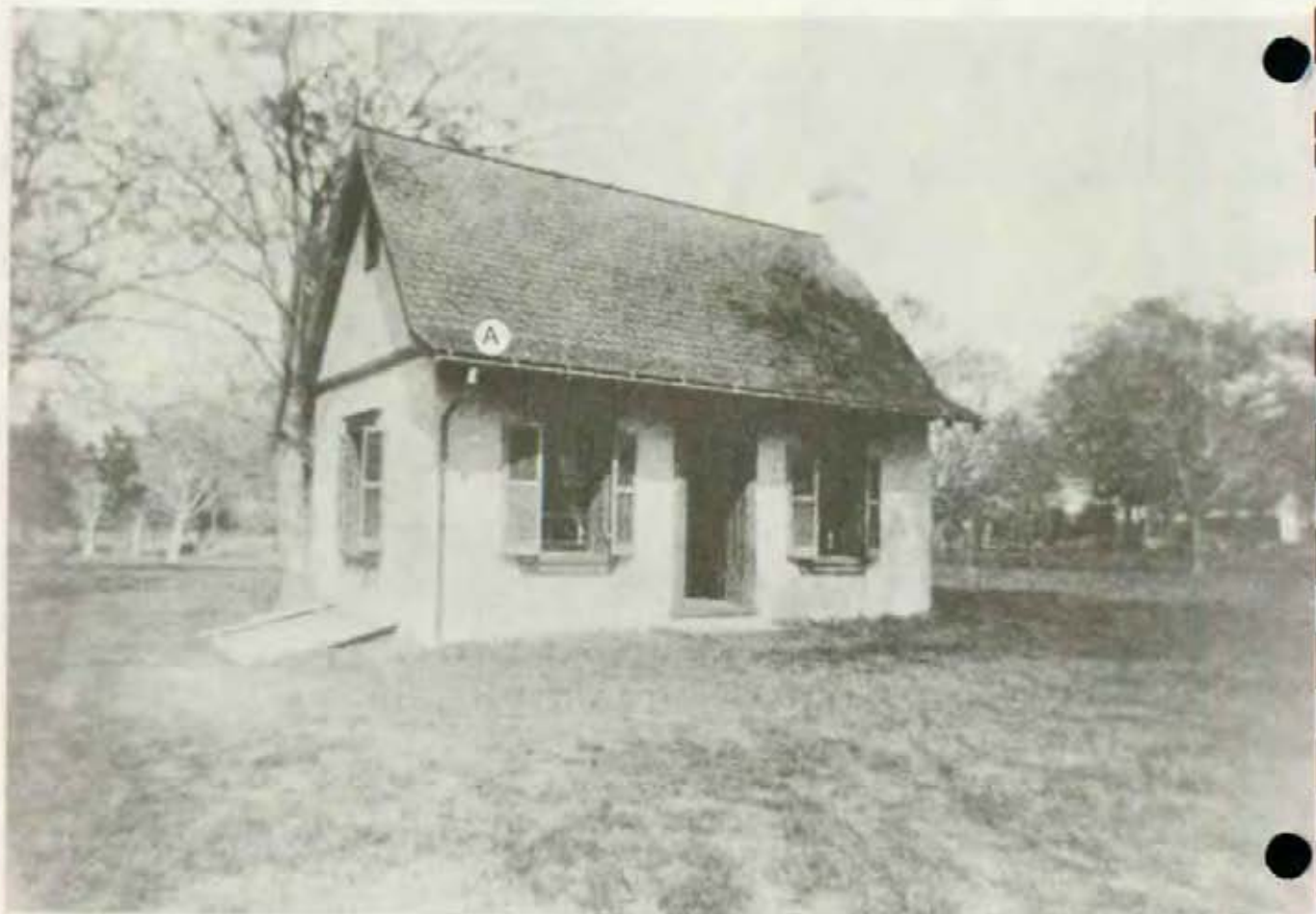
5 SOUTH ELEVATION - OUTBUILDING (CONSTRUCTED C. 1760) A
