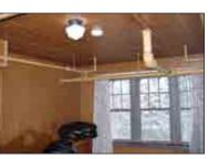
Figure 4.22: Exposed Sprinkler Piping in Guest Room
