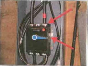
Component Right phase line side wire lug connection or internal problem in circuit breaker Probable Cause Loose corroded or Internal problem
