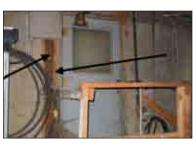
Figure 4.2: Third Basement Stairway Fire Separation Deficiencies
