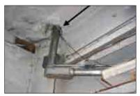
Figure 4.1: Third Basement Ceiling Penetrations
