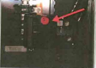
Component Upper phase heating possible internal problem in circuit breaker #24,26,28,30 sub prt upstairs Probable Cause Internal problem
