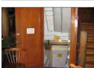
Figure 4.6: Non-Rated Enclosure to Second Basement
