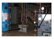
Figure 4.3: Close Proximity of Propane HW Heater and Boiler Burner
