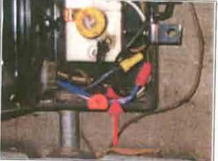
Component Load side red wire nut connetion on purple wire below fused disconnect switch Probable Cause Loose or corroded wire nut
