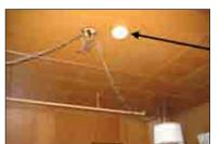
Figure 4.18: Typical Battery Powered Guest Room Smoke Detector (Note: This is not connected to the building alarm system.)
