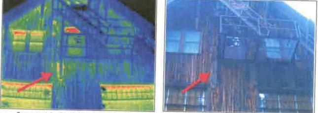
Component Small temp difference around north 2nd floor mounting bracket of fire escape, possible moisture problem or other an Probable Cause Possible moisture or other anomole
