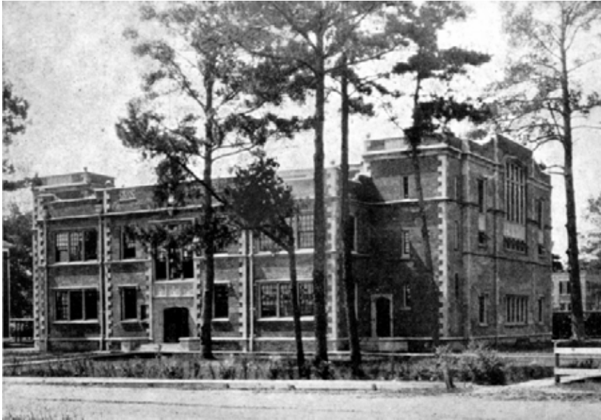
Figure 11. Front (north) façade of Women's Gymnasium showing pine trees and hedges and walkways along College Avenue, 1927. Note the former neighboring building at the far left.(Northwestern State University, Watson Memorial Library, Cammie G. Henry Research Center (Potpourri Yearbook)).
