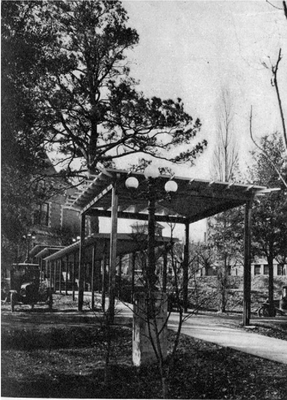
Figure 14. Walkway from Main Gate to Normal Hill lined with electroliers, and ornamental vegetation including the "Sentinel Pine" (top center) and sheltered with pergolas, 1924 (Northwestern State University, Watson Memorial Library, Cammie G. Henry Research Center (Potpourri Yearbook)).
