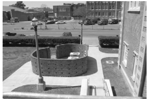
Figure 60. The southwest brick utility pod and part of the ADA-compliant ramp as seen from the steel staircase (OCLP, 2004).
