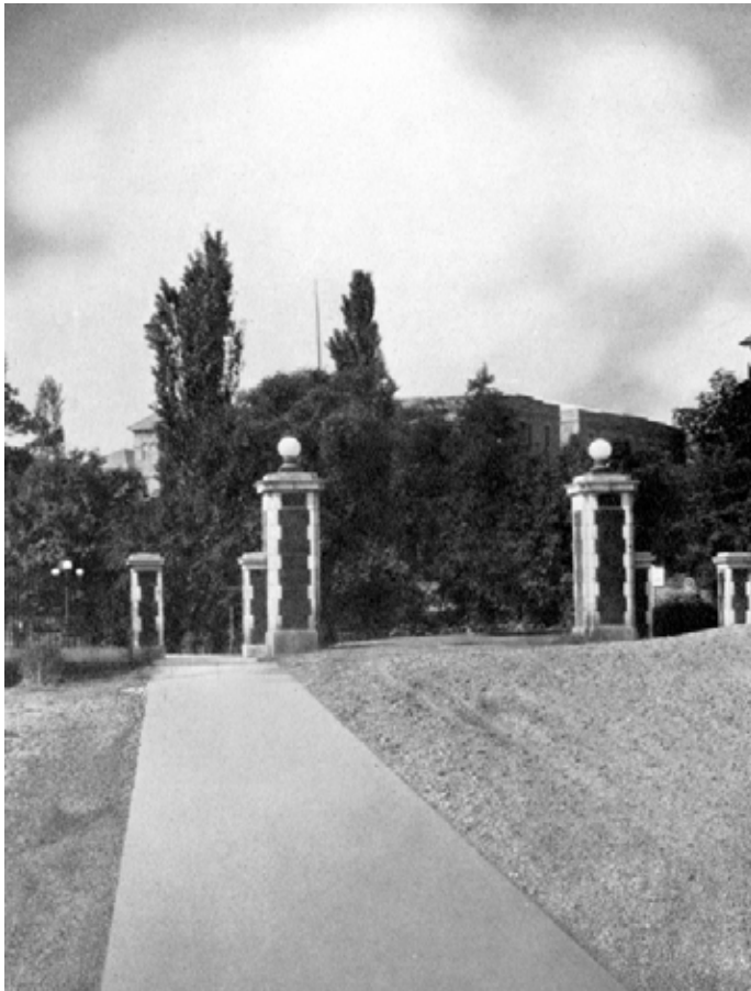
Figure 16. Main Gates along College Avenue, 1928 (Northwestern State University, Watson Memorial Library, Cammie G. Henry Research Center (Potpourri Yearbook)).
