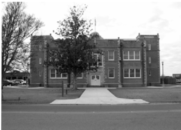
Figure 56. Front façade and north lawn of Nelson Hall as seen from College Avenue (OCLP, 2004).
