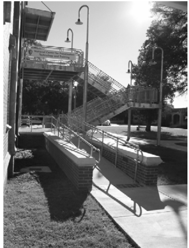
Figure 64. Accessibility ramp leading to Nelson Hall's main (south) entrance landing beneath the steel staircase (OCLP, 2004).
