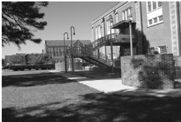
Figure 59. The steel staircase flanked by two brick utility pods along the south façade of Nelson Hall (OCLP, 2004).
