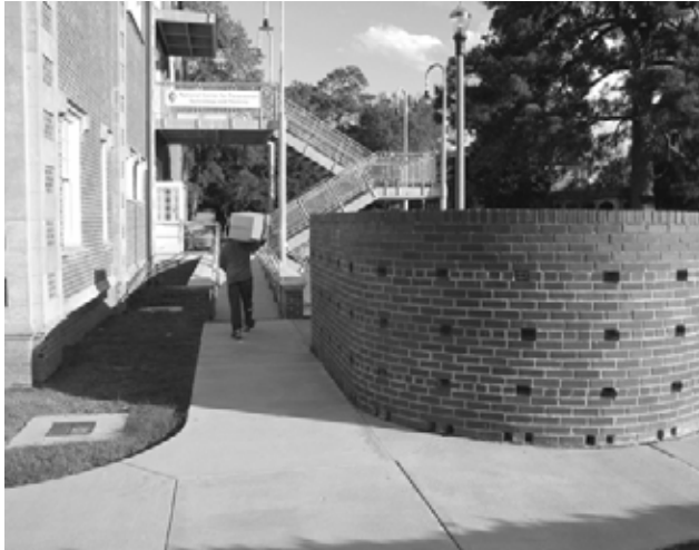
Figure 63. Walkway from Caspari Street parking area to Nelson Hall's current main entrance pinched between the building's south façade and a brick utility pod (OCLP, 2004).
