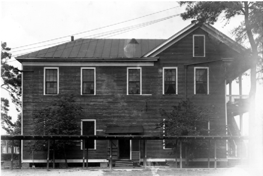
Figure 30. The old Fine Arts building formerly located in the vicinity of Horseshoe Drive east of the Women's Gymnasium, c. 1939 (year of demolition). The pergola-covered walkway in the foreground lead to Normal Hill (Northwestern State University, Watson Memorial Library, Cammie G. Henry Research Center (Potpourri Yearbook)).
