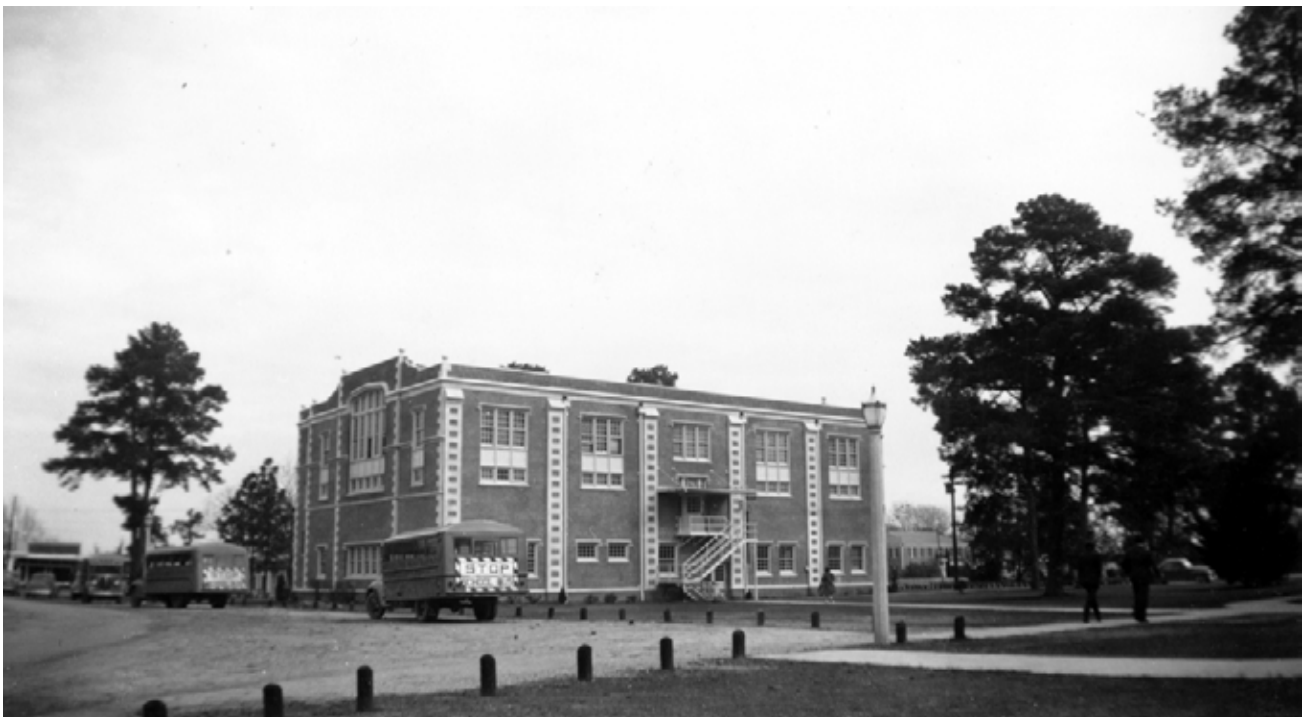
Figure 34. South lawn of the Women's Gymnasium, 1941 (Northwestern State University, Watson Memorial Library, Cammie G. Henry Research Center (1941 Booklet-Insurance of Campus Buildings)).
