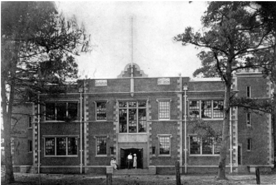
Figure 8. Front (north) façade of Women's Gymnasium showing pine trees, 1924 (Northwestern State University, Watson Memorial Library, Cammie G. Henry Research Center (Potpourri Yearbook)).
