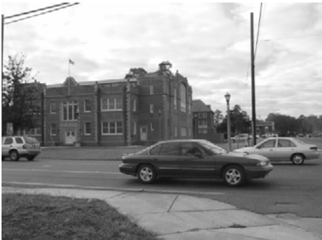
Figure 61. Heavy traffic on College Avenue (LA Route 6) at the intersection with Caspari Street. Nelson Hall with the Caspari Street perpendicular parking spaces to the right are in the background (OCLP, 2004).
