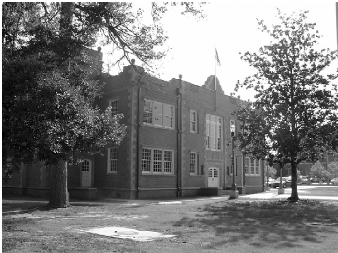
Figure 52. North lawn of NCPTT's Nelson Hall (former Women's Gymnasium), c. 2001 (NCPTT).
