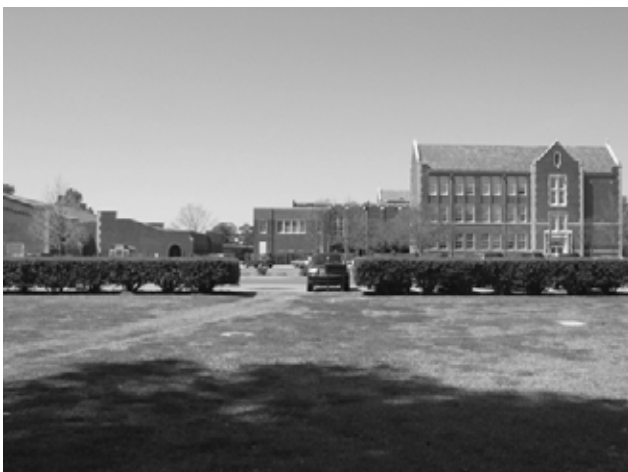
Figure 69. Waxleaf privet hedge between south lawn and Caspari Street parking area with gap in the center (OCLP, 2004).
