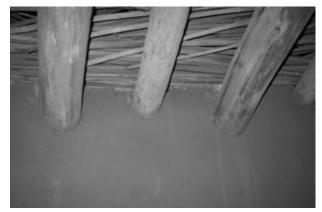
FIGURE 108. View of intersection of rafters and clay wall. (NPS-SERO-CR, 2004)
