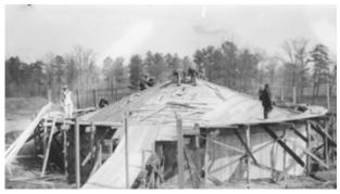
FIGURE 33. View of completed form for roof, March 1, 1937. (Swanson, OCMU Coll.)
