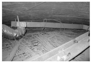
FIGURE 109. View of cane matting above main roof. Note sawn batten spiked to rafter to hold cane in place. (NPS-SERO-CR, 2004)
