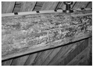
**FIGURE 112.** View of north beam with typical mold growth. (NPS-SERO-CR, 2004)
