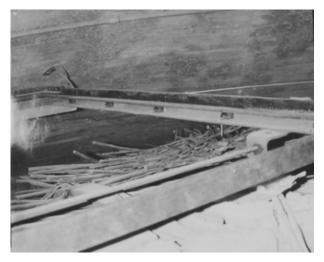
FIGURE 75. View of inside of concrete shell above lodge ceiling, 1974, showing part of original track installed for retracting skylight in 1937. (OCMU Coll.)
