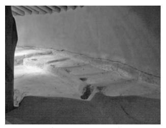
FIGURE 96. View of seats on northeast side of lodge, with highest surviving portion of encircling wall. Whitish band at base of wall is mold. (NPS-SERO-CR, 2004)
