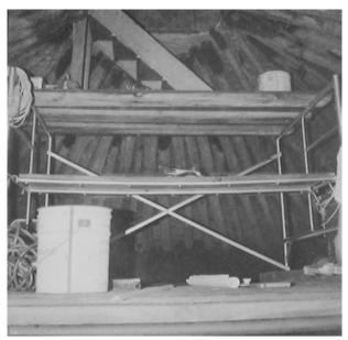
FIGURE 73. View of scaffolding erected in April 1975 for work on interior of concrete shell. (OCMU COII.)
