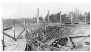
FIGURE 30. View of Earth Lodge, February 2, 1037, with north half of wall complete and rebar in place for south half. (Swanson, OCMU Coll.)
