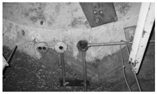
**FIGURE 117.** View at top of inside of concrete shell, showing remnants of 1937 electrical system and of white paint applied to improve the day-light effect of the original lighting. (NPS-SERO-CR, 2004)
