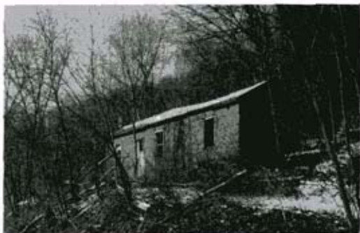
FIG. 15. ABANDONED WORKER'S HOUSE, VILLAGE OF PARKS QUARRIES. PHOTOGRAPH BY ALLISON RACHLEFF.
