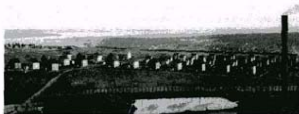
FIG. 1. T-PLAN HOUSES BUILT 1899-1900 AND 2-1/2-STORY BEARS ROEBUCK HOUSES BUILT 1918 BY QUINCY MINING COMPANY, PEWABIC, MICHIGAN. UNDATED PHOTOGRAPH, MTU ARCHIVES.
