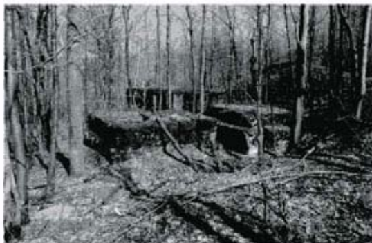
FIG. 5. FOUNDATIONS, MINE VENTILATION SYSTEM. DOLPH/SUNNYSIDE INDUSTRIAL DISTRICT. PHOTOGRAPH COURTESY OF CHRIS, INC., NORTH WALES, PA.
