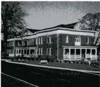
FACING THE CAMPUS ROAD
