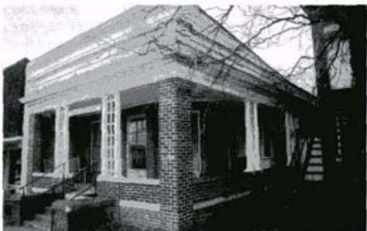
FIG. 1. LADIES REST ROOM, LEWISBURG, TN. PHOTOGRAPH COURTESY OF CARROLL VAN WEST.
