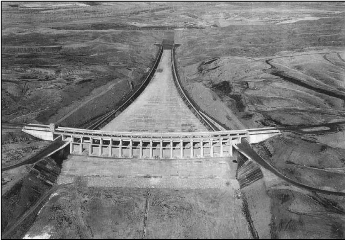
Figure 6-4: The spillway gate structure and concrete lined canal at Fort Peck. Source: Records of the U.S. Army Corps of Engineers, Record Group 77, National Archives and Records Administration, College Park, Maryland.
