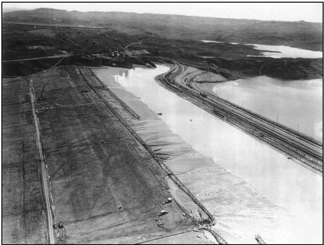
Figure 6-8: The completed east section of Fort Peck Dam before the slide. Hydraulic fill material was discharged through traps in the bottom of the dredge pipe. As the fill rose, the rail lines at the upstream edge (right) were relocated at higher levels to provide for placing the blanket of gravel and protective stone. June 29, 1938. Source: Records of the U.S. Army Corps of Engineers, Record Group 77, National Archives and Records Administration, College Park, Maryland.
