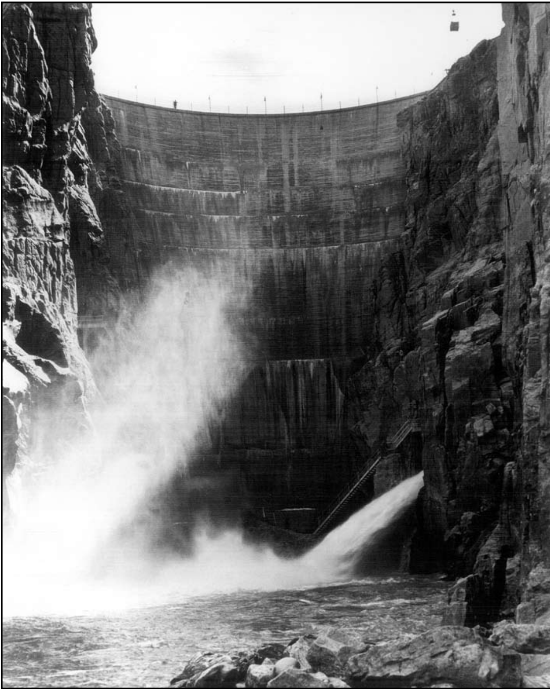
Figure 2-9: In 1910 the Bureau of Reclamation completed Buffalo Bill Dam on the Shoshone River near Cody, Wyoming. This constant radius concrete arch dam is 325 feet high. The dam delivers irrigation water and has a powerplant. Source: Bureau of Reclamation.
