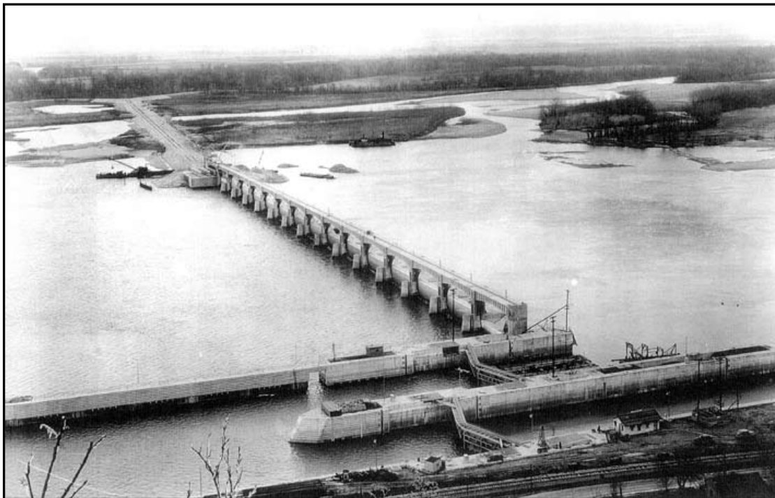
Figure 8-13: Mississippi River Dam #24. Source: Records of the U.S. Army Corps of Engineers, Record Group 77, National Archives and Records Administration, College Park, Maryland..
