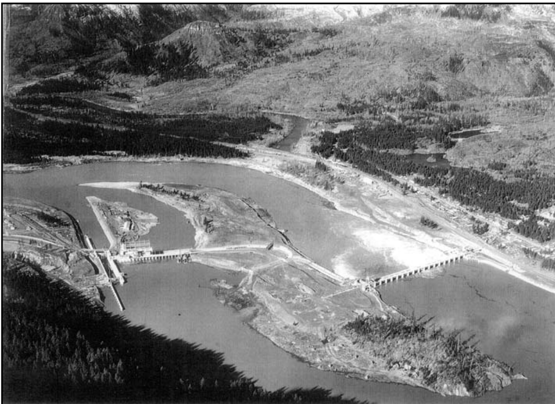
Figure 5-7: At Bonneville Dam the locks and powerhouse are on the left, Bradford Island is in the middle, and the main spillway dam is on the right. Source: Records of the U.S. Army Corps of Engineers, Record Group 77, National Archives and Records Administration, College Park, Maryland.
