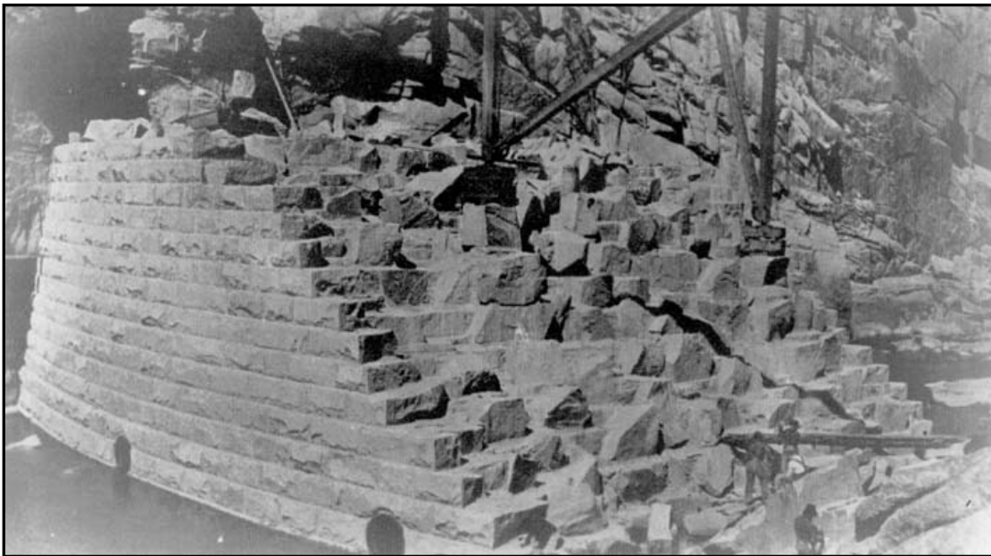
Figure 2-7: Pathfinder Dam was constructed with huge blocks of stone. Source: Bureau of Reclamation
