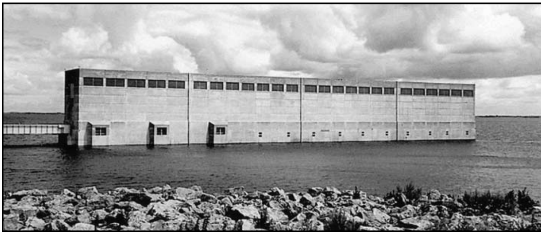
Figure 6-27: Water intake structure at Garrison Dam. Source: David P. Billington.
