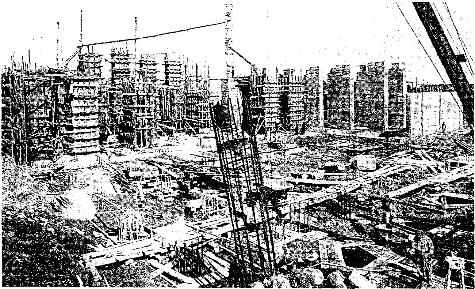
Constructing super structure foundation - October 1, 1914
