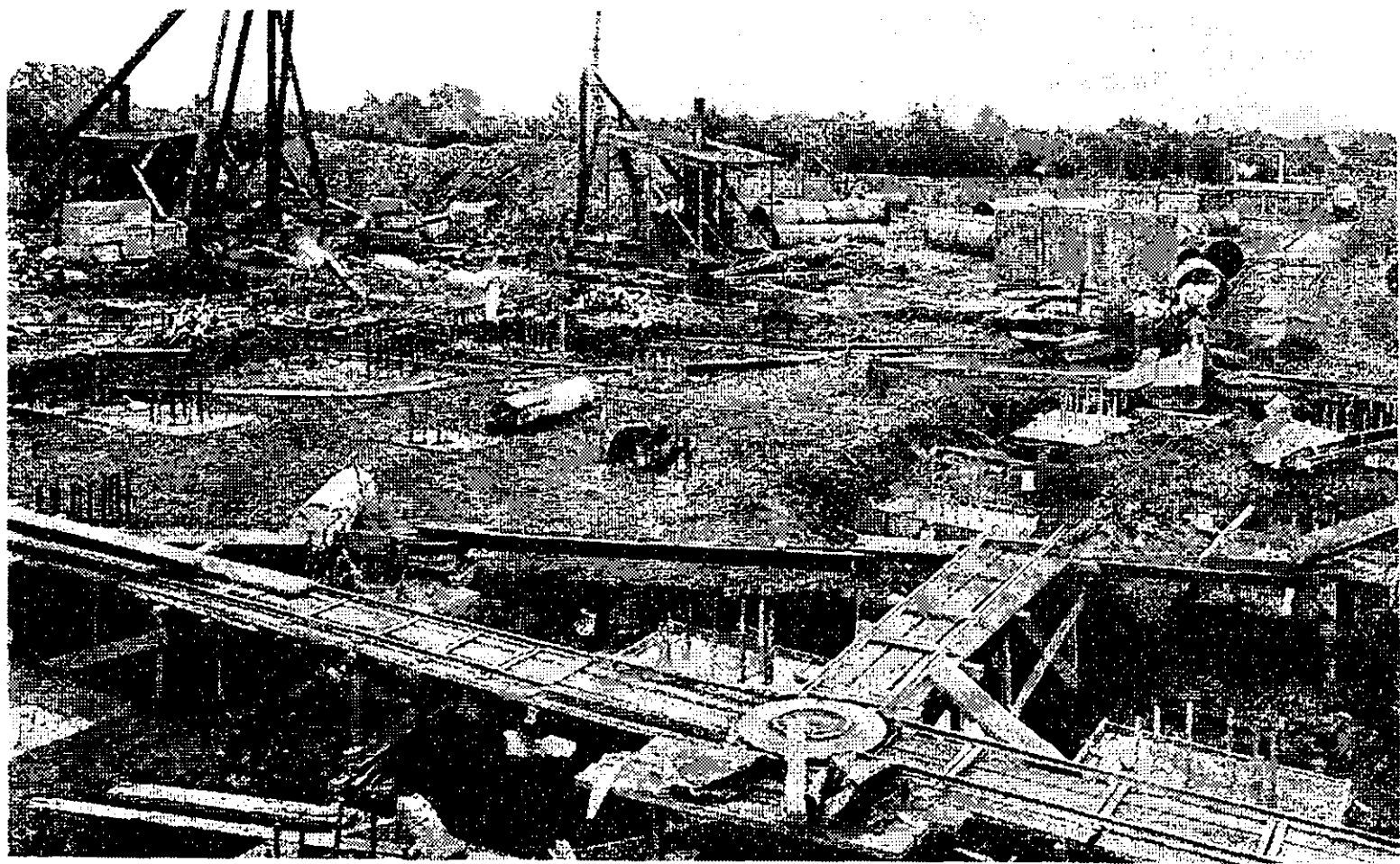
Sinking the caissons for concrete subfoundation to bedrock. (July 1, 1914)
