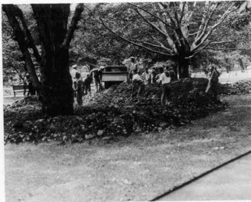
Fig. 35.--Workmen removing topsoil from around trees in Lafayette Park, July 1937.
