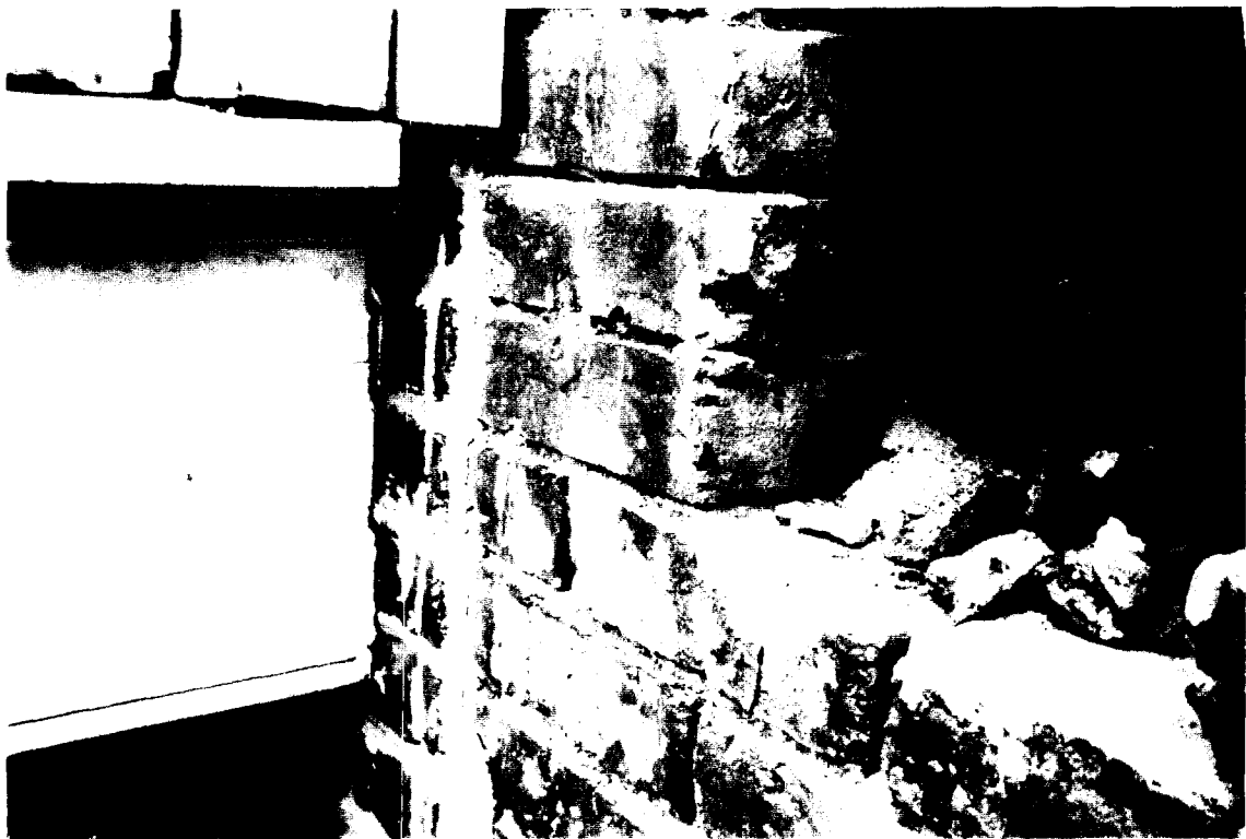
63-S Main House - View looking west into probe in the south elevation. South porch framing is at left.
