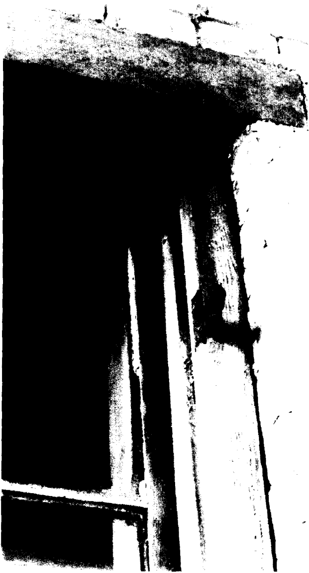
66-A Dependency - Caulk gaps at window frames on north facade.
