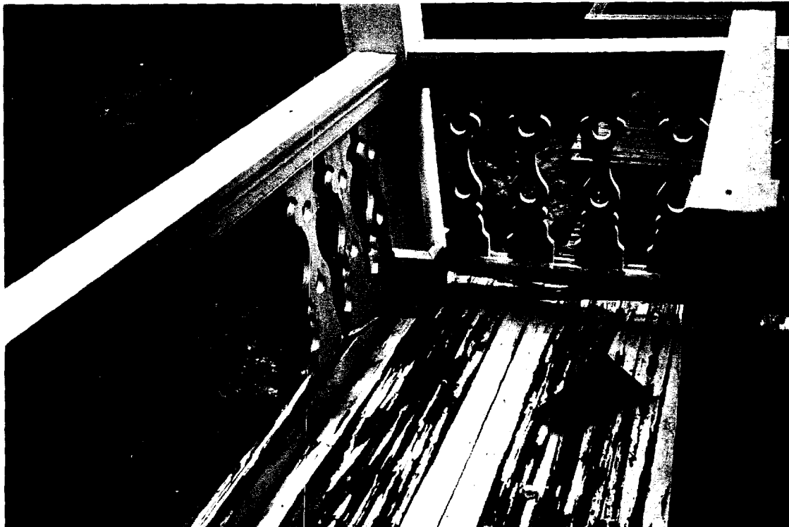
27-A Main House - Peeling paint on porch, and rotted balustrade.
