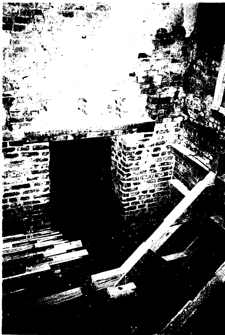
42-S Main House - View of rotted wood below south porch ground floor.
