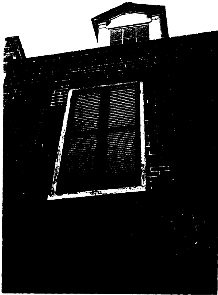
28-A Main House - Peeling paint on north facade window frames.
