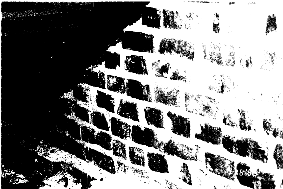
23-A Main House - Deteriorated mortar on east wall in attic.
