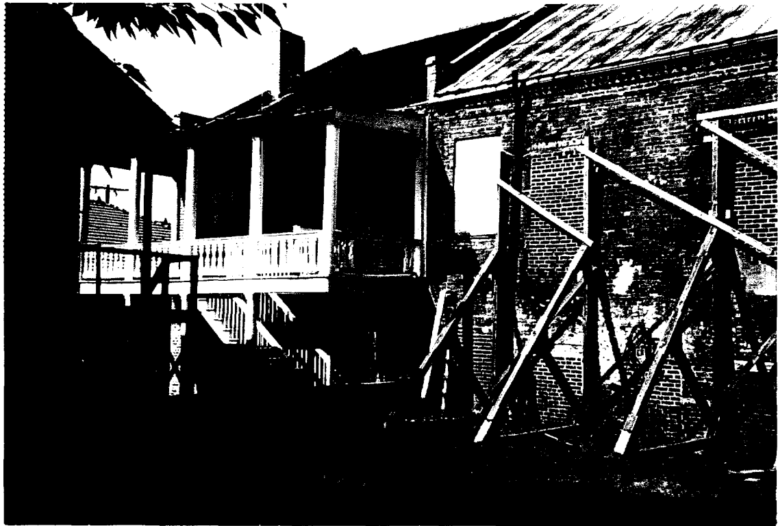
54-S Main House - South elevation of the William Johnson House and McCallum House. Note missing wood column on right side of porch.
