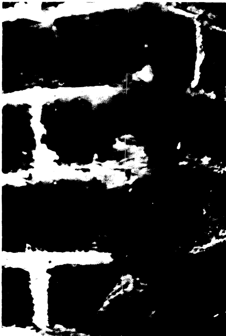
64-A Dependency - Poor match of mortar on north facade.
