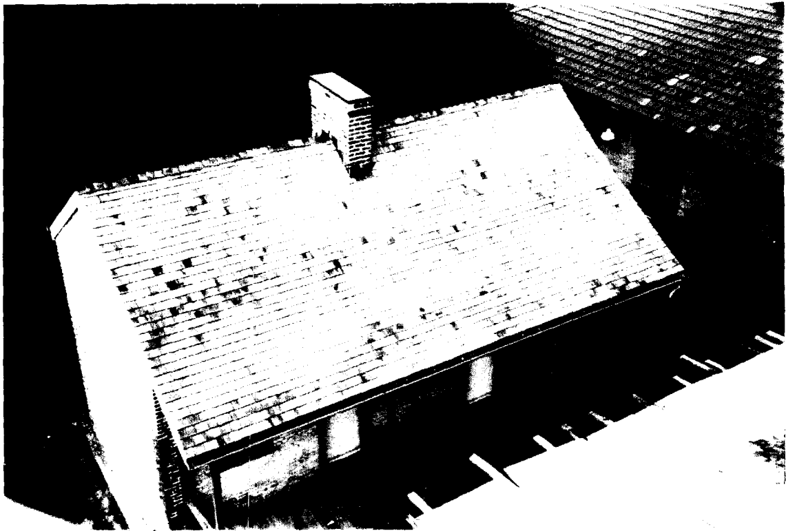
58-S Dependency - View of the northern half of the roof of the dependency.
