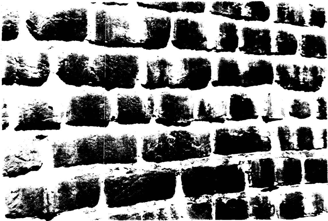
71-S Dependency - Close-up of deterioration of brick on the south elevation.
