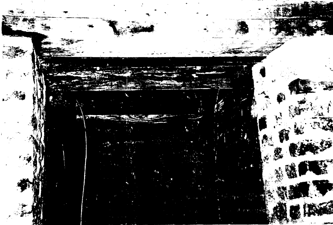
42-S Main House - View of rotted wood below south porch ground floor.
