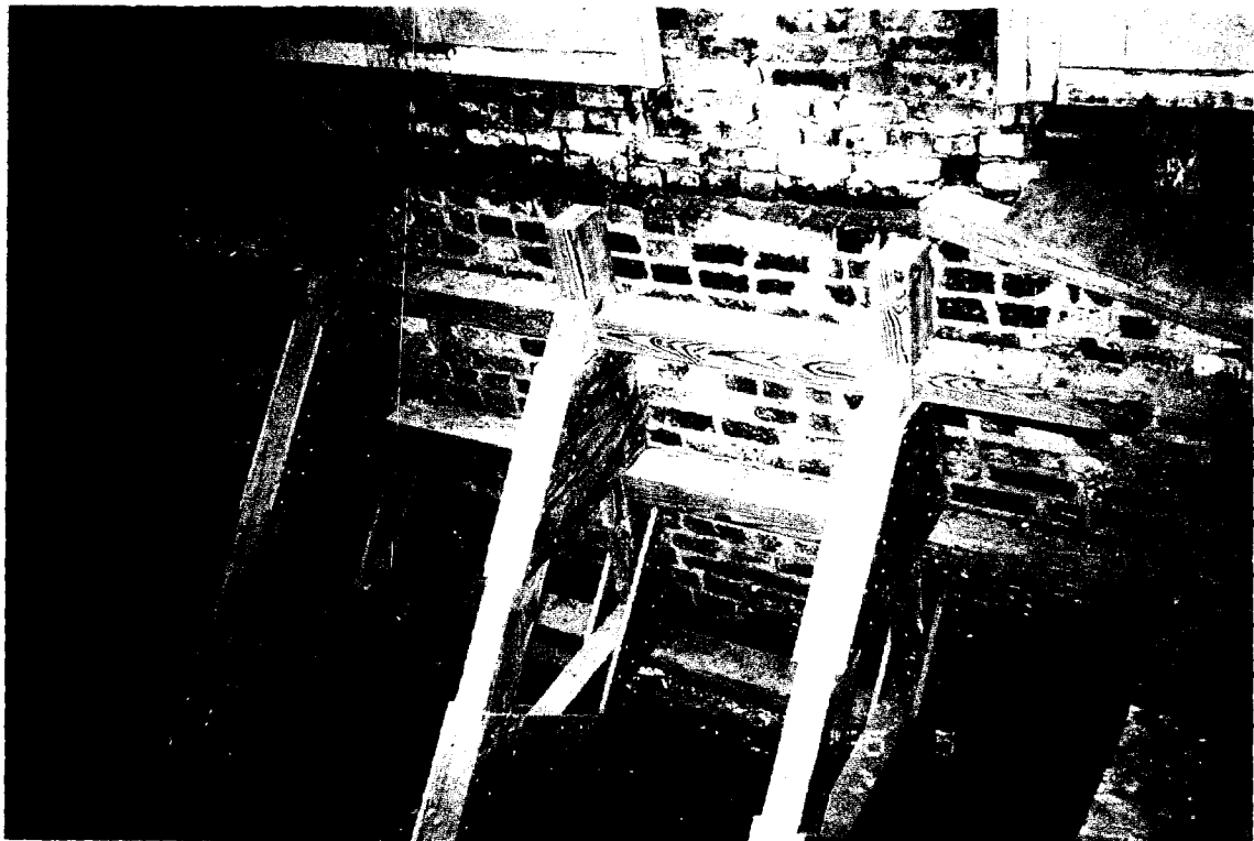
51-S Main House - View of north end of basement, showing diagonal bracing installed by National Park Service.
