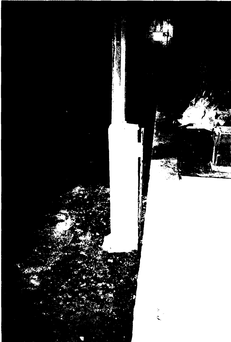
44-S Main House - View of bottom of weather column supporting second-floor partition wall above.
