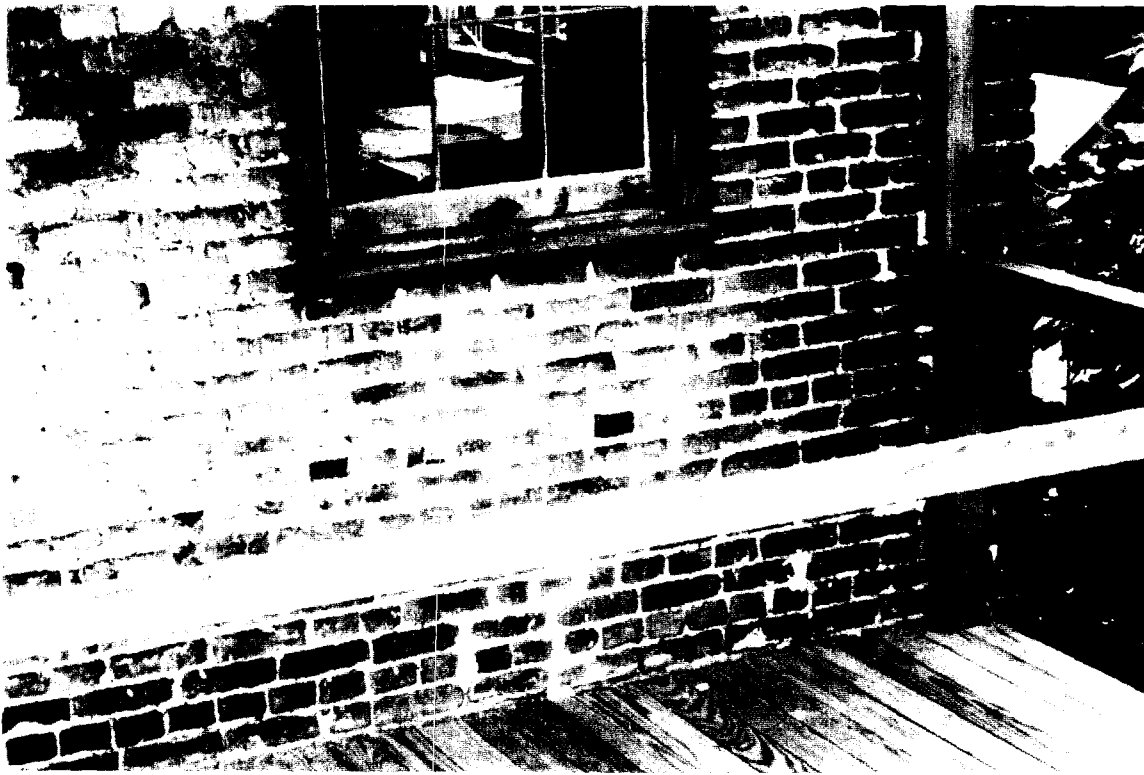
64-A Dependency - Poor match of mortar on north facade.
