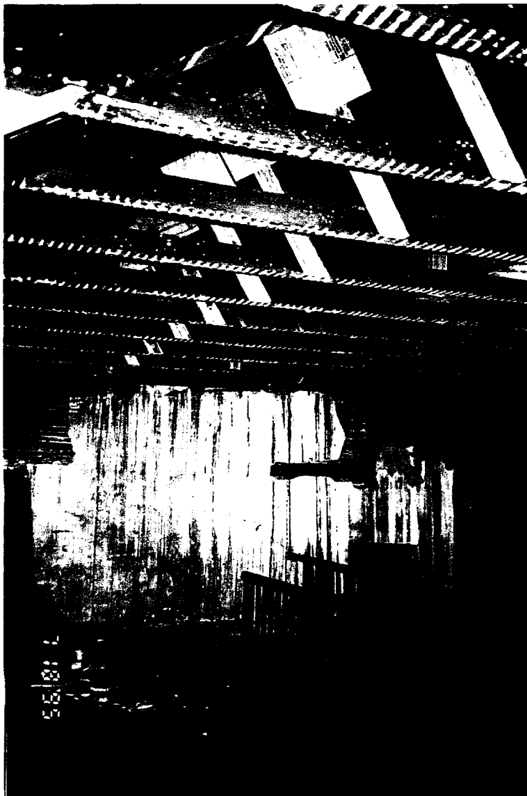
40-A Main House - Missing third-floor plaster.
