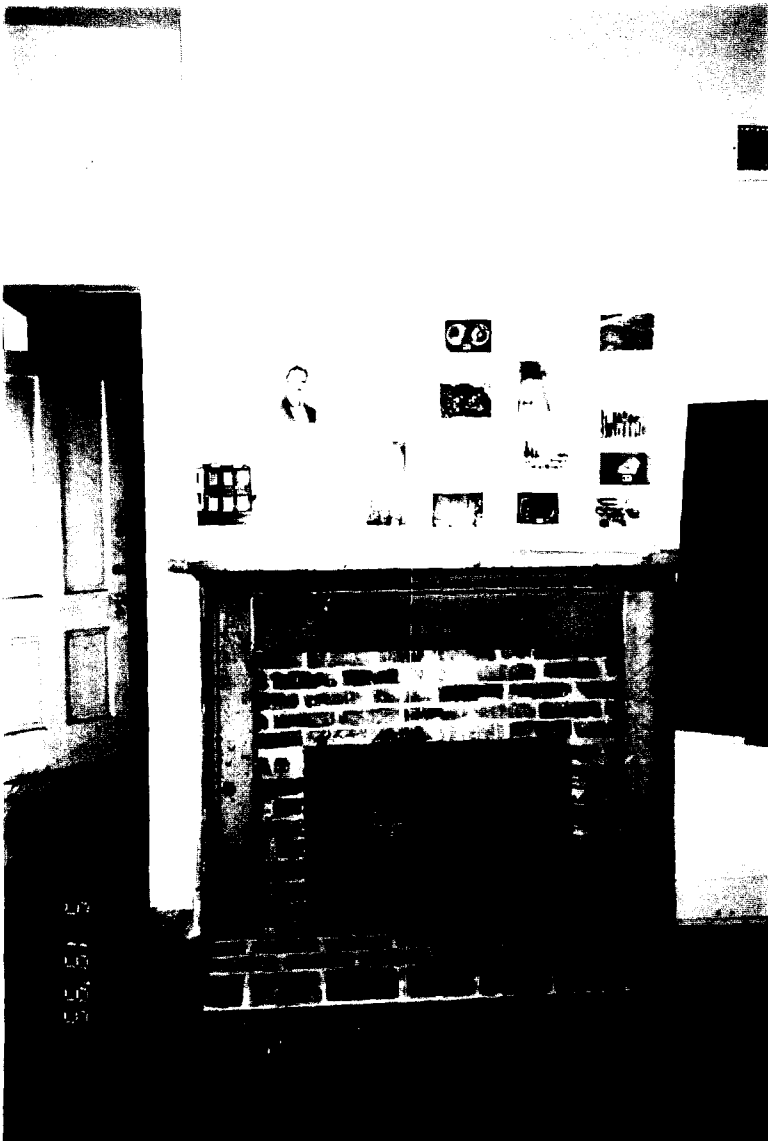
68-A Dependency - Second-floor walls replastered, unpainted.
