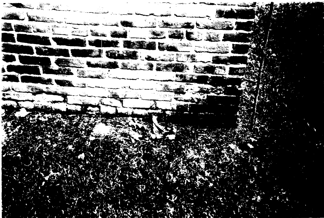
72-S Dependency - View of the rising damp damage to the brick and mortar at the southwest corner.
