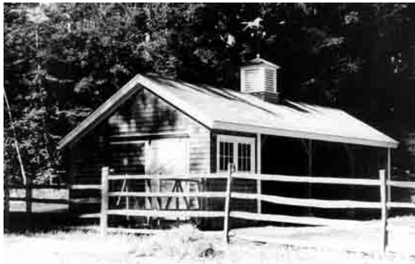
Figure 6.26: The Horse Shed, view west with its original three open stalls, c.1965. Billings Family Archives. The four-rail split-rail fence in the foreground enclosed a small corral; the entire Upper Meadow was also enclosed by the same type of fence. The dirt road visible through the center of the meadow is a remnant of the original Kitchen Garden designed by R. M. Copeland.
