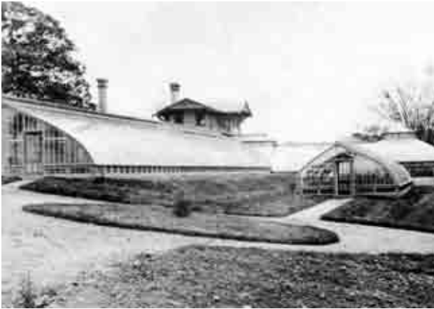
Figure 3.23: The west side of the Hothouses, with the Grapery and adjoining hotbed to the left, the Rosary to the right, and the Belvedere, Tropical House, and Octagon in the background, c.1875. Billings Family Archives. The circle at the end of the service drive to North Street is in the foreground.
