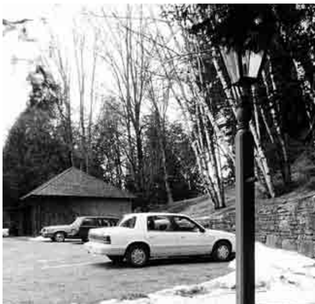
Figure 6.24: The parking area at the rear of the Mansion illustrating the new garage, built c.1977. National Park Service, 1997. The Colonial-style lantern and parking area were installed during the Rockefellers' initial improvements in the late 1950s.
