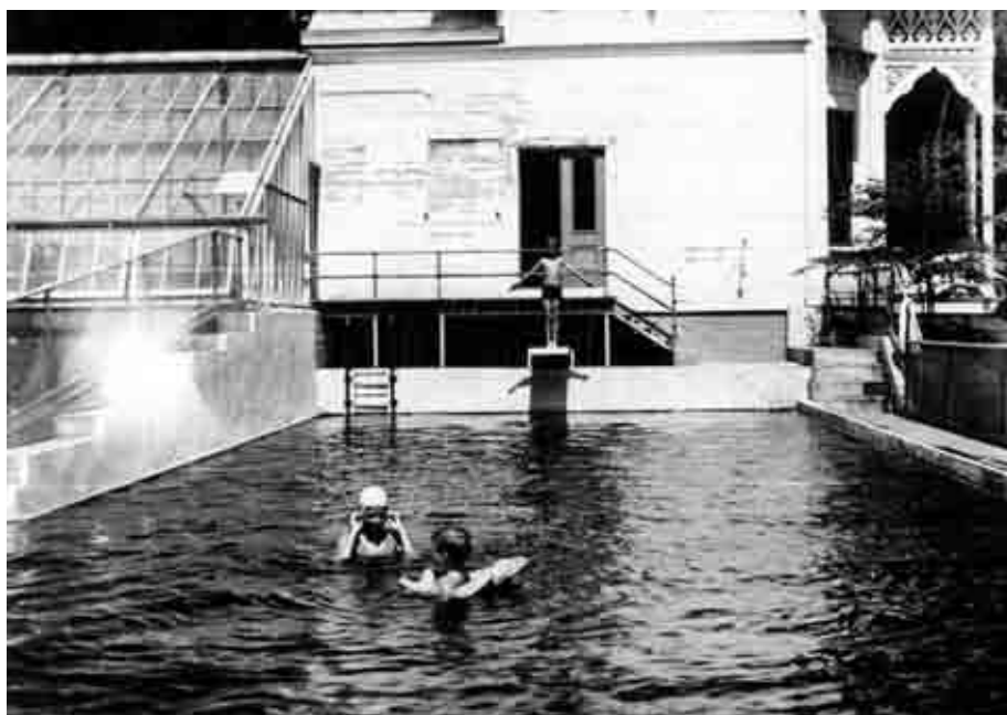
Figure 5.14: The new swimming pool built in the foundations of the Hothouses, showing the south wall of the Belvedere, formerly within the Tropical House, c.1937. Billings Family Archives. The remaining greenhouse, the former Grapery, is at the left.
