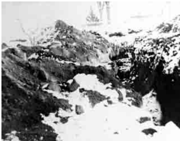
Figure 6.16: View east from the Mansion verandah in the winter of 1962, showing excavation undertaken for construction of the Mansion fallout shelter. Courtesy Mimi Bergstrom, Woodstock, Vermont.
