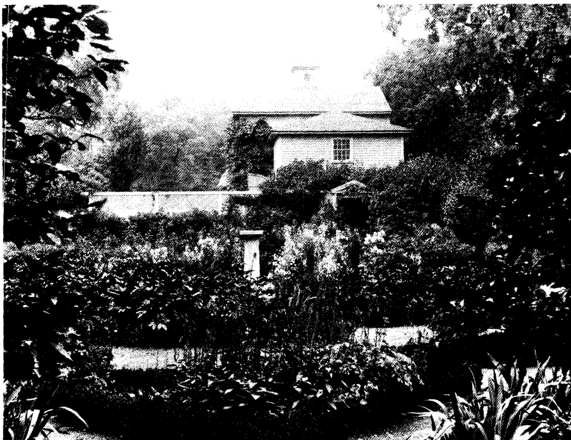
Figure 40. The completed trellis after 1905. Photograph by Martha Hutcheson. Courtesy of the Morris County Park Commission.
