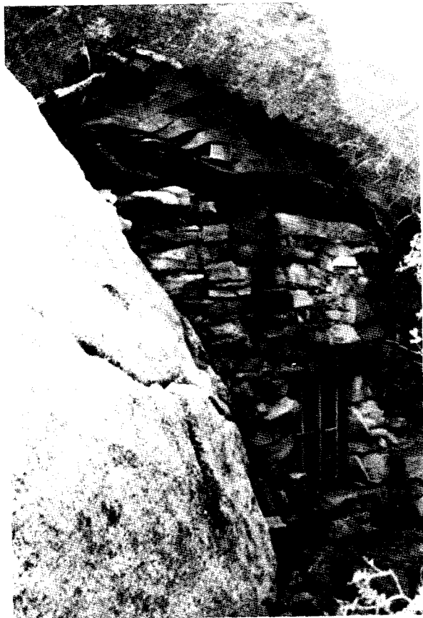
Illustration 74 (left). Outside wall of rock house, Eagle Cliff Mine. Note tin can roof and six-light window. NPS photo by Gordon S. Chappell, 1976.
