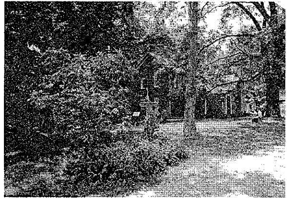
Figure III-8: Farmhouse and front yard, 8/11/98.
