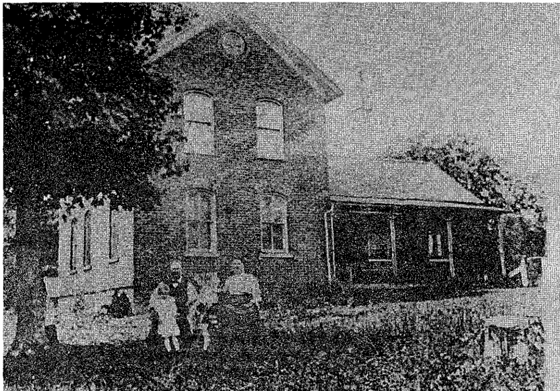
Figure II-15: The south and east sides of the house, with the windmill visible in back, circa 1908. (H2-0002)
