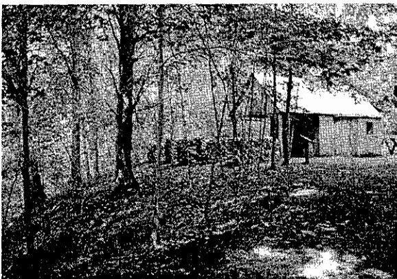
Figure III-29: Sugar camp, southeast elevation and slope, 8/11/98.
