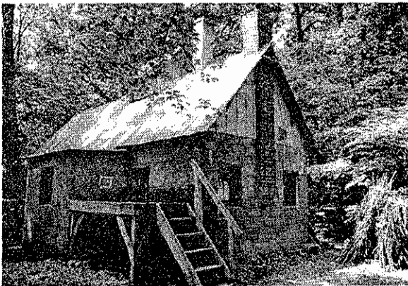
Figure III-28: Sugar camp, northeast elevation, 8/11/98.
