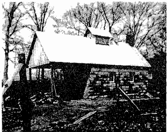
Figure II-32: The sugar camp with a fence running along the ravine. Early 1935 or 1936--the pump house addition has not yet been built. (INDU8138)
