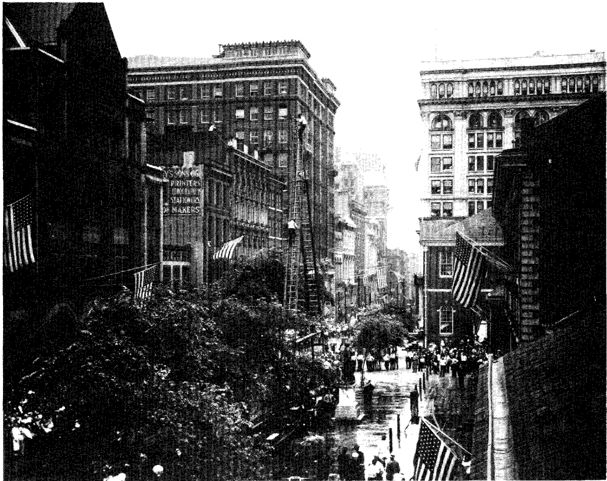
FIGURE 19. CHESTNUT STREET OPPOSITE INDEPENDENCE HALL, 1937. As if to emphasize the civic concern over the fire danger to Independence Hall, ceremonial fire drills were often held here. This 1937 photograph records a drill staged for the National Association of Fire Commissioners. Of the neighboring Chestnut Street buildings seen here, only the Lafayette Building (the tallest building) and a few of the small, ornate bank buildings to the right of it survive. None succumbed to fire. ( Independence National Historical Park photo. )
