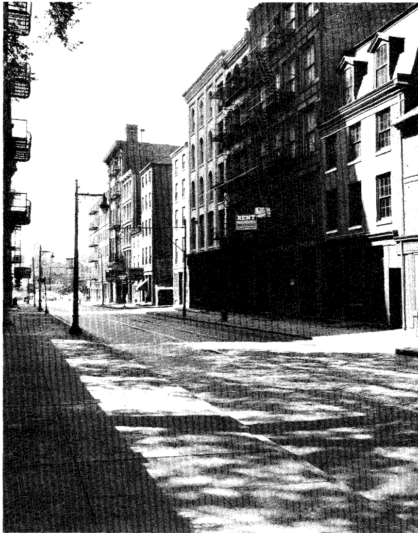
FIGURE 26. FIFTH STREET BEFORE DEMOLITION FOR THE SECOND BLOCK OF THE MALL, 1953. Part of the second block, between Commerce and Cuthbert streets, is seen from Fifth Street in 1953. Demolition for the first block had opened a view to the south to Old City Hall. Trees on the first block subsequently obscured this view. ( Independence National Historical Park photo. )
