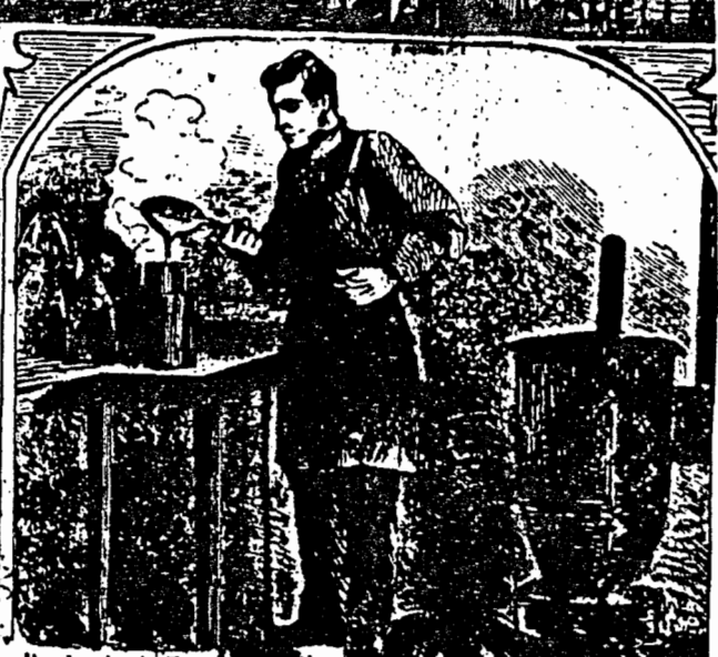
Pouring in the Lead.
