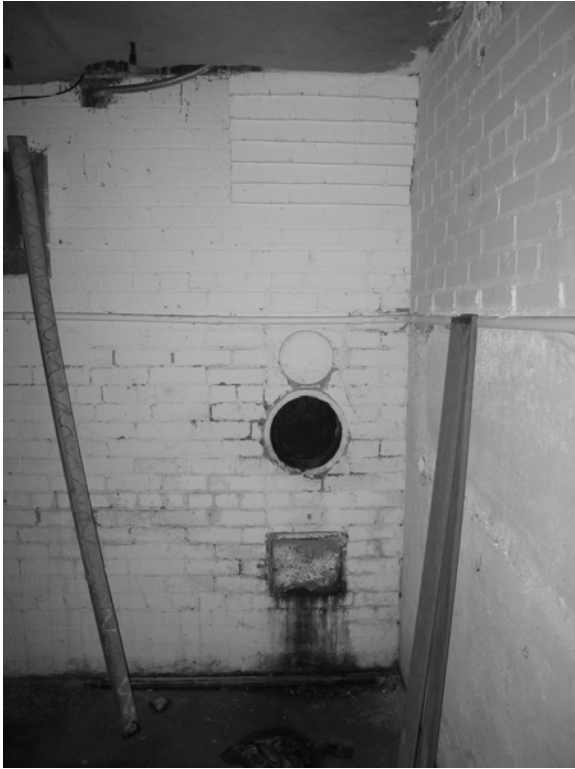
Figure C-3 Concrete and brick foundation wall
