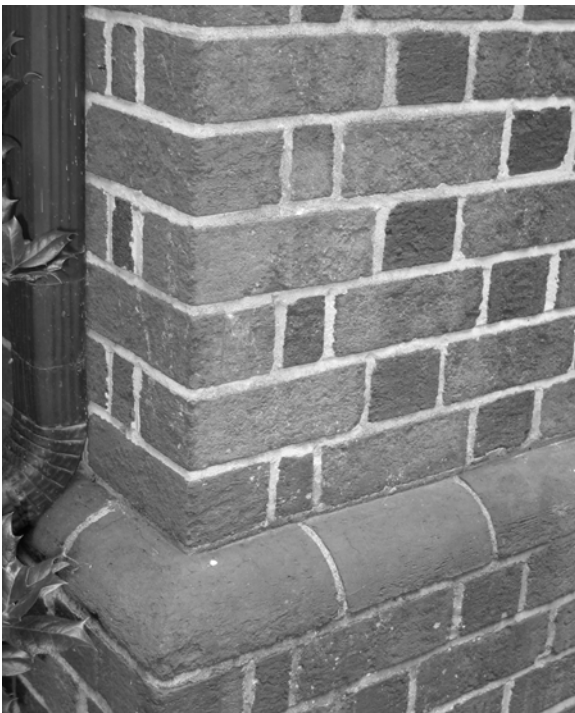
Figure C-4 Flemish bond brick wall and watertable
