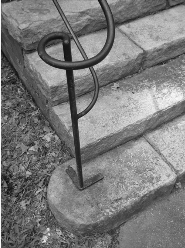
Figure C-15 Front entrance stairs and railing
