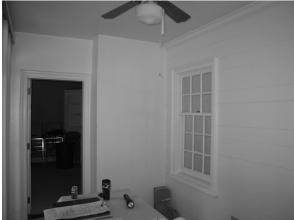
Figure C-31 Room 104 facing northwest
