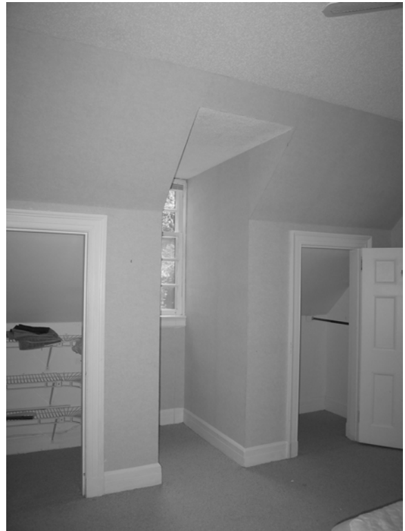
Figure C-40 Room 201 facing southwest
