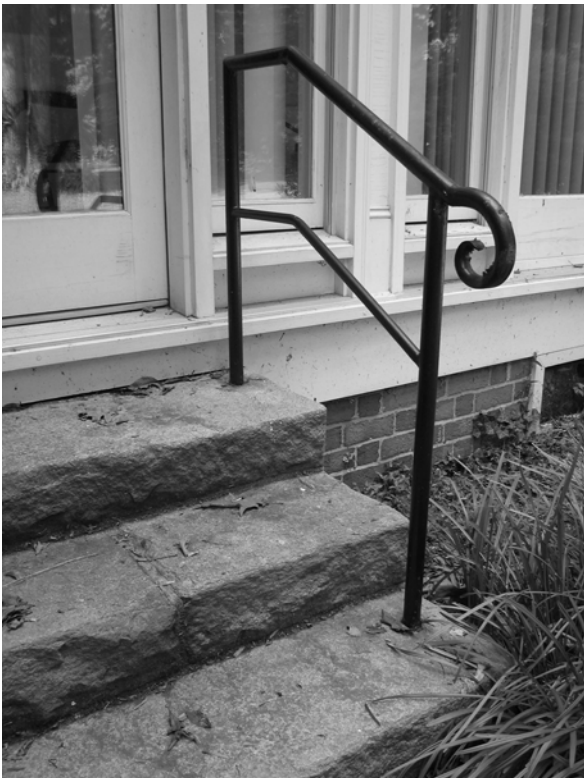
Figure C-16 South porch stairs and railing
