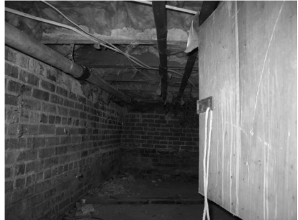
Figure C-18 View into basement crawl space
