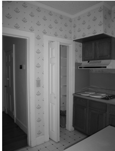
Figure C-36 Room 107 facing northwest
