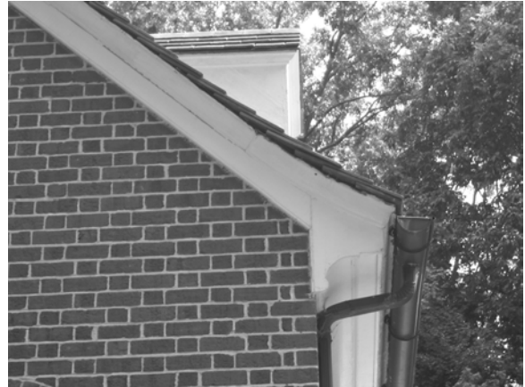
Figure C-9 Rake board and cornice at main block
