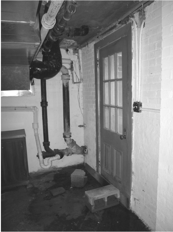
Figure C-20 Exterior sash door at north wall of Room 001
