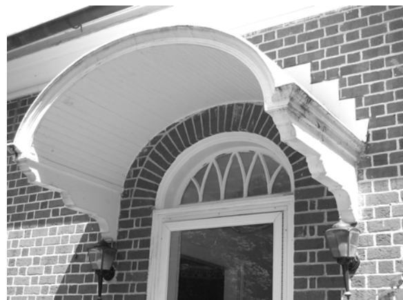
Figure C-17 Hood at front entrance
