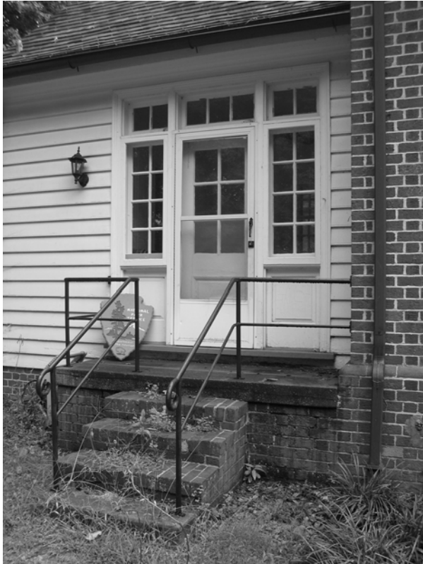
Figure C-11 North doorway to east wing
