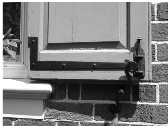
Figure C-14 Shutter hardware
