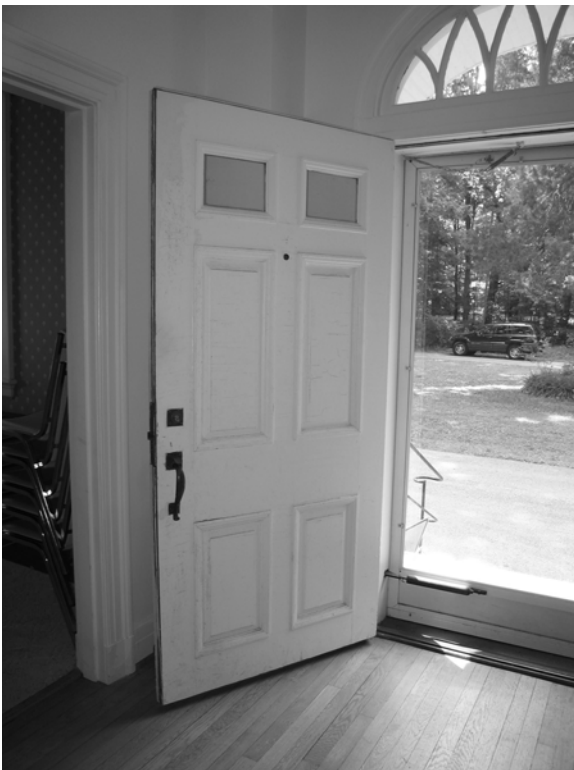
Figure C-26 Exterior door on south wall of Room 102
