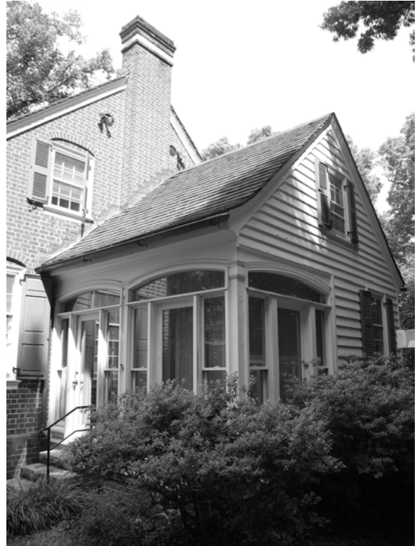
Figure C-5 Southeast oblique of frame wing
