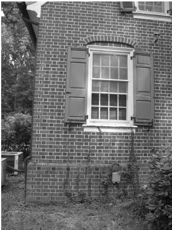
Figure C-12 Eight-over-twelve window on west elevation
