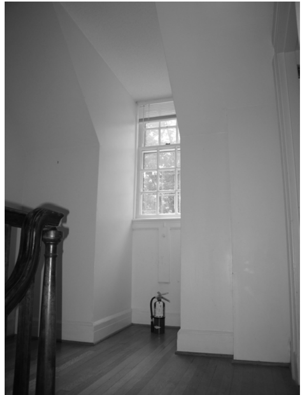
Figure C-42 Dormer window on north wall of Room 202
