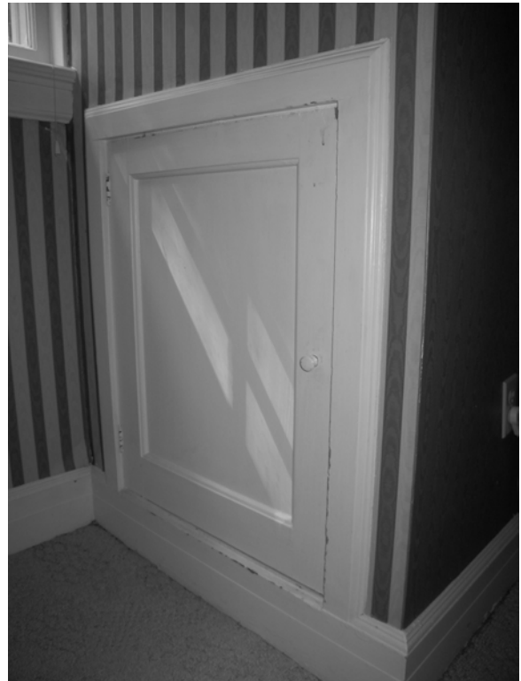
Figure C-46 Attic access door in south dormer
