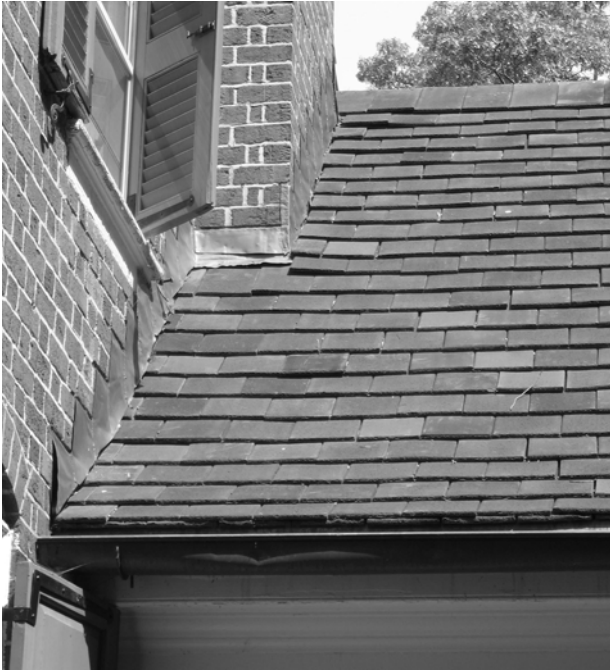
Figure C-7 Roof shingles, stepped flashing, and gutter
