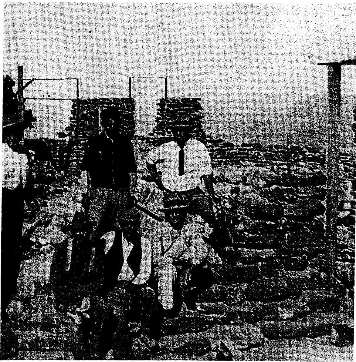
Figure 1. This photo depicts the construction crew in front of the Yavapai Observation Station during construction in 1928. The curve of the open terrace is discernible in the background and the local stones that form the walls are seen rising around the window openings. GCNPA Photo Number 16796.
