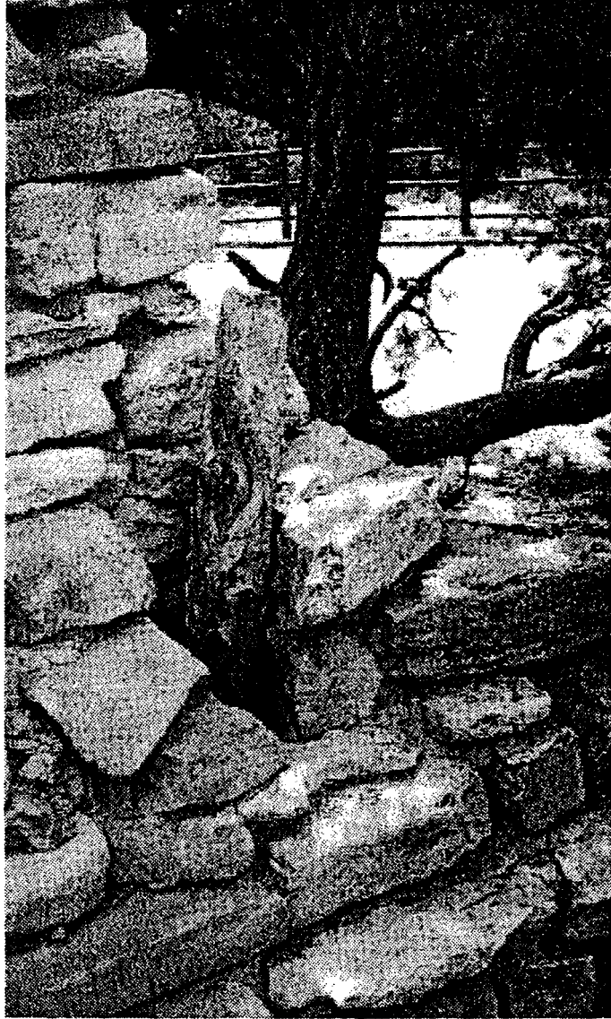
Figure 14. This image illustrates the tree well on the west side of the building, though the tree is no longer extant. Maier, ever sensitive to the surrounding landscape, incorporated this unplanned feature into the building during construction to accommodate an existing tree rather than cut it down. Photo dated May, 2000.
