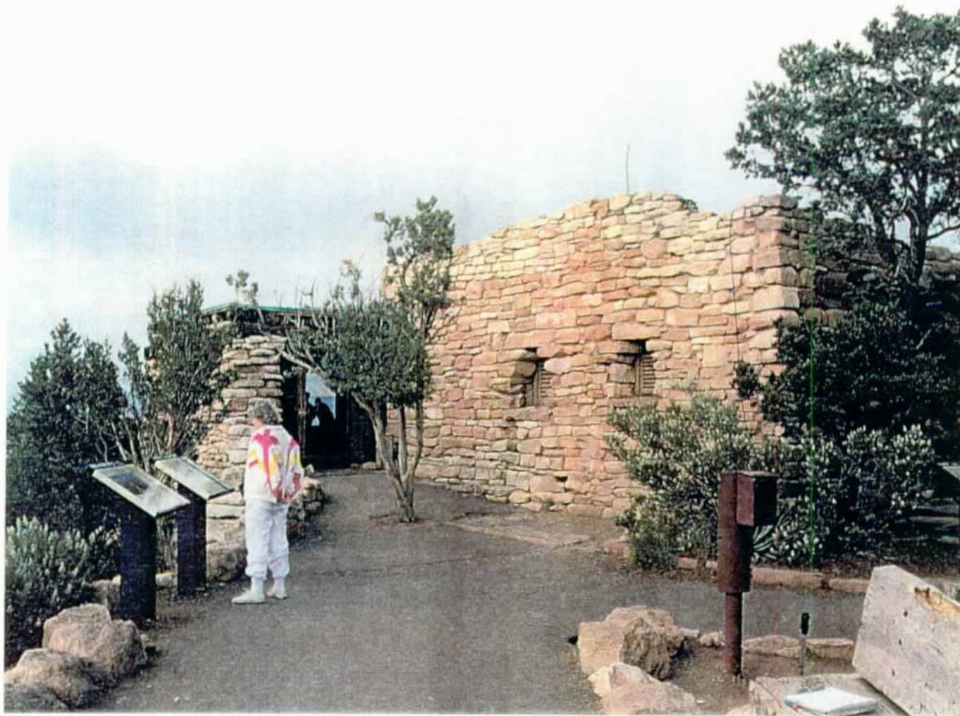
ELEVATION LOOKING NORTHEAST
