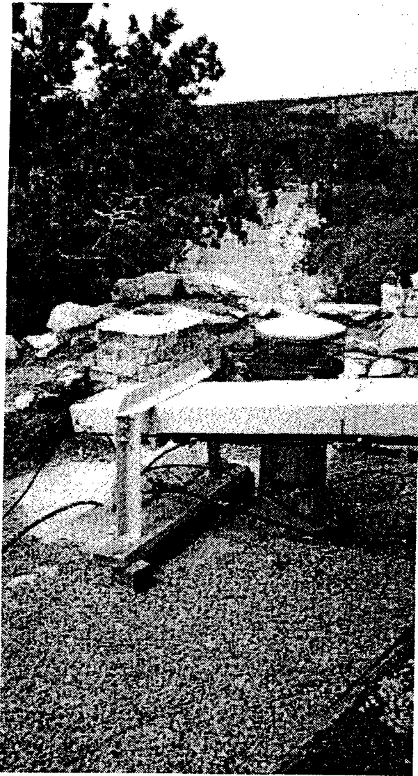
Figure 9. This image illustrates typical conditions on the flat tar and gravel roof. In the foreground is the brick chimney below the parapet. View is looking to the southwest corner. Long view is looking southwest. Note paved rim trail and boulders along the walk. Photo dated May, 2000.
