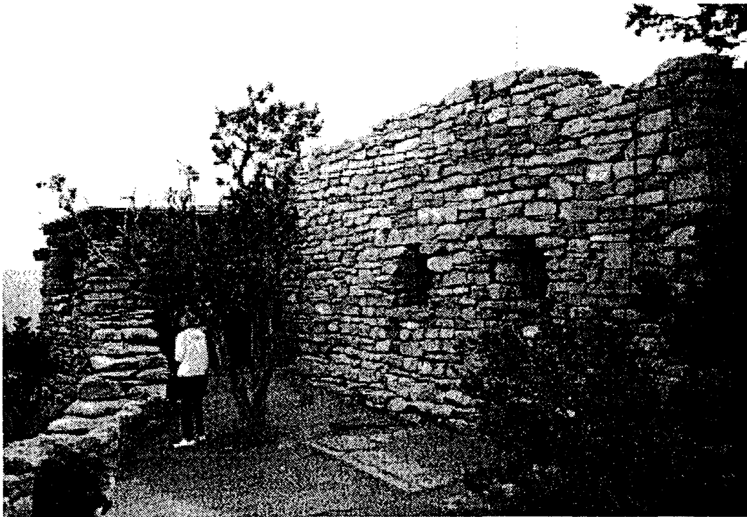
Figure 4. This image illustrates the west side of the Yavapai building. Photo dated May, 2000.
