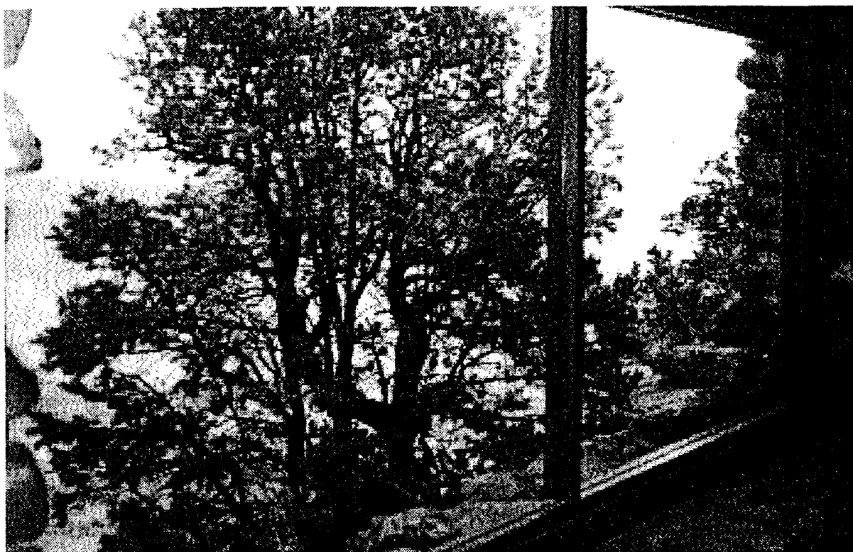
Figure 18. This image illustrates the windows on the east side of the Yavapai interior, inside the foyer entrance. The windows were installed in 1979, replacing the 1953 glazing. The windows look to the north. Photo dated May, 2000.
