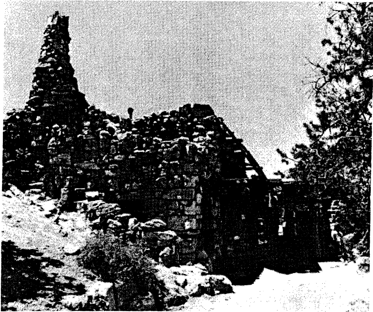
Figure 39. This image illustrates the exterior of Mary Colter's Hermit's Rest, 1914. Hermit's Rest was designed to look like a dwelling constructed with local materials by an untrained frontiersman. The exterior was meant to resemble a haphazard jumble and its roofline inspired the jagged profile at Yavapai. Image from Grattan, Virginia. Mary Colter, Builder Upon the Red Earth . p. 28
