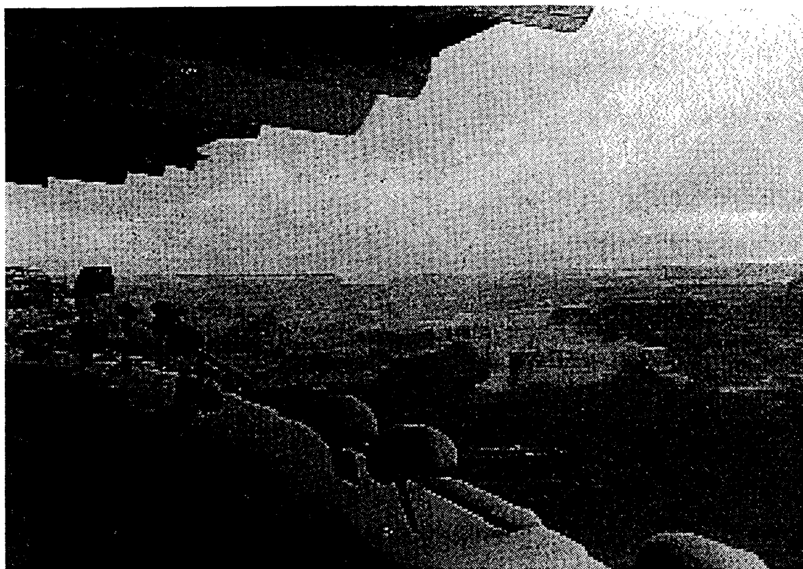
Figure 28. This photo of the open terrace at the Yavapai Observation Station during a snowstorm shows snow piled on top of the parapet and telescopes. The ingress of snow was described as a recurring problem that prevented the building from staying open year-round. Photo dated is 1944. GCNPA Photo Number 7022.
