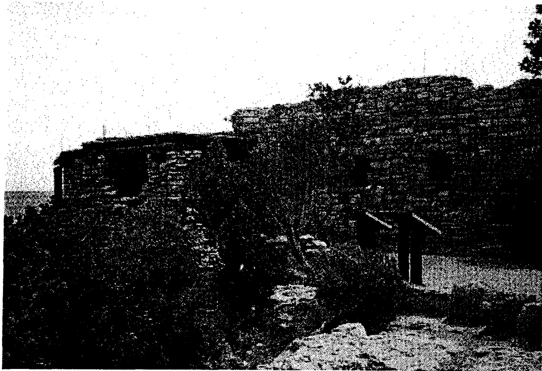
Figure 5. This image illustrates the western elevation of the Yavapai building. Photo dated May, 2000.
