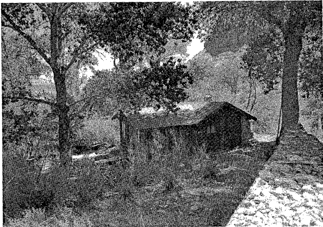
Figure 11. The image illustrates the roof configuration of the Trail Caretaker's Residence. From this angle, the image also illustrates the orientation of the cabin toward the inner canyon. ARG Photo dated May, 2000.
