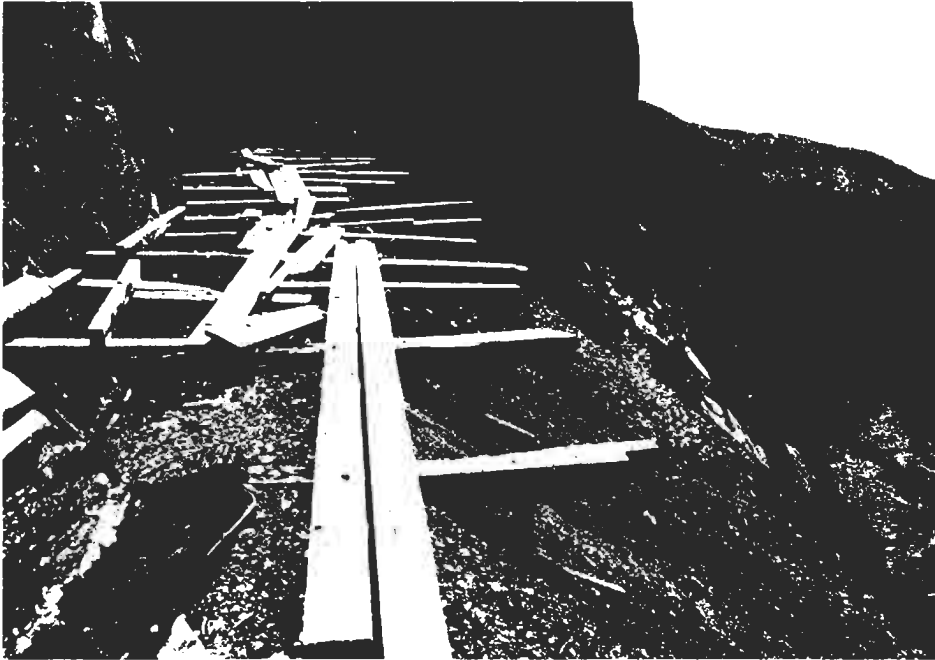
Lincoln Canyon Mine Tramway Supports
