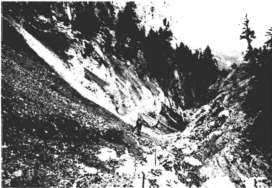
Lincoln Canyon Mine Waste Pile
