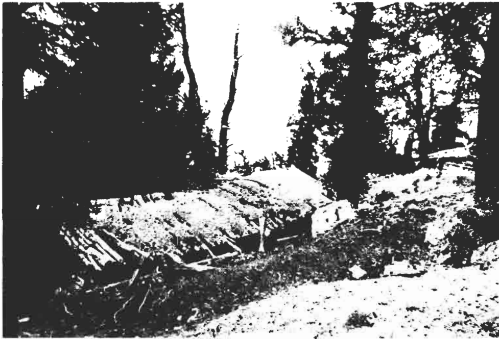
Views of Cabins at St. Lawrence Mine
