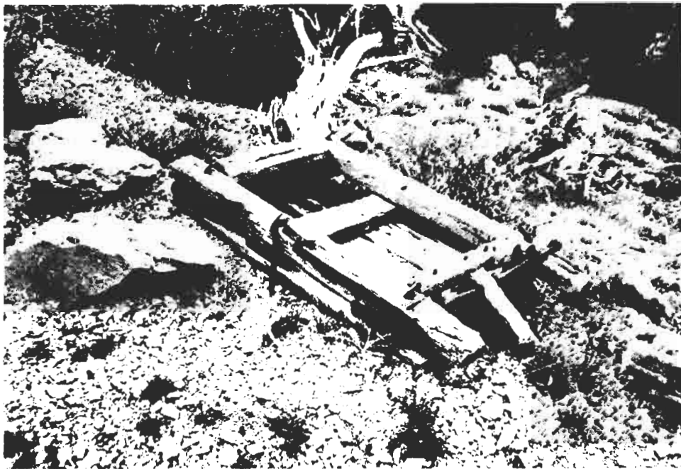
Sled at St. Lawrence Mine
