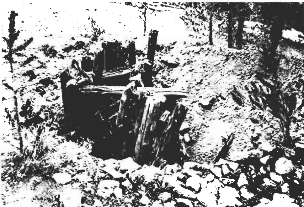
Views of Collapsed Adits and Shafts at St. Lawrence Mine
