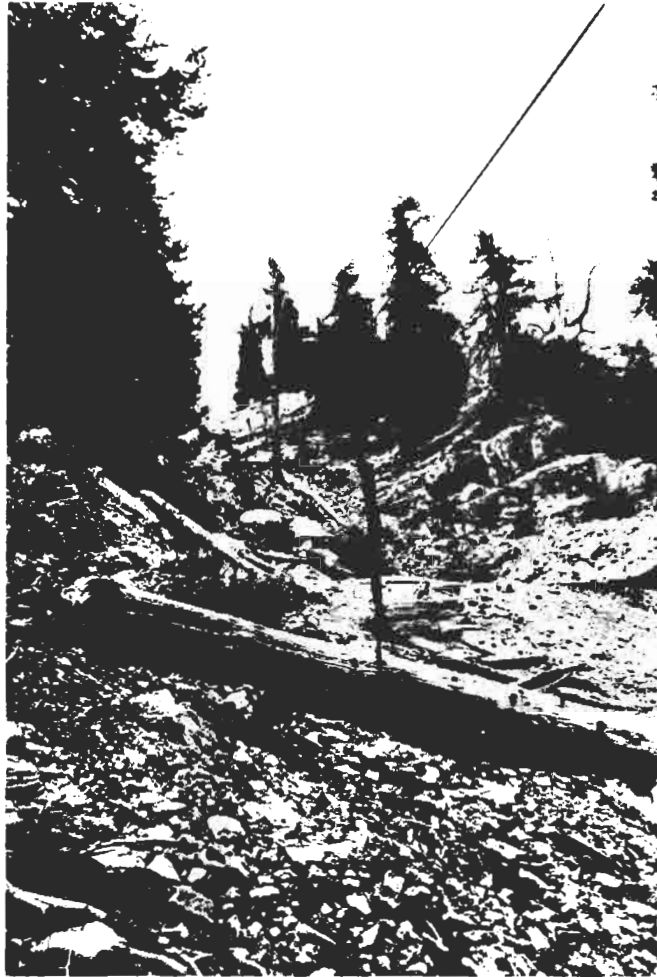
View of Cableway Remnants at St. Lawrence Mine
