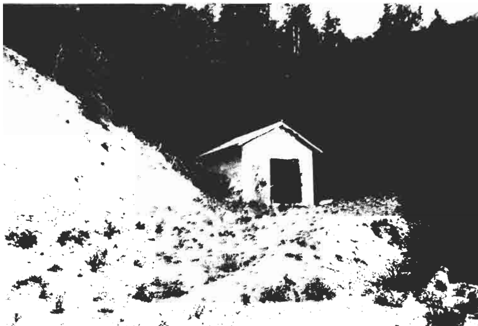
Cinder Block Dynamite Structure
