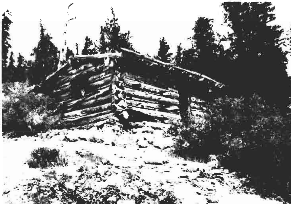
Views of Cabins at St. Lawrence Mine
