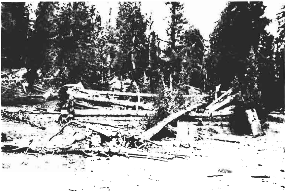
Partially Collapsed Cabin at St. Lawrence "South"
