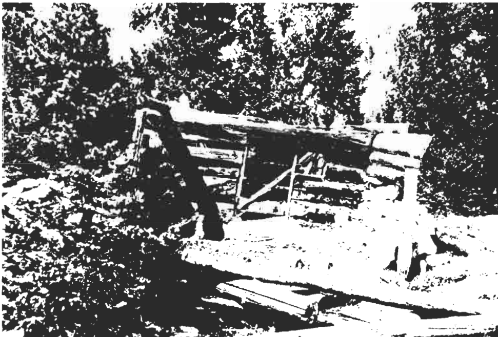
Partially Collapsed Log Cabin at Johnson Mine Just Below Johnson Lake
