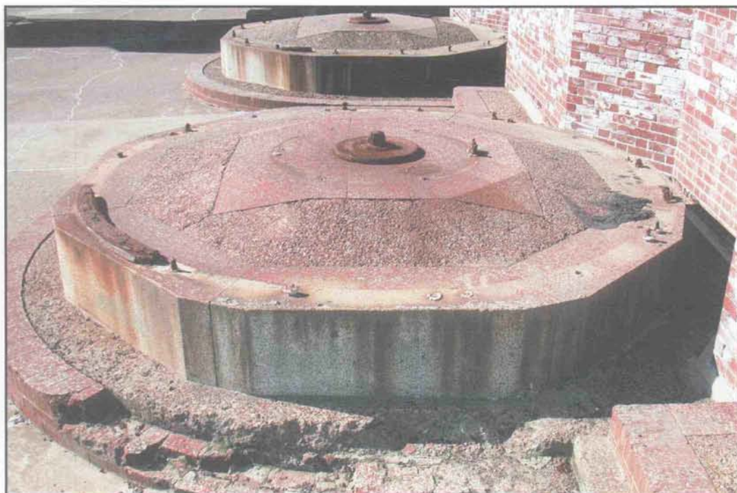
Condition Photo 8: Gun Emplacement No. 104; Open joints, spalled and missing bricks at the gun emplacements. Metal attachments are improperly sealed and are corroding and staining the concrete and granite materials. (Courtesy of ARG, 2003)
