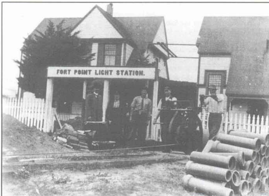
Below: Two of the assistant keepers' houses at the Fort Point Light Station were built atop the hill south of the fort. A windlass helped haul supplies up the steep slope to the "wickies" homes. Terra cotta pipes in the foreground were for plumbing. Photo circa 1910. Credit: Fort Point NHS Collection, Golden Gate National Recreation Area.
