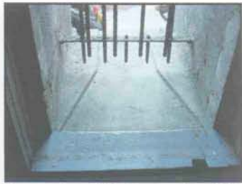
The outline of the former rifle slit is visible in all the window sills along the southwest gorge elevation. (Jane Lehman, 2005)
