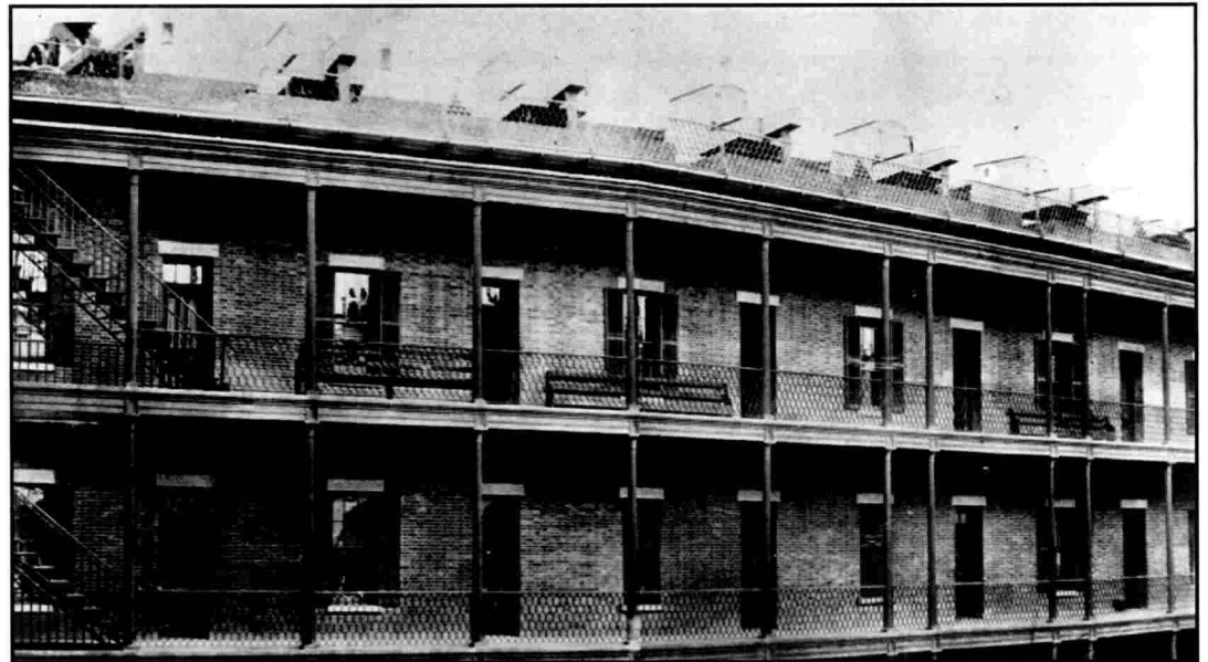
Figure 4. Photograph: Gorge side of Fort Point, viewed from the parade, 1865. Credit: Fort Point NHS Collection, Golden Gate National Recreation Area.
