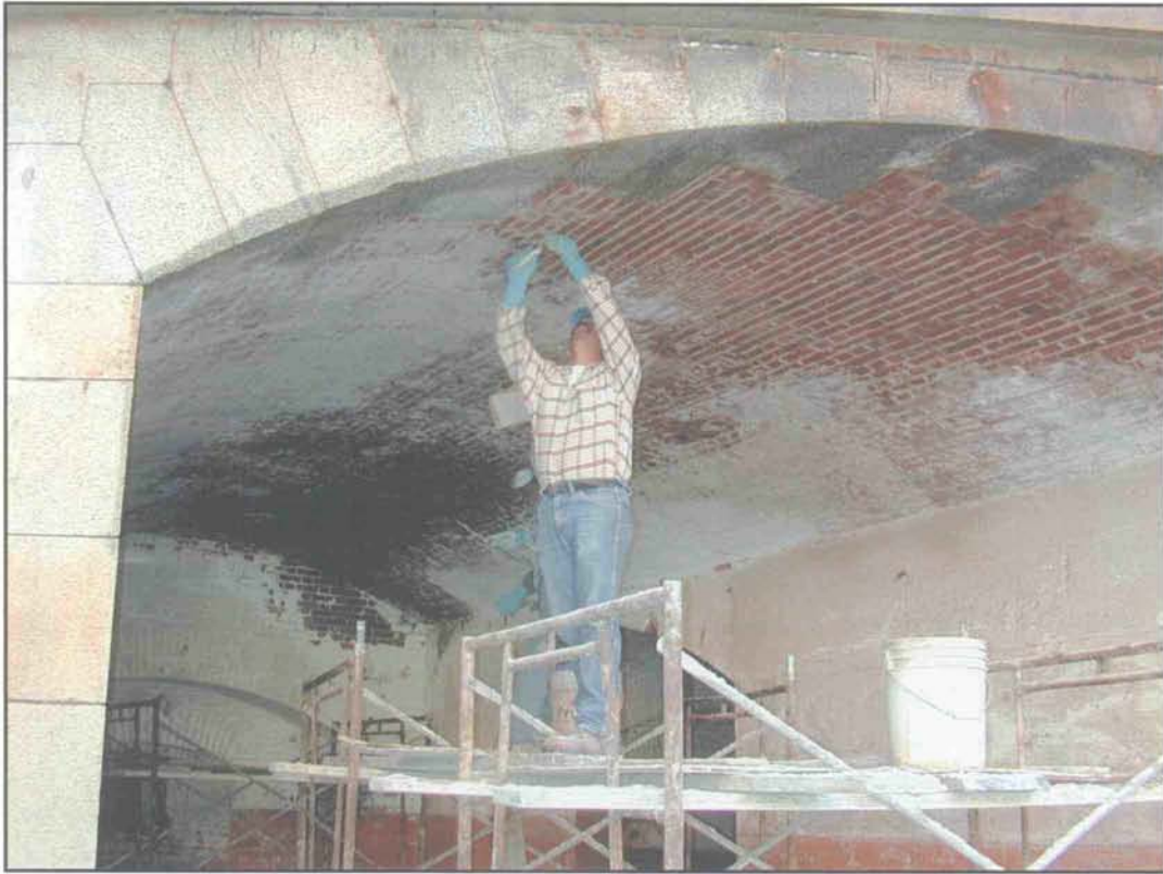
Condition Photo 22: Masonry repointing project at 1 st tier. (Courtesy of ARG, 2003)
