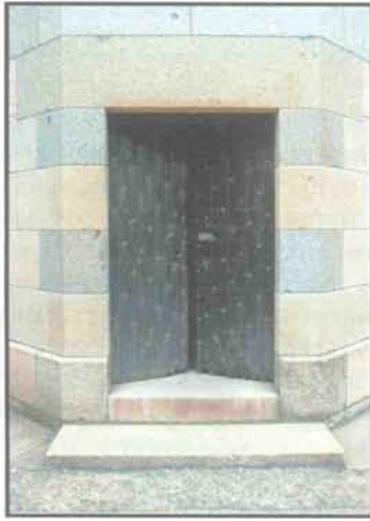
Courtyard level doors into stair #2. This is one of the few pairs of heavy wood doors original to the fort's construction. (John Martini, 2005)
