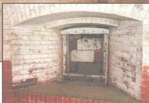
Most of the iron embrasures have deteriorated over the years and the openings have been infilled with brick and block for security purposes. (John Martini, 2005)
