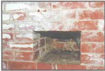
This small kitchen vent has a keystone brick on the top part of the opening. (John Martini, 2005)
