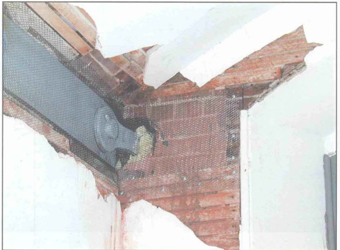
Condition Photo 21: Detail of brick lath, wire mesh, and plaster layers. (Courtesy of ARG, 2003)
