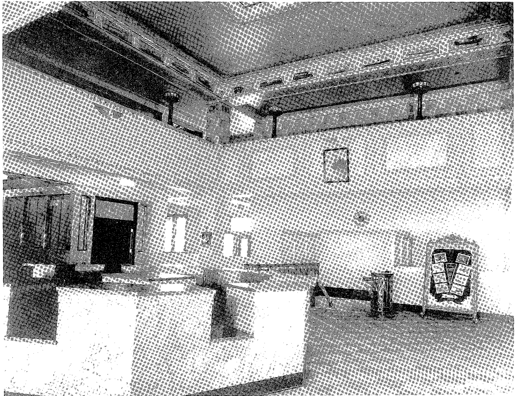
Figure 155. View of lobby, looking northeast, showing interior finishes, stairway down to passenger-loading tunnel, and baggage-check counter, 1937.
