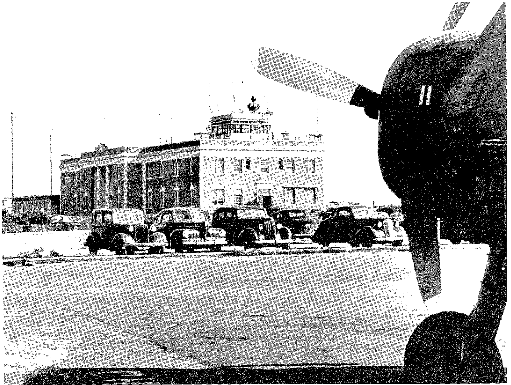
Figure 149. West and south sides of the Administration Building, showing glass blocks installed in windows W 1-24 and W 1-25, ca. 1945.
