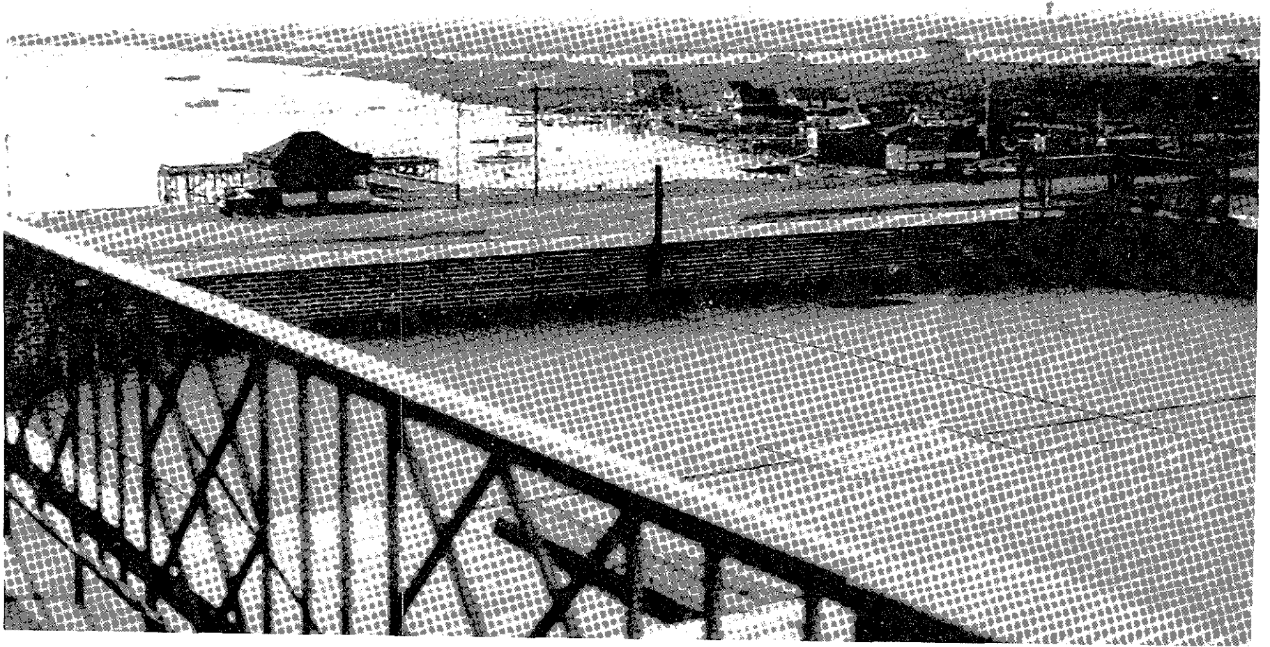
Figure 134. Northwest corner of Administration Building roof, looking west, ca. 1935. (Photograph does not show spotlights installed on the west parapet in 1936.)
