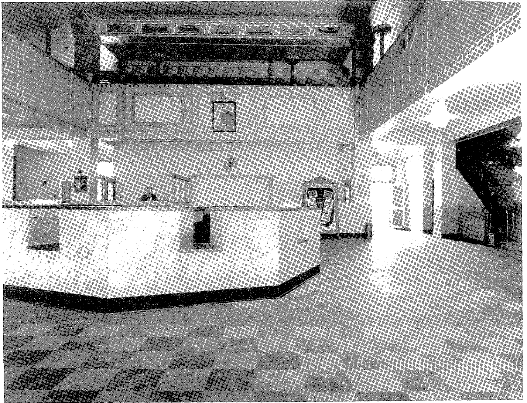
Figure 157. View of lobby, looking east, showing interior finishes and baggage-check counter, 1937.
