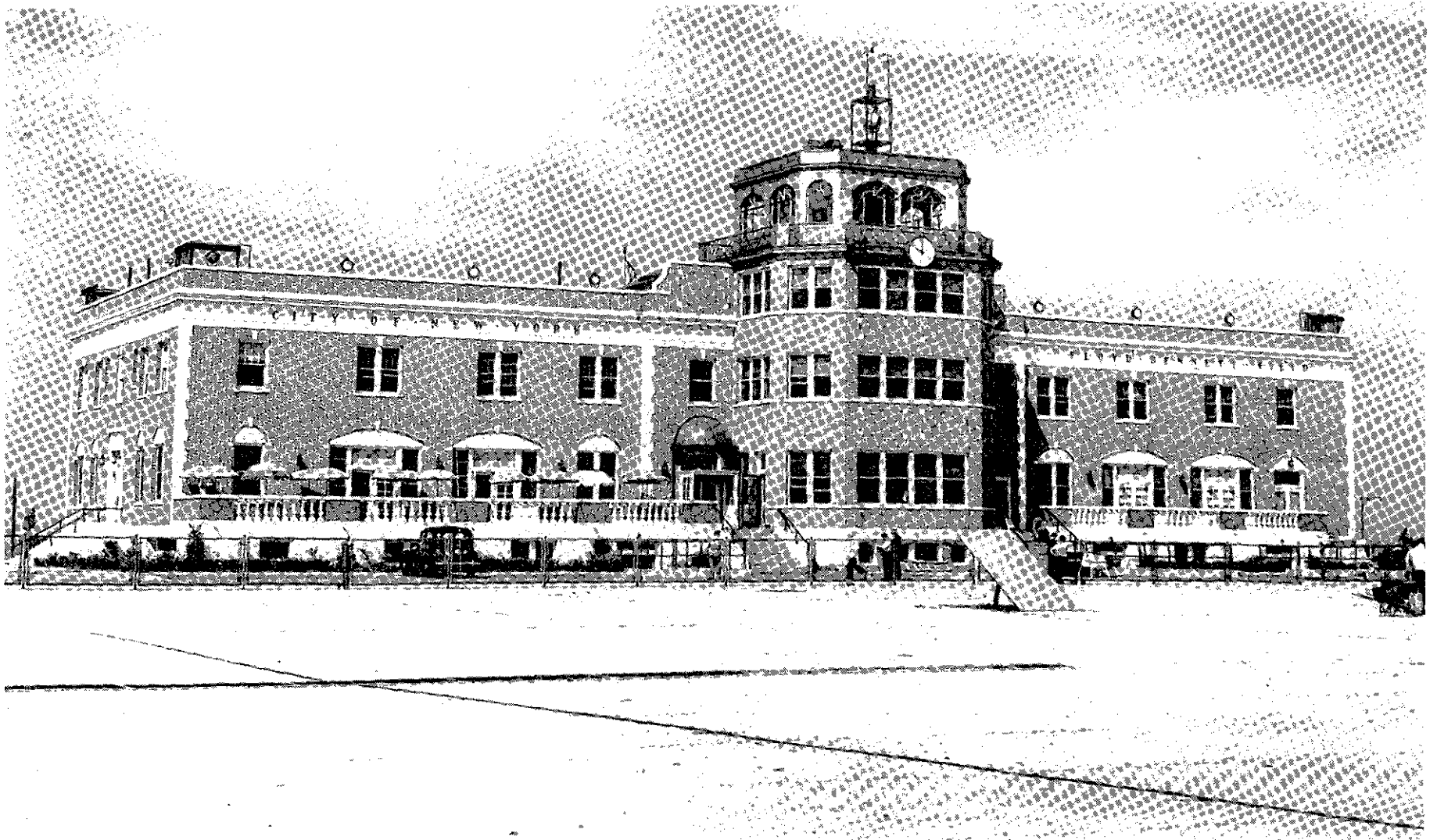
Figure 128. The Administration Building newly constructed, south and east sides of building, ca. 1932.
