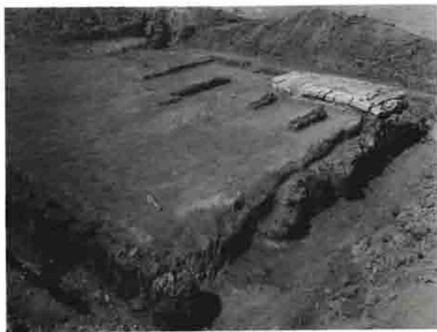
Figure 39. Photo. Building 6-510 Vestibule. [Cattanach 6/29/57 Neg FOUN-156(s)]
