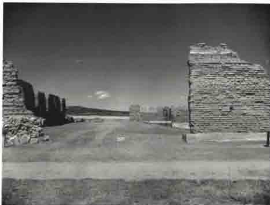
Figure 4. Same view after removal of dirt and debris. [Wilson 4/29/59 Neg FOUN-356(s)]
