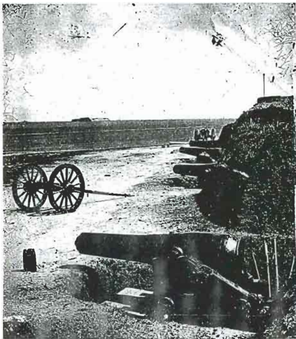
Fort Johnson's four-gun water battery, 1865. Top to bottom: 8-inch howitzer, siege and garrison, Model 1841; 10-inch columbiad, Model 1844, rifled & banded; 7-inch double-banded Brooke rifle; 10-inch Confederate columbiad; 10-inch Confederate columbiad. The carriage to the left is a wagon used for transporting mortars (National Archives).
