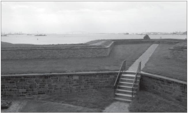
Figure 8.17 Star Fort Ramparts. Construction of the Star Fort Ramparts began in 1794; despite numerous repairs and alterations the configuration of the structure has been retained. The ramparts are comprised of several structural components constructed variously of earth and masonry. In profile these exhibit an irregular stepped appearance. Contributing. OCLP, July 2003.
