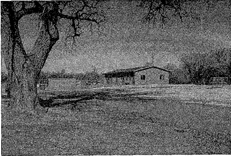
Figure 35. NHS maintenance facility. [LCA, 4/96]
