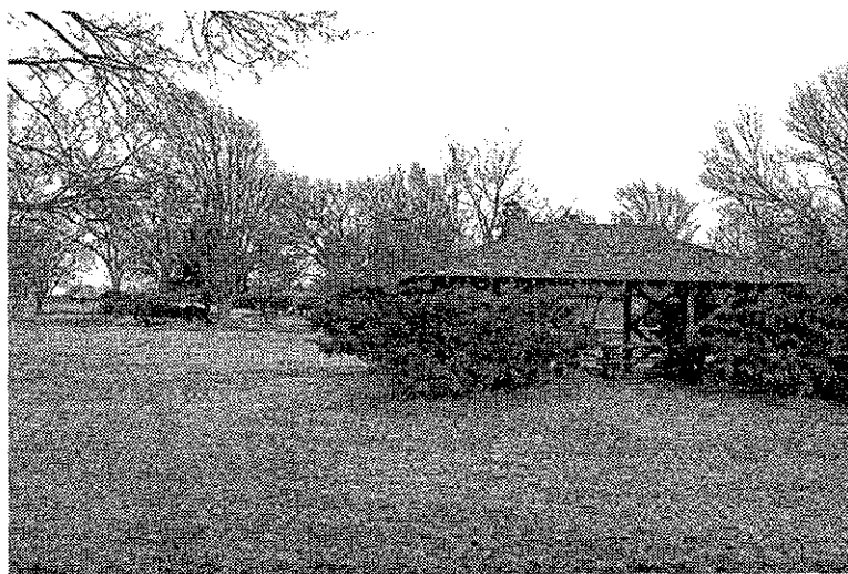
Figure 77. Timber and wood-and-steel shelters at the picnic area. [LCA, 4/96]
