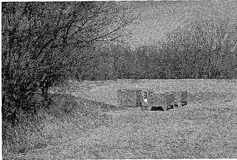
Figure 85. HVAC equipment adjacent to entry walk. [LCA, 4/96]
