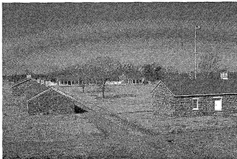
Figure 32. Parade ground seen from the roof of the blockhouse. [LCA, 4/96]
