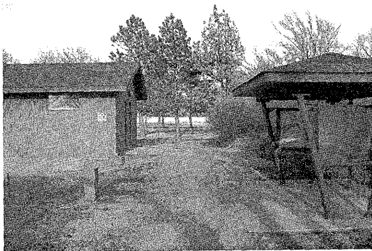
Figure 65. Restroom building and exhibit shelter at picnic area. [LCA, 4/96]
