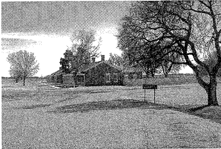
Figure 57. Service road south of entrance bridge. [LCA, 4/96]
