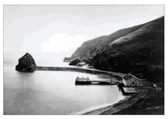
some protection to the cove from the currents of the open bay. Within this protected area, a small wharf was constructed which had a sixty-foot front of crib work covered with plank. (Photo SH1) Supplies and materials were barged in from San Francisco and unloaded at the wharf, and a steamer was used to transport personnel.<sup>15</sup>
