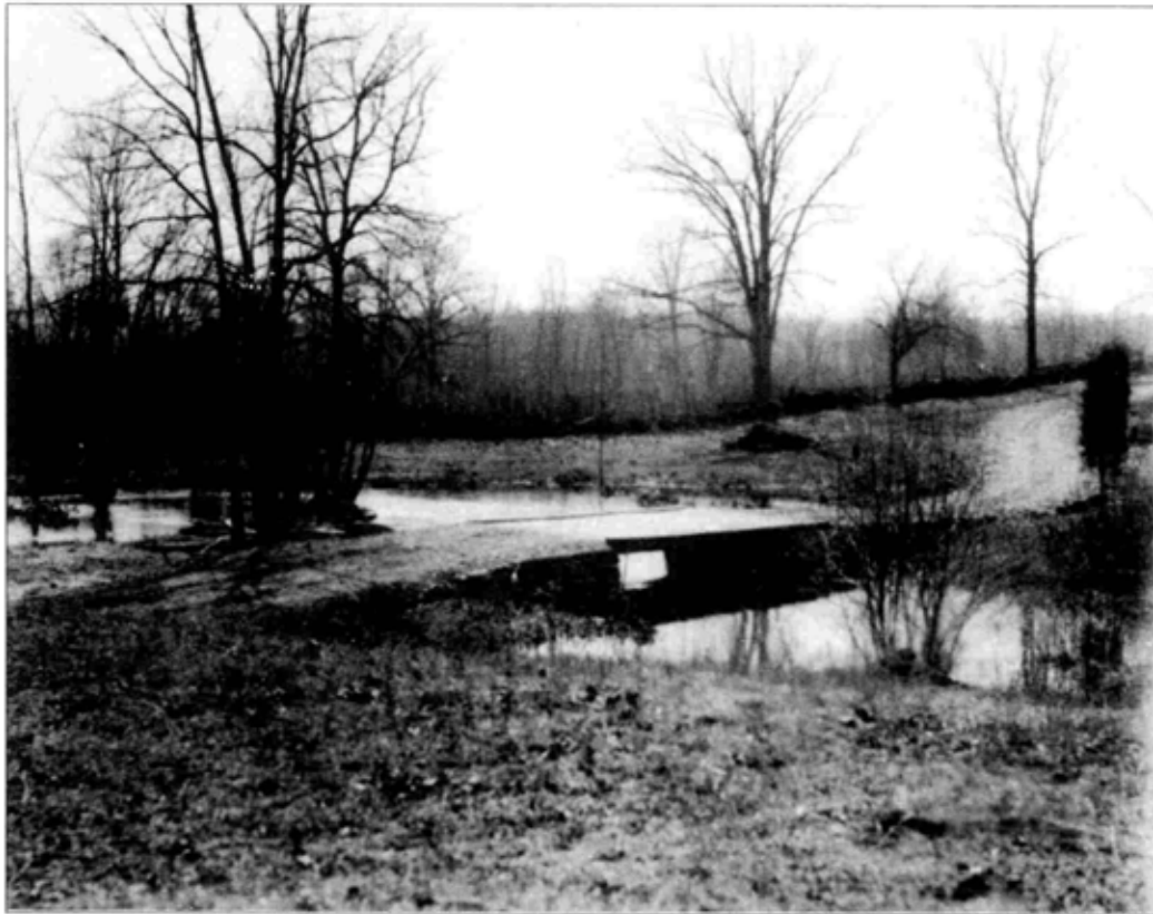
Figure 3.1. A 1925 photo looking southwest from the Stone Cottage site after brush clearing of the area was complete. Notice the stone wall in the background that separated the Bennett and Tompkins Farms. FDRL 48 22 4039 (6).
