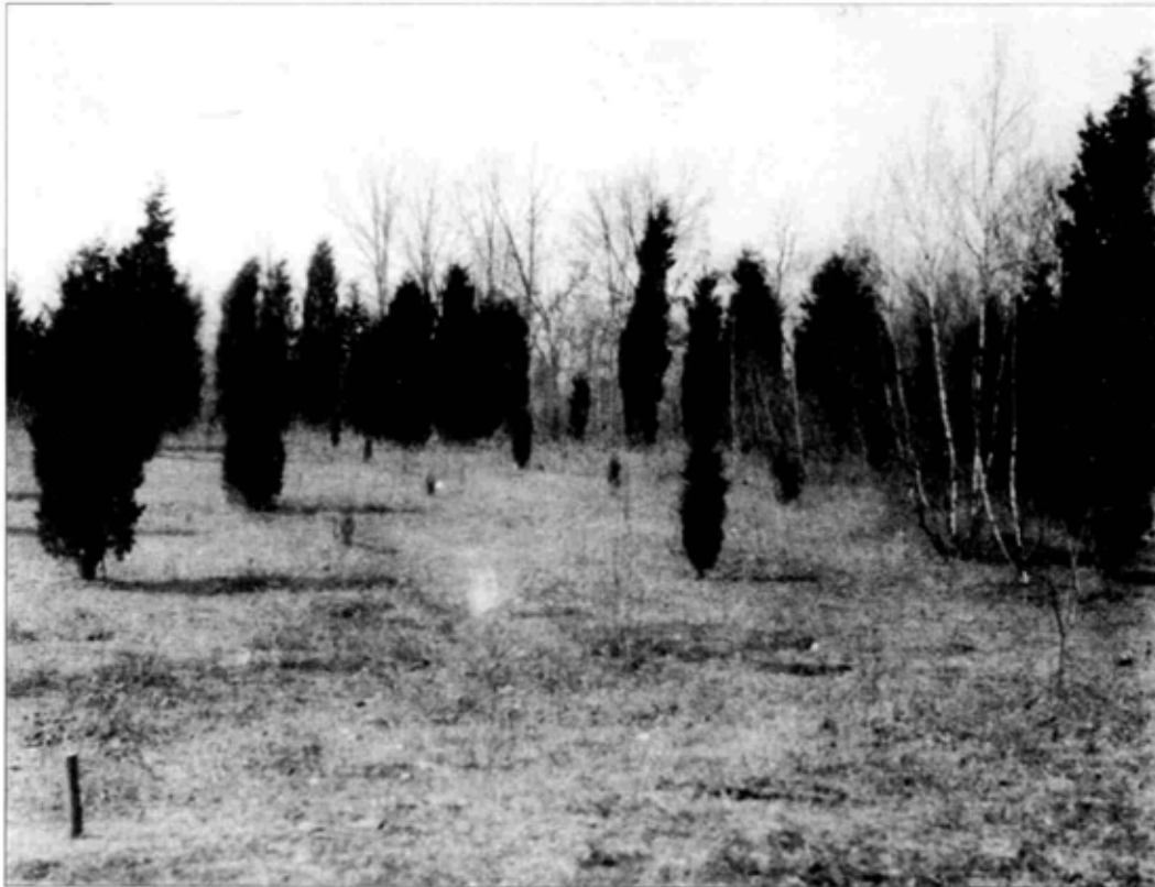
Figure 2.6. The Val-Kill site just before construction of the Stone Cottage, 1925. Note the birch and cedar trees and relatively little undergrowth. FDRL 48 22 4039 (3).
