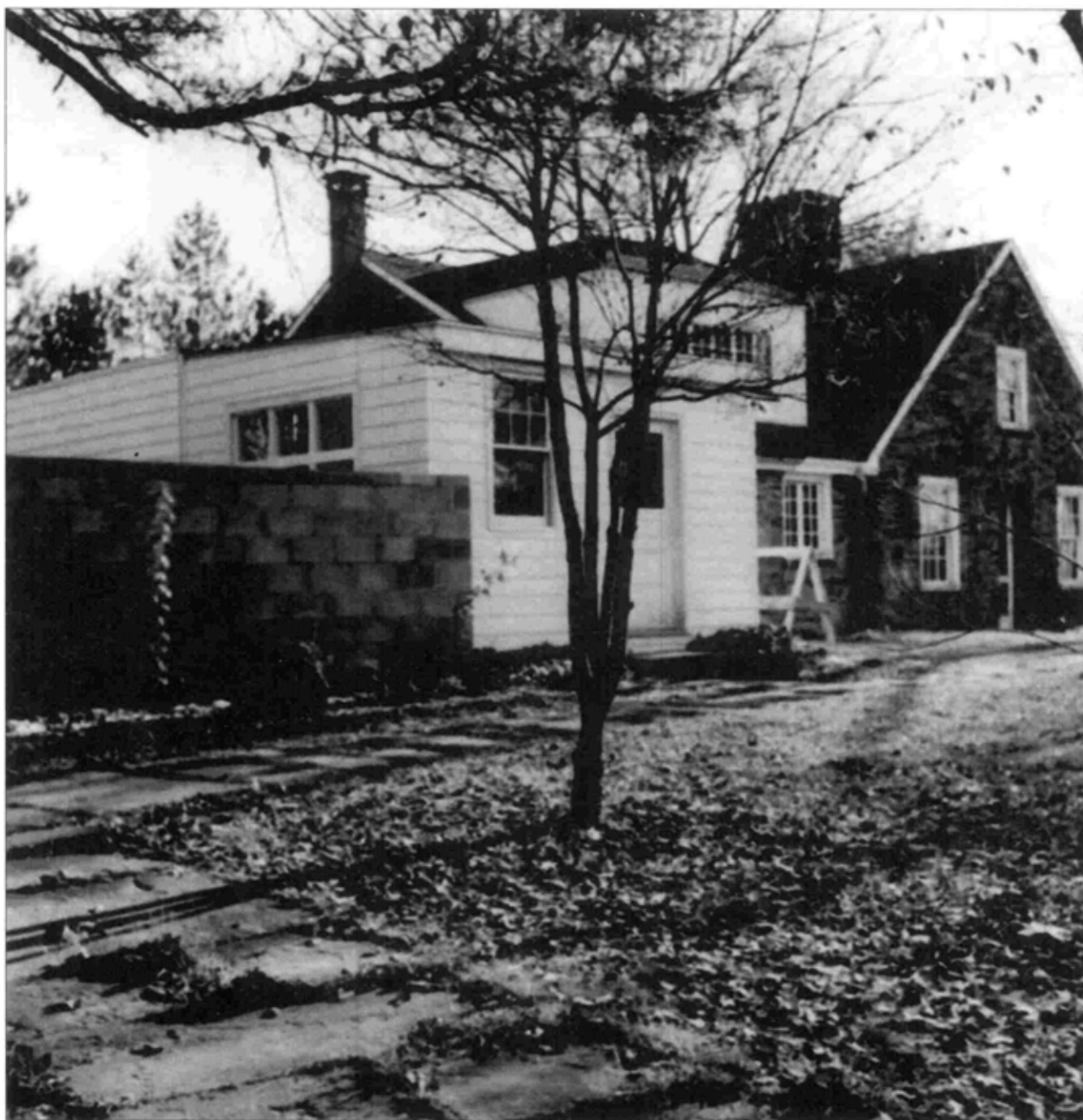
Figure 4.14. Stone Cottage, 1961. This photo, taken a year before Mrs. Roosevelt's death, shows the laundry room addition and concrete-block wall installed by John Roosevelt. The formal gardens designed by Nancy Cook no longer remain along the north side of the cottage. FDRL 65 332 (a).
