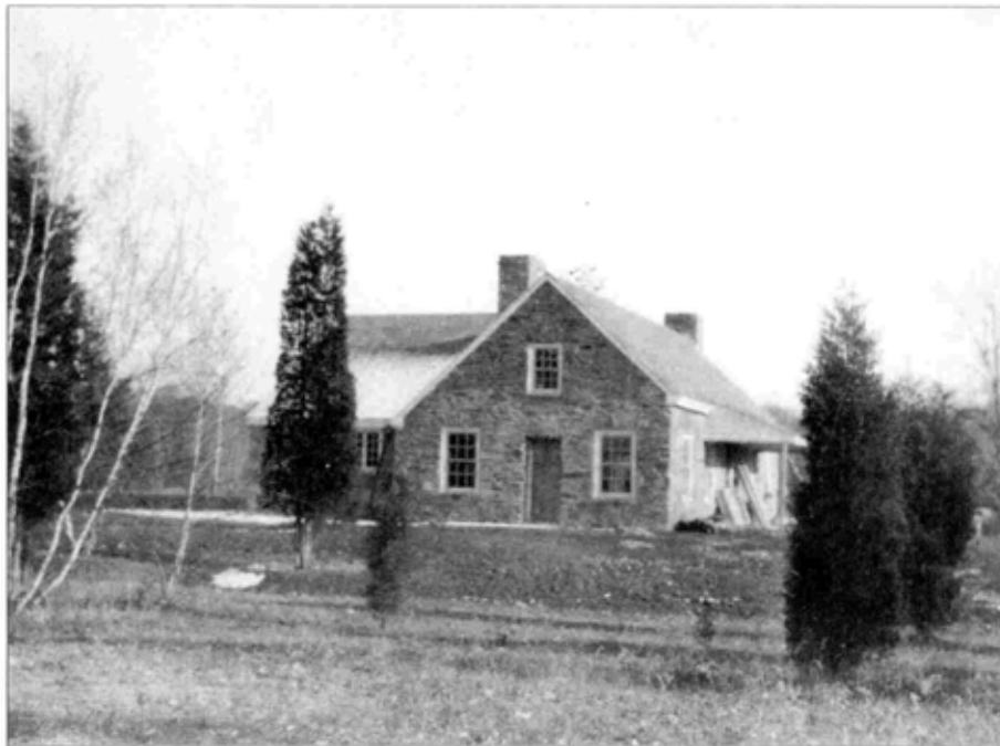
Figure 3.6. Stone Cottage under construction in 1926. Areas north of the cottage remained undisturbed, witnessed by the birch and cedar trees in the foreground. Cook-Dickerman Collection, 779. ROVA Archives.
