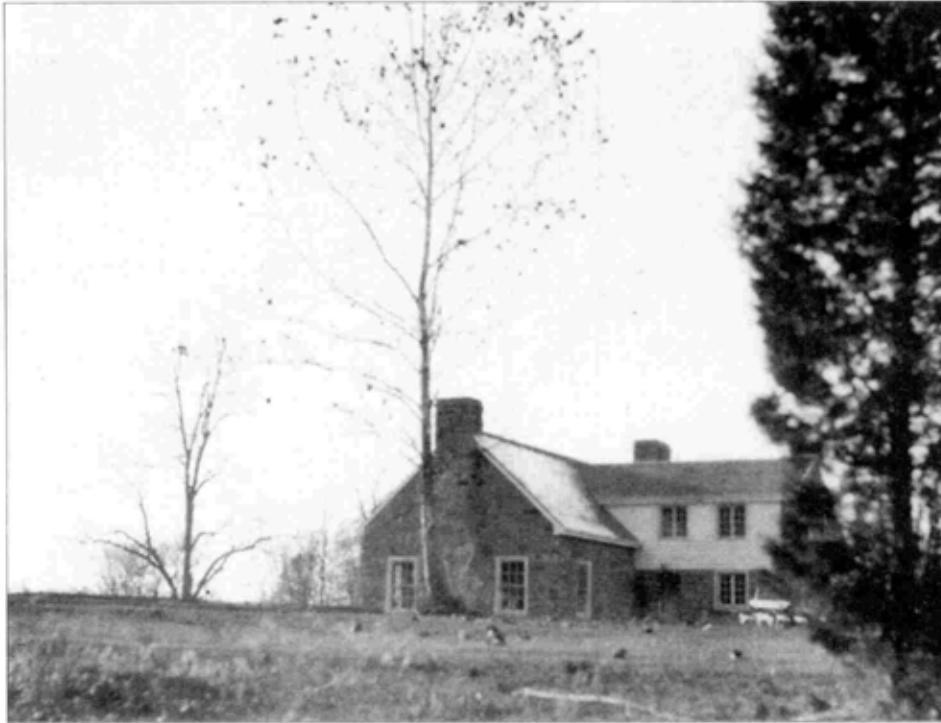
Figure 3.7. Stone Cottage as seen from the south in 1926. Notice the stumps in the foreground and cleared landscape. Only a sycamore tree remained in the vicinity of the house. Cook-Dickerman Collection, 780. ROVA Archives.
