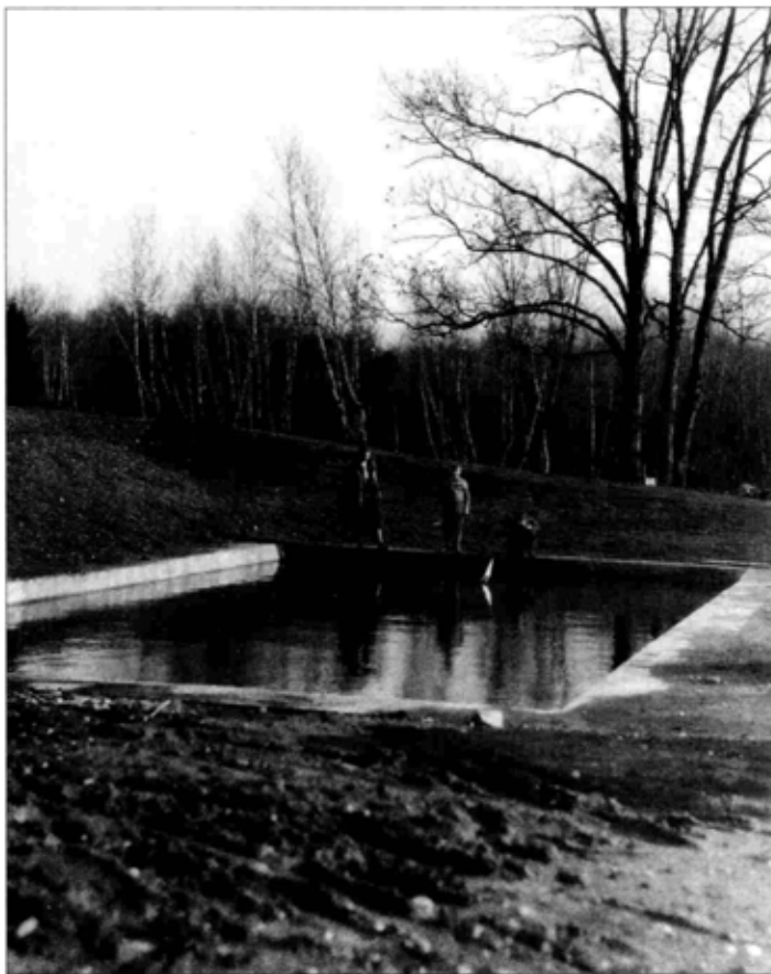
Figure 3.3. A 1925 photo of the newly completed pool located southwest of the still incomplete Stone Cottage. Notice the driveway behind the pool, connecting the bridge and Stone Cottage. Cook-Dickerman Collection, 827. ROVA Archives.
