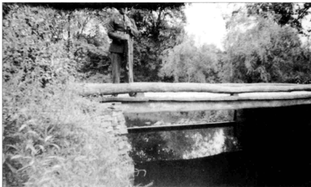
Figure 3.28. The updated bridge, circa 1935. A new deck and a low wooden railing were installed. Cook-Dickerman, 842. ROVA Archives.
