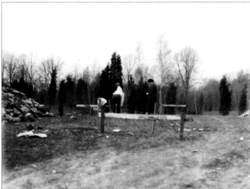
Figure 3.4. Stacking the foundation of the Stone Cottage, 1925. Cook-Dickerman Collection, 776. ROVA Archives.
