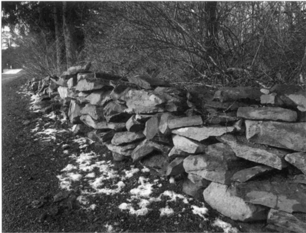
Figure 7.20. Typical stone wall at Val-Kill. This is an informal dry-laid wall created from agricultural activities (OCLP, 2003).
