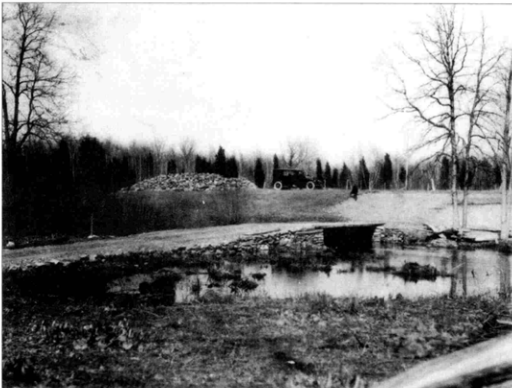
Figure 3.2. A 1925 photo looking northeast across the Fall-Kill towards the Stone Cottage construction site. Notice the improved bridge with a new plank deck and the cleared creek banks. FDRL 48 22 4039 (2).
