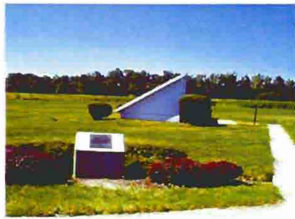
Figure 39. The Pylon building was added in 1941 to improve the visibility of the flying field from the Memorial.
