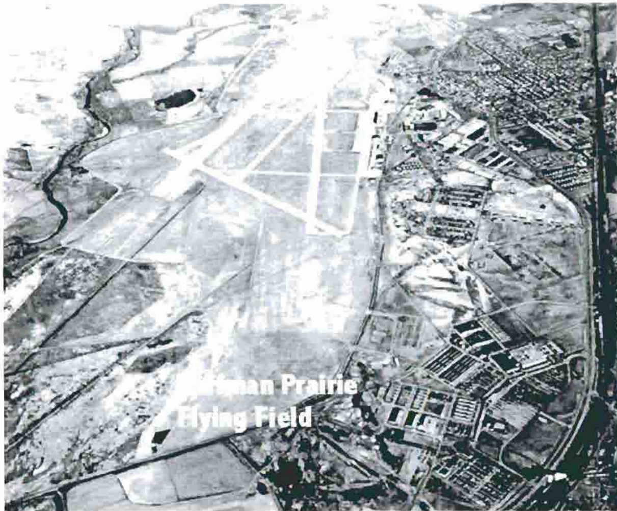
Figure 32. 1952 photo showing Huffman Prairie Flying Field and its proximity to the runways.
