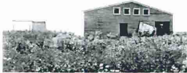
Figure 27. East and north walls of 1910 hangar, ca. 1923.
