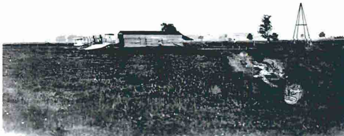
Figure 7. Huffman Prairie Flying Field, flight number 19. This photograph shows the 1905 hangar and flyer and the launching catapult.
