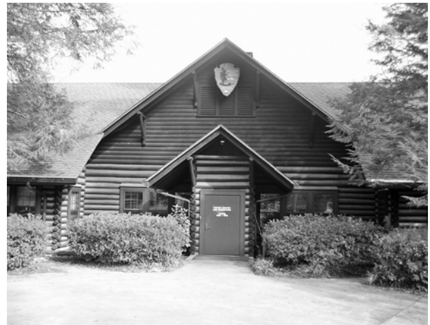
FIGURE 40. View of front entrance to Island Ford Lodge. (Marti Gerdes, NPS-SERO-CRD, 2005)
