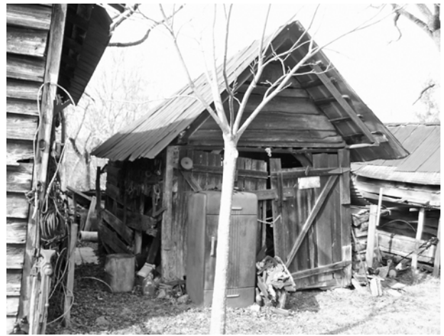
FIGURE 13. View west-northwest of gear house. (Marti Gerdes, NPS-SERO-CRD, 2005)
