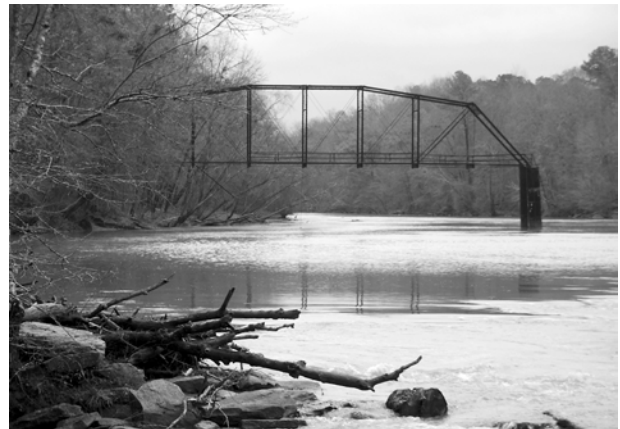
FIGURE 3. View north of Jones Bridge. (Marti Gerdes, NPS-SERO-CRD, 2005)
