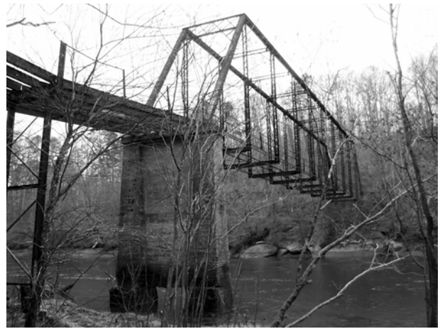
FIGURE 2. View at east end of Settles Bridge. (Marti Gerdes, NPS-SERO-CRD, 2005)
