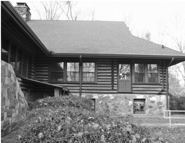
FIGURE 39. View of rear wing of Island Ford Lodge. (Marti Gerdes, NPS-SERO-CRD, 2005)
