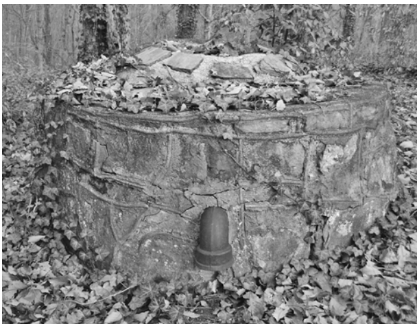
FIGURE 36. View of well at Collins-Yardum House. (NPS-SERO-CRD, 2005)
