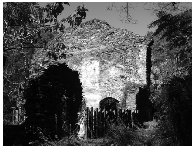
FIGURE 25. View of Marietta Paper Company Mill #1. (Marti Gerdes, NPS-SERO-CRD, 2005)
