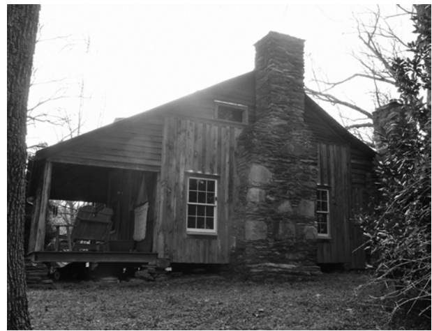
FIGURE 17. View of east end of George Power House. (Marti Gerdes, NPS-SERO-CRD, 2005)
