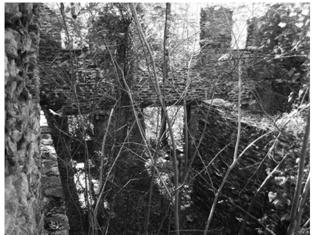
FIGURE 24. View of Marietta Paper Company Mill #1 (Marti Gerdes, NPS-SERO-CRD, 2005)
