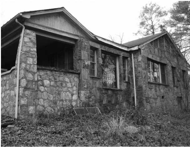
FIGURE 34. View of east side of Collins-Yardum House. (NPS-SERO-CRD, 2005)
