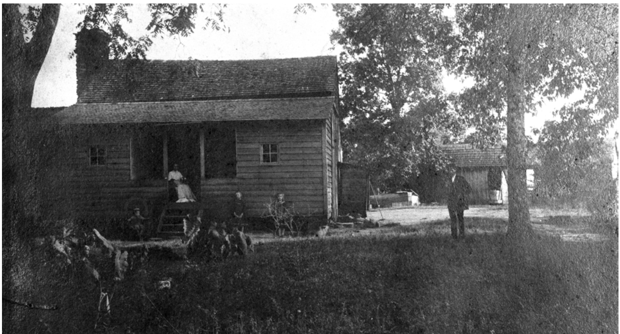
FIGURE 10. View south of James C. Power house at what is now known as Hyde Farm, late 1800s. (Vanishing Georgia Collection, Georgia Department of Archives and History)
