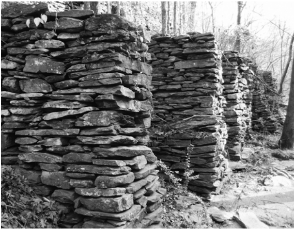
FIGURE 27. View of piers of millrace to Mill #1. (Marti Gerdes, NPS-SERO-CRD, 2005)
