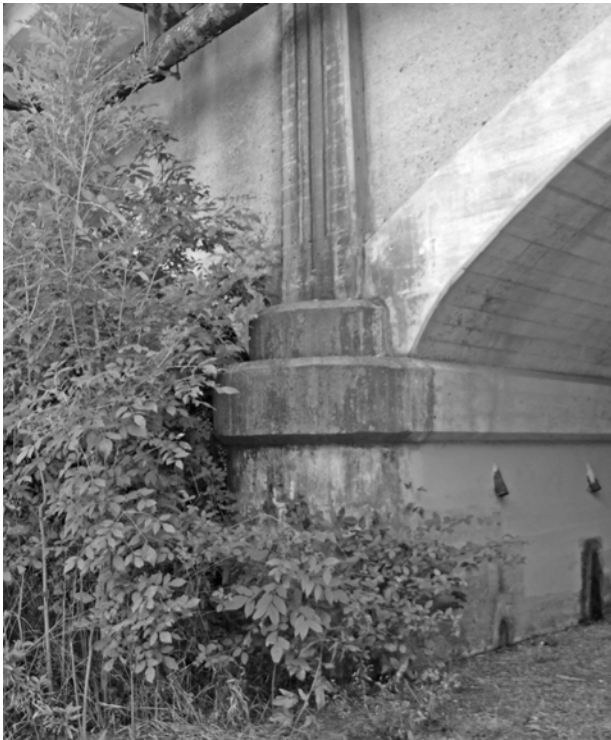
FIGURE 5. View of typical buttress in Roswell Road bridge. (T. Jones, NPS-SERO-CRD, 2006)
