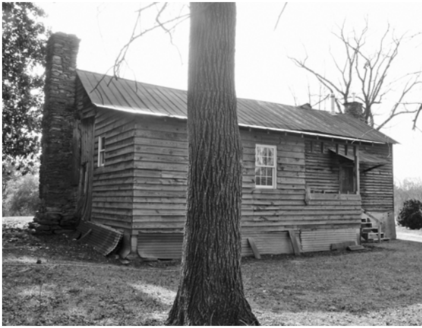
FIGURE 6. View south-southwest of Hyde House. (Marti Gerdes, NPS-SERO-CRD, 2005)
