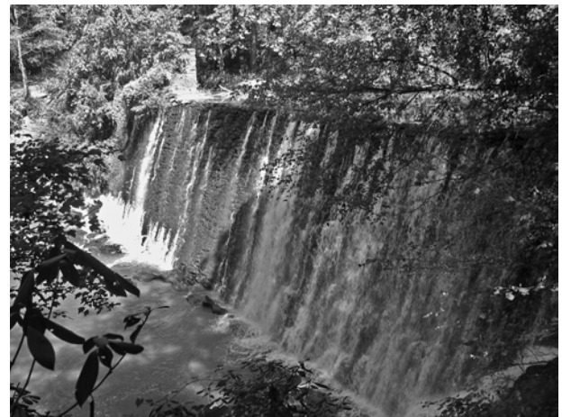
FIGURE 20. View of the main dam for the Roswell Manufacturing Company's mills.
