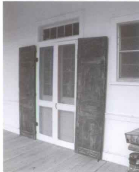
Figure 37 Typical French doors with solid wooden shutters. (NPS-SERO-CRS, 2001)
