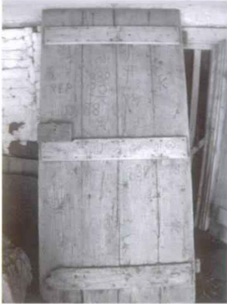
Figure 51 View of board door at basement level, typical of the oldest doors in the house. (NPS-SERO-CRS, 2001)
