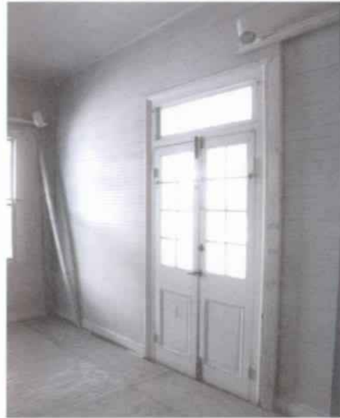
Figure 81 View of French doors in Room 207, which are of a different era from the other French doors in the house. (NPS-SERO-CRS, 2001)
