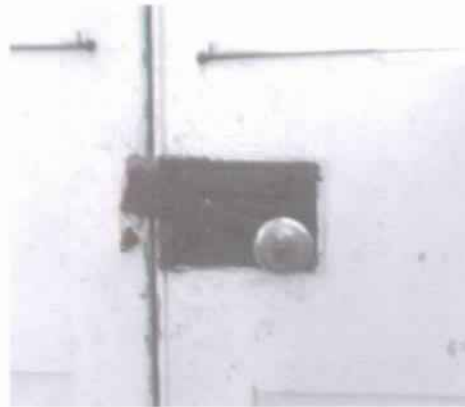
Figure 53 Early spring lock on French doors in dining room. (NPS-SERO-CRS, 2001)
