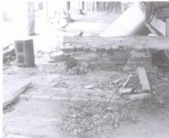
Figure 32 Demolished foundation for fireplaces under kitchen wing. (NPS-SERO-CRS, 2001)
