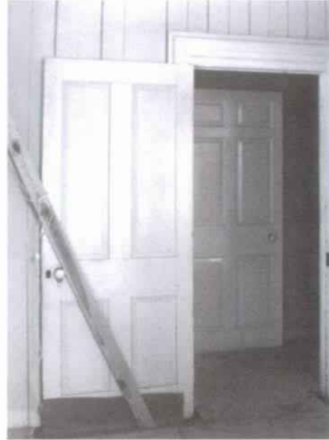
Figure 52 View of four-panel door from 1880s and, through doorway, typical six-panel door from 1830s. (NPS-SERO-CRS, 2001)
