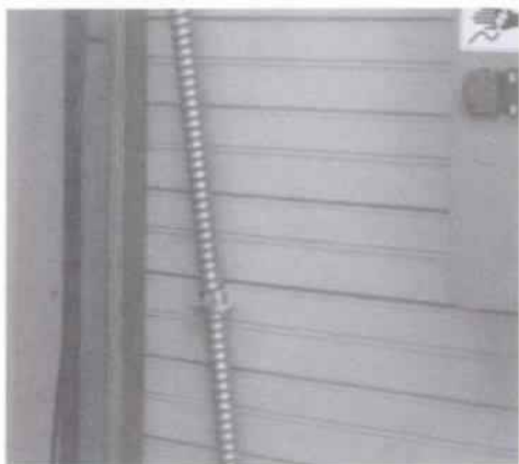
Figure 50 Typical beaded, tongue-and-groove boards used to panel parts or all of walls and ceilings in 202, 204, 207, 209, 215, and 216. (NPS-SERO-CRS, 2001)
