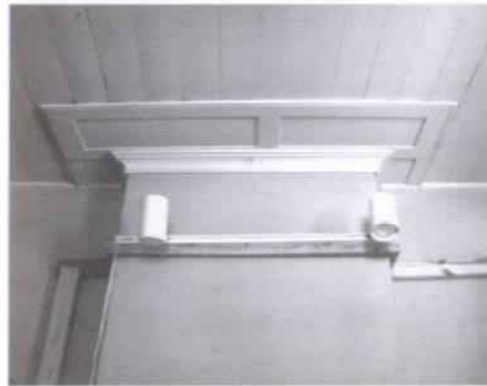
Figure 75 View of paneling at chimney breast in front bedroom (205). (NPS-SERO-CRS, 2001)
