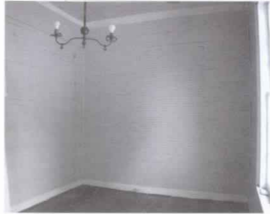
Figure 94 View southwest in stranger's room, showing window that was closed when sitting area was created at north end of kitchen in 1964. (NPS-SERO-CRS, 2001)
