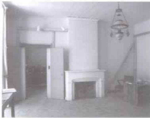
Figure 76 View south in parlor (206), showing door to front bedroom. (NPS-SERO-CRS, 2001)
