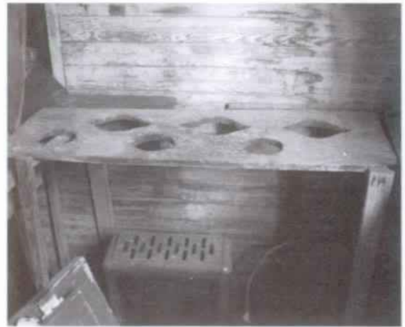
Figure 109 View of wooden shelf for pots next to kitchen sink. (NPS-SERO-CRS, 2001)
