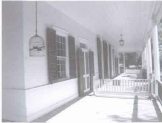
Figure 42 View north on front or east gallery. (NPS-SERO-CRS, 2001)
