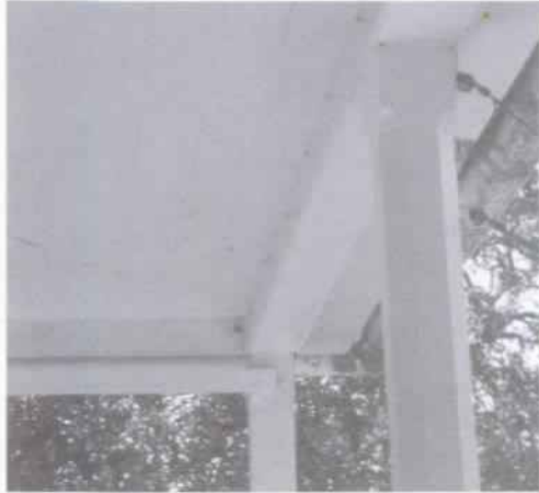
Figure 46 View of typical porch header and column top. (NPS-SERO-CRS, 2001)
