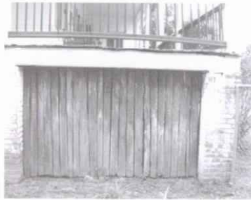
Figure 41 View of the third type of foundation enclosure. (NPS-SERO-CRS, 2001)
