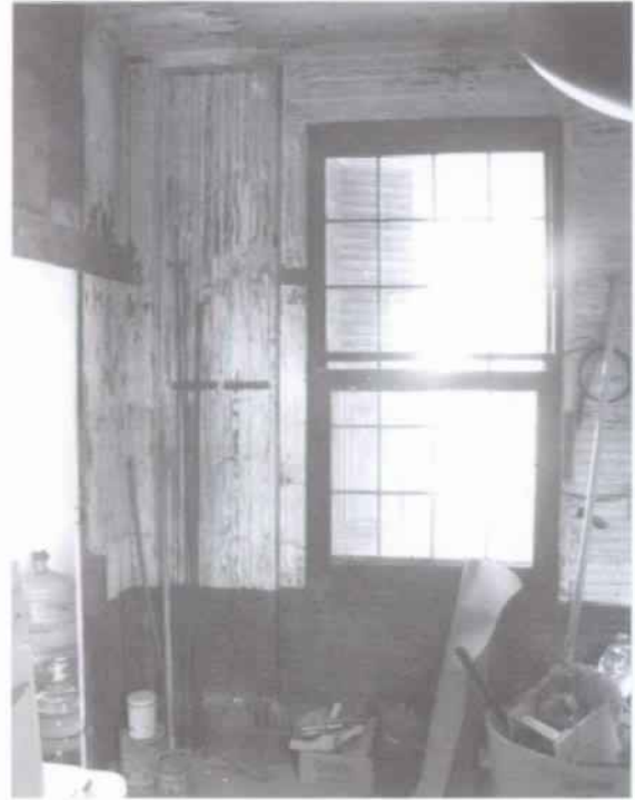
Figure 108 View of southeast corner of old kitchen; paneled inset to left of window may have contained a water-heating apparatus. (NPS-SERO-CRS, 2001)
