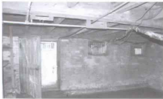
Figure 59 View to north in 104, showing door exiting beneath north gallery. (NPS-SERO-CRS, 2001)
