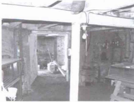
Figure 56 View to east of north side of "Museum" in 102. (NPS-SERO-CRS, 2001)
