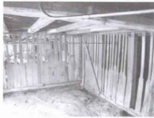
Figure 40 View of a somewhat of foundation enclosure. (NPS-SERO-CRS, 2001)
