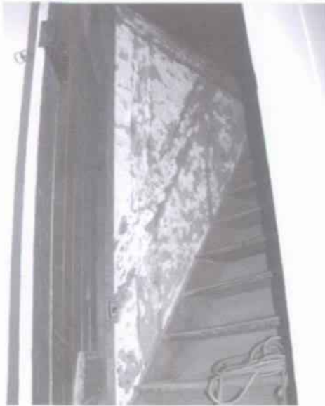
Figure 34 View of timber-framed bousillage construction, whitewashed, visible in stairwell to attic. (NPS-SERO-CRS, 2001)
