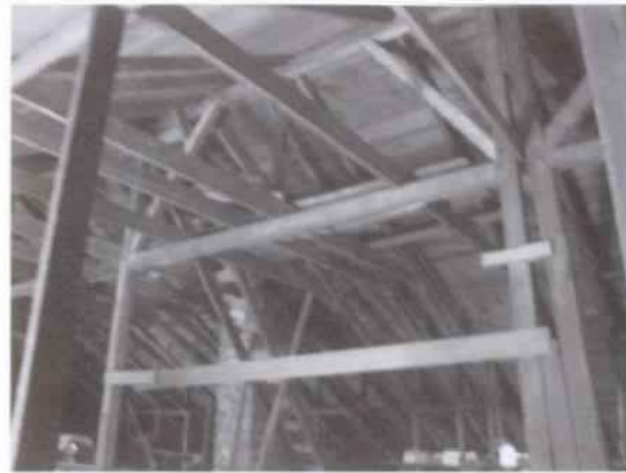
Figure 35 View to southwest in attic, showing original roof framing. (NPS-SERO-CRS, 2001)
