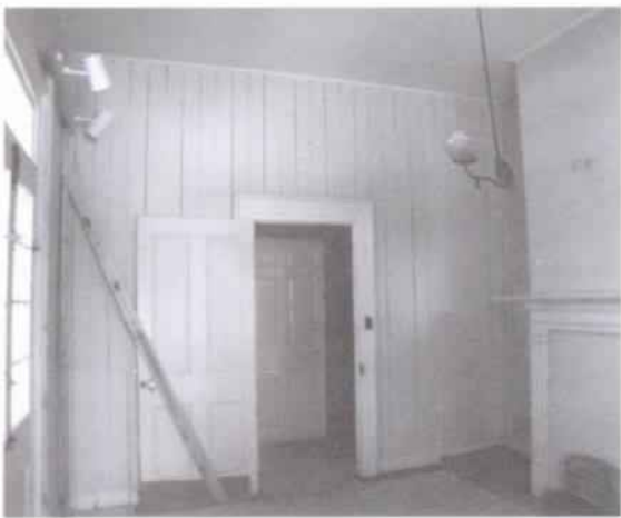
Figure 80 View south in Room 207 showing wall added c. 1880 to create central hall. (NPS-SERO-CRS, 2001)
