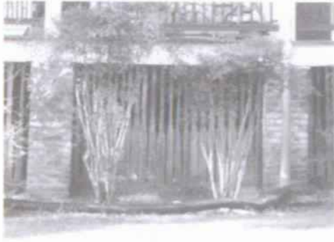
Figure 39 Views of earliest type of foundation enclosures, (c. 1870). (NPS-SERO-CRS, 2001)
