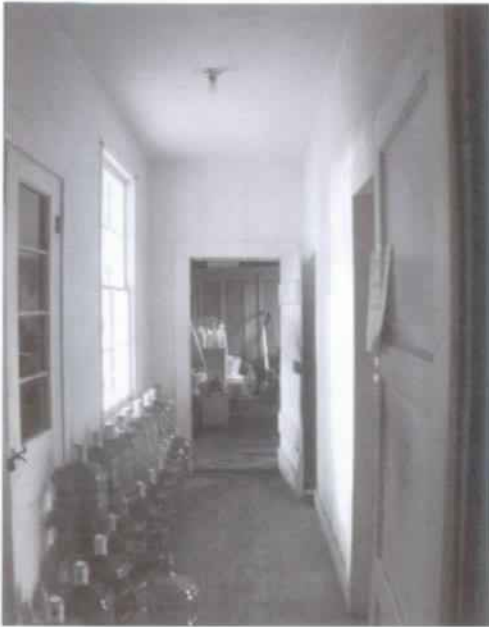
Figure 110 View of hall from east toward old kitchen. (NPS-SERO-CRS, 2001)
