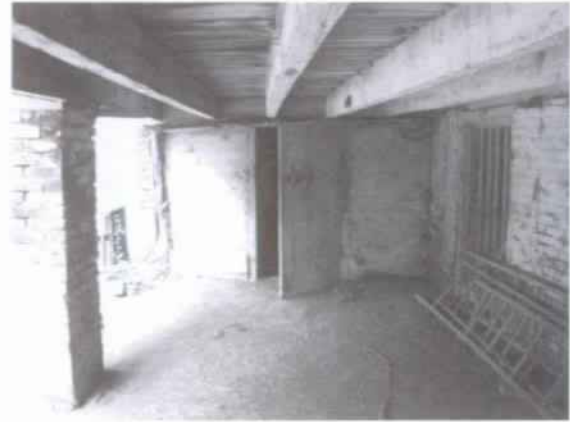
Figure 64 View west under south gallery, showing door to gas room. (NPS-SERO-CRS, 2001)
