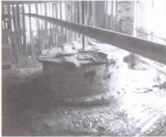
Figure 29 View of cistern beneath rear gallery. (NPS-SERO-CRS, 2001)
