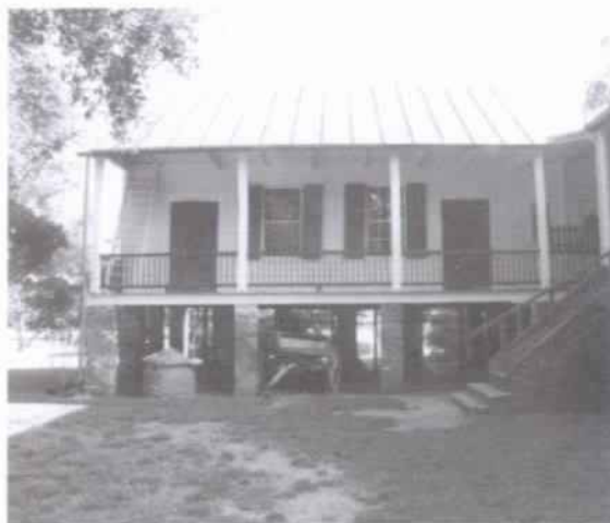
Figure 28 View of south side of old kitchen (c. 1865) off west side of main house. (NPS-SERO-CRS, 2001)
