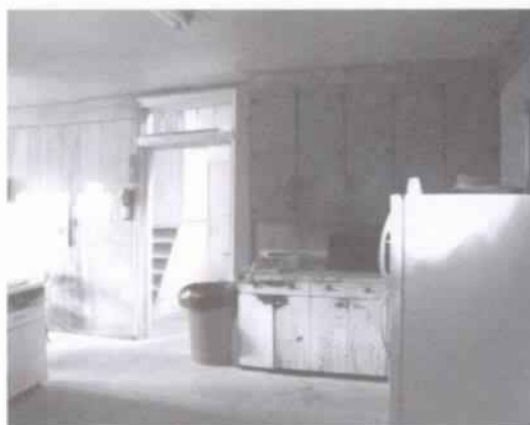
Figure 102 View to east in kitchen, showing connection to Room 212. (NPS-SERO-CRS, 2001)
