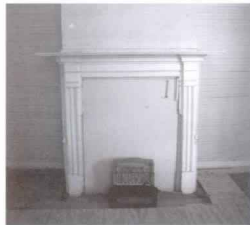
Figure 82 View of mantelpiece in Room 207, one of two antebellum mantles remaining in the house. (NPS-SERO-CRS, 2001)
