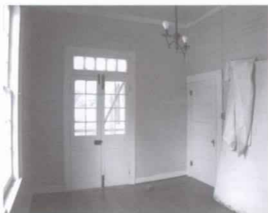
Figure 93 View east in stranger's room (Room 211). (NPS-SERO-CRS, 2001)
