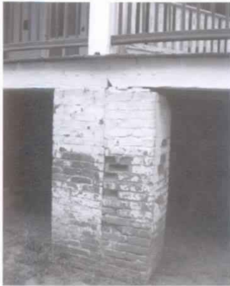
Figure 31 Brick piers on north end of east gallery. Pier at left is from the original house, c. 1821; pier at right is from the first expansion of the house, c. 1825. (NPS-SERO-CRS, 2001)
