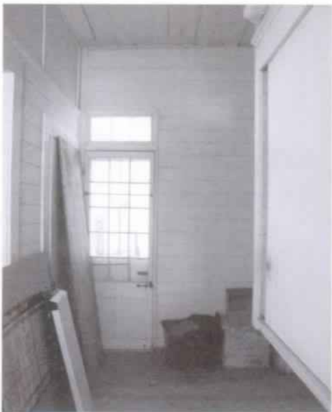
Figure 66 View to north in dressing room. (NPS-SERO-CRS, 2001)
