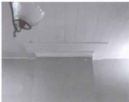
Figure 92 View of paneling at chimney breast in dining room. (NPS-SERO-CRS, 2001)
