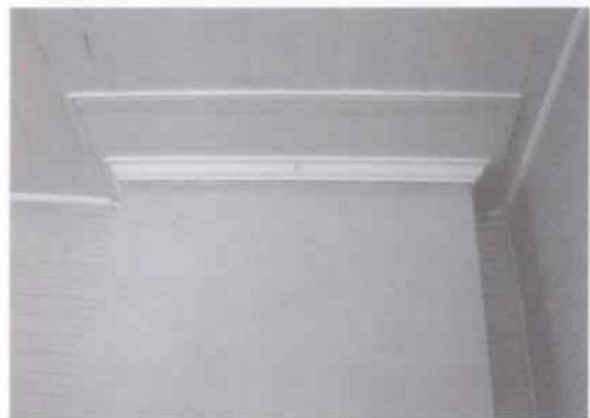
Figure 69 Top, view of mantel piece in master bedroom; below, view of chimney breast and ceiling paneling. (NPS-SERO-CRS, 2001)
