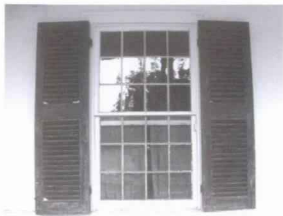
Figure 38 Typical 12/12, double-hung window with louvered shutters, c. 1835. (NPS-SERO-CRS, 2001)
