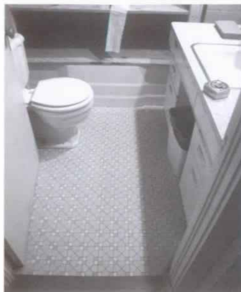
Figure 71 View of bathroom floor. (NPS-SERO-CRS, 2001)
