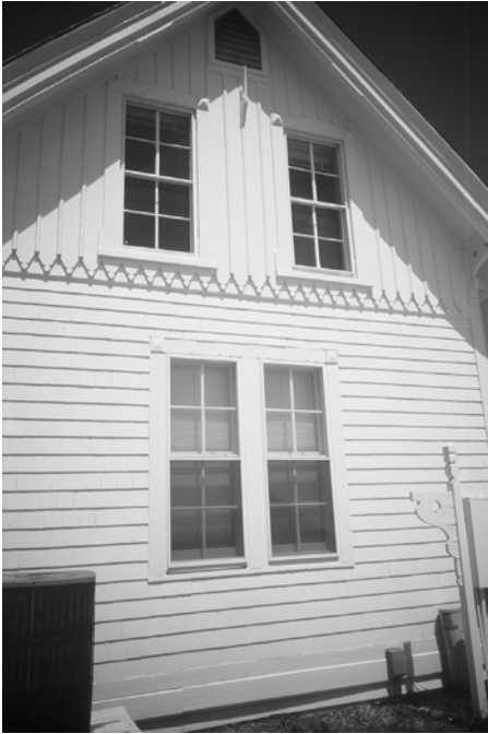
Figure C-4 South gable of the station
