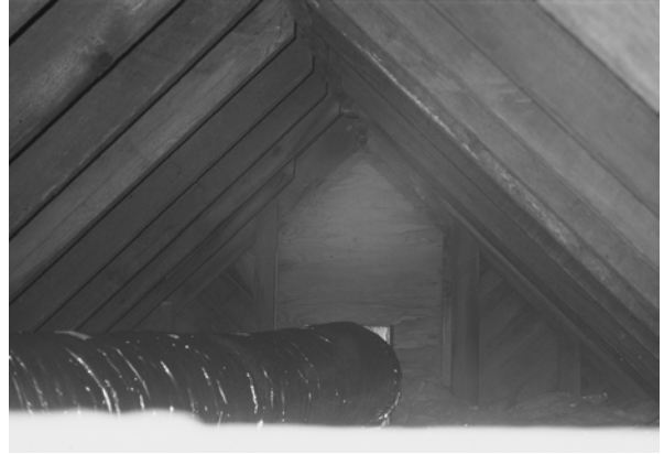
Figure C-5 Attic of the station
