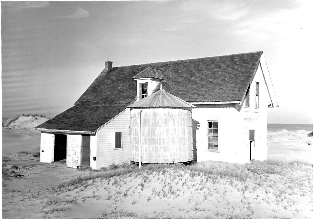
I.15 1879 Station from the southwest, Jan. 10, 1955. Label – “Neg. No: 55-16, Date: 1/10/55, Print File: St/M, General Description, Location, Other pertinent Data: Supt. Residence prior to being moved. Negative by: A.D.” [Albert Dillahunty]
