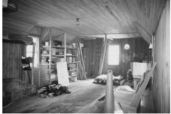
Figure C-27 View of boat house Room 101, looking northeast
