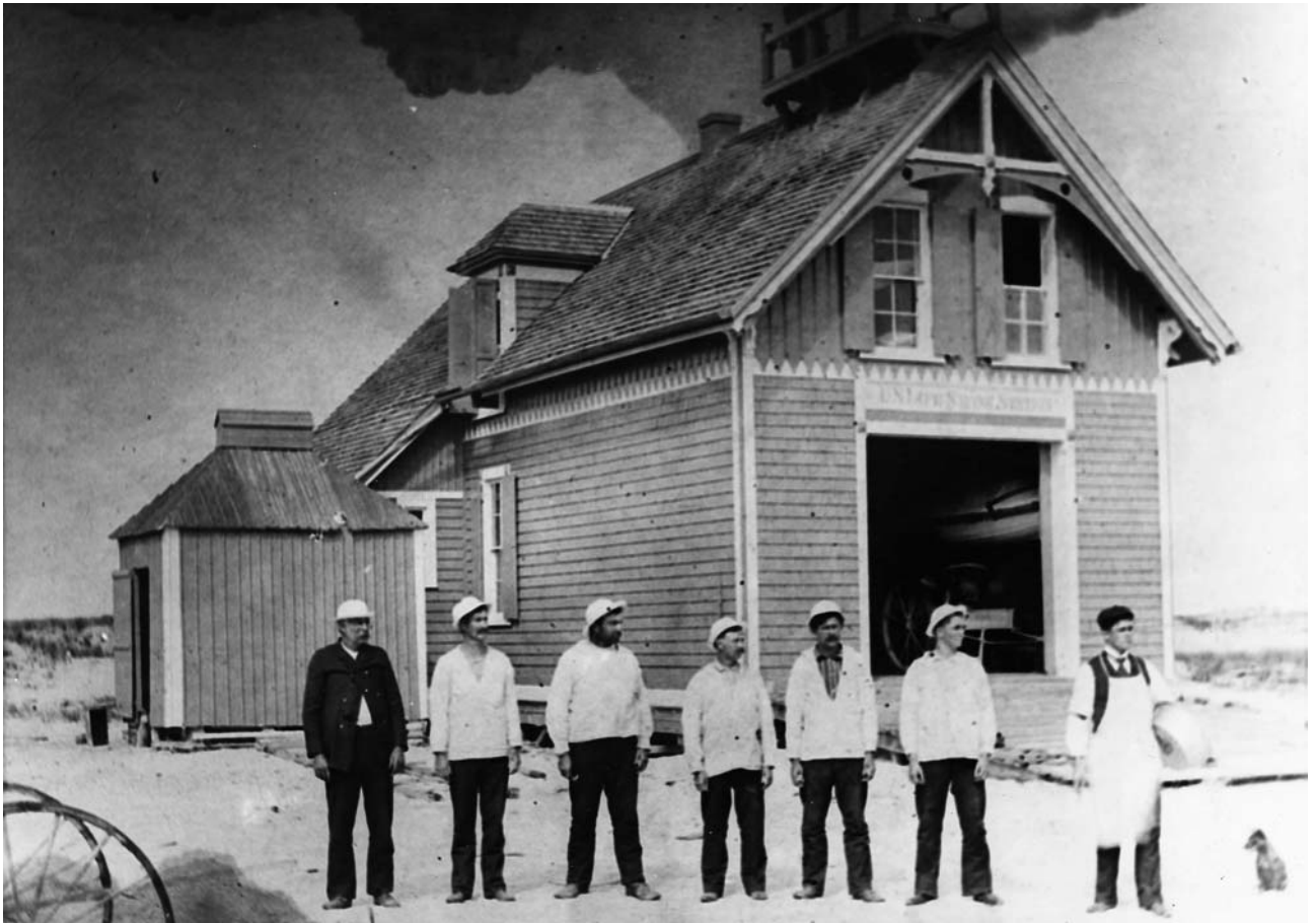
I.3 1879 Bodie Island Life Saving Station from the southeast; crewmembers not identified. Ca. 1898 based on damage to outbuilding roof similar to photo number 1 above. Courtesy of Outer Banks History Center.
