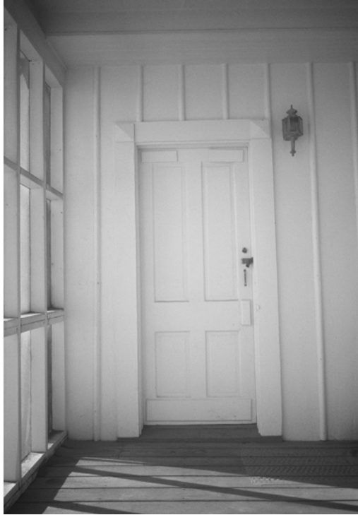
Figure C-25 Door on south elevation of boat house
