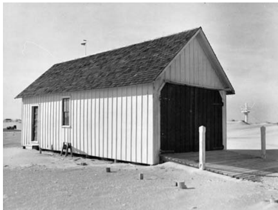
Figure A-9 1916 Boat House, c. 1955, unknown photographer; archives of the National Park Service, Outer Banks Group
