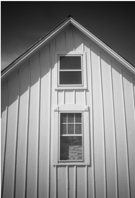
Figure C-26 Windows on east elevation of boat house
