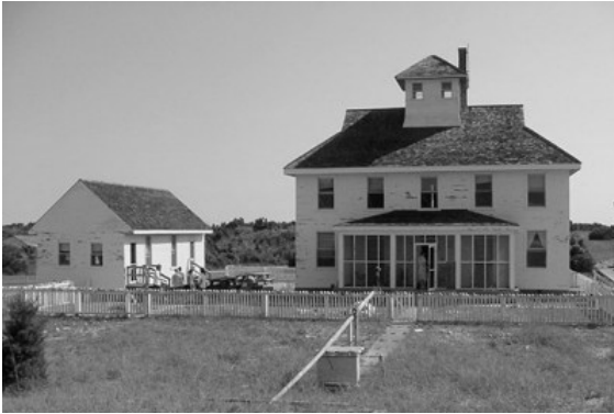
Figure B-3 Chatham Type station at Cape Lookout (Cape Lookout Studies website)
