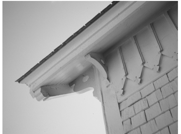
Figure C-2 Bracket and fascia detail
