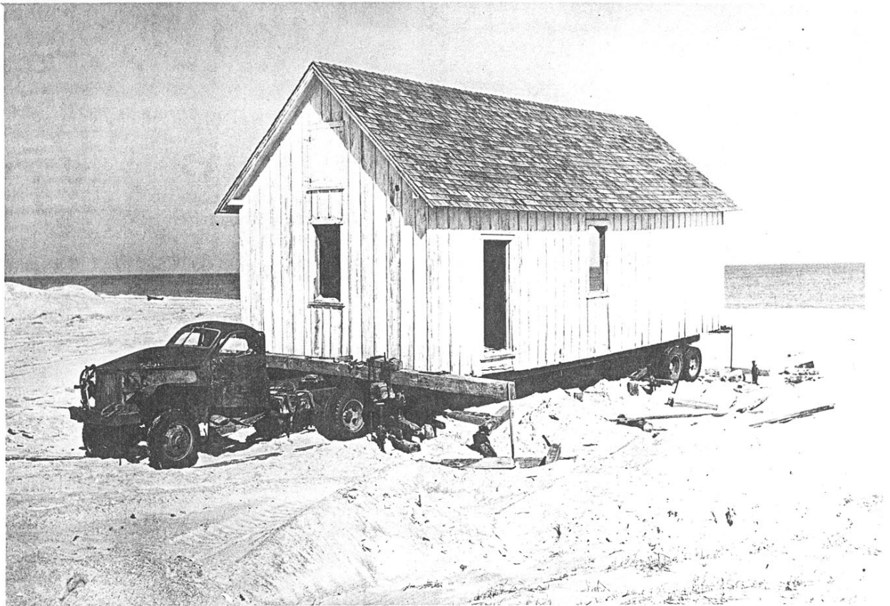
I.20 1916 boat house from the southwest, Feb. 8, 1955. Label – “Neg. No: 55-?, Date: 2/8/55, Print File: St/M, General Description, Location, Other pertinent Data: B.I. Boat House (Supt. garage) being moved. Negative by: Albert Dillahunty Large print?” Shows north and west elevations.
