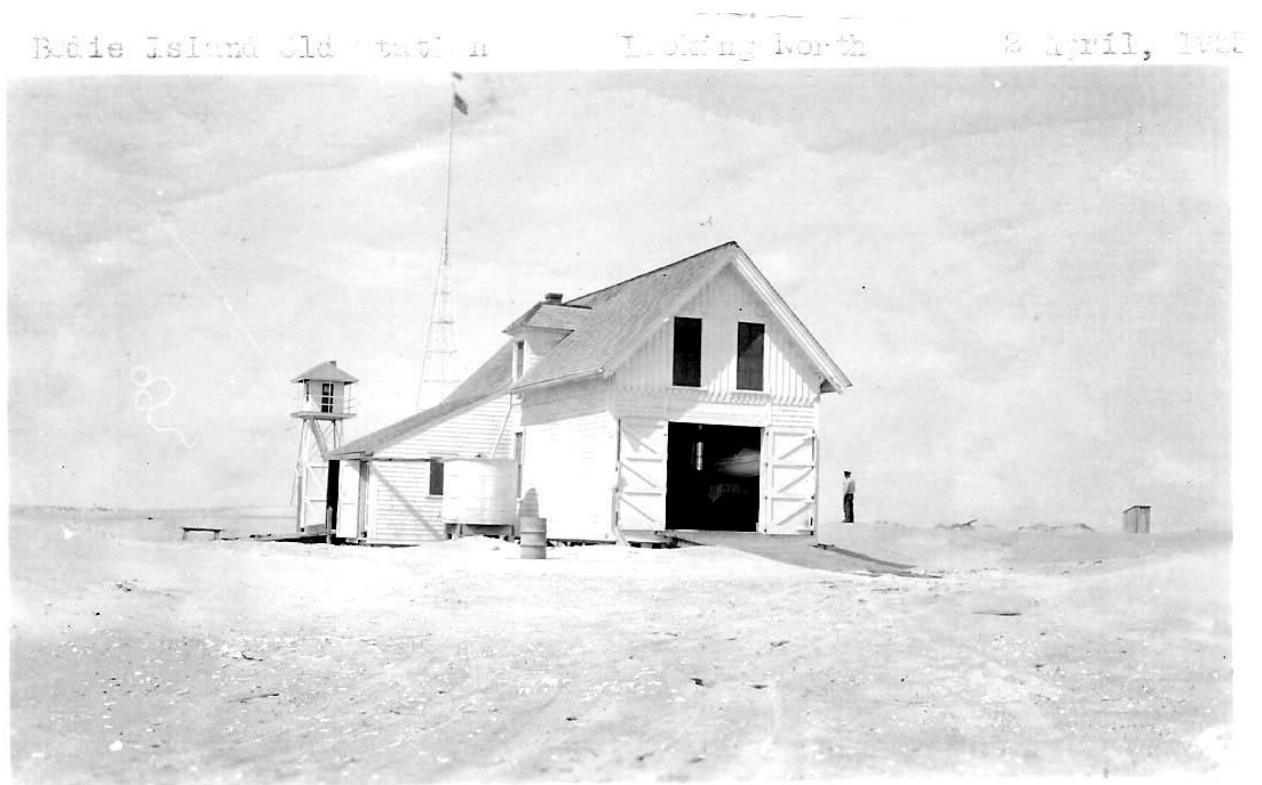
I.7 1879 Station from the southeast dated April 2, 1935. Label - “Bodie Island Old Station Looking North, 2 April 1935.” Shows station without tower and with enlarged 1925 lean-to, 1925 lookout tower in place, and radio/flag tower.
