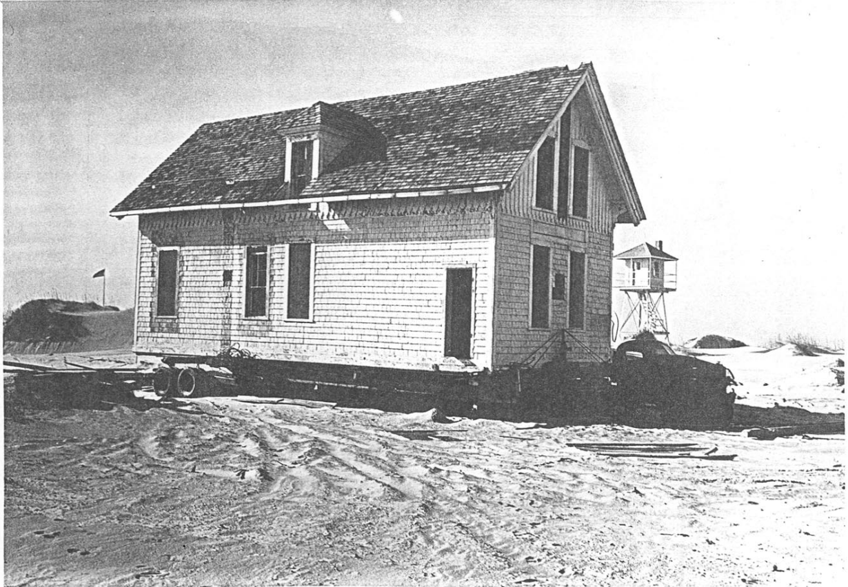
I.19 1879 Station from the east, Jan. 31, 1955. Label – “Neg. No: 55-21, Date: 1/31/55, Print File: St/M, General Description, Location, Other pertinent Data: Supt. Residence being moved. Negative by: A.D.” [Albert Dillahunty]. Shows east facade with two south windows added, original window under the dormer, door added at the north end, and scar of exterior chimney in north gable end.
