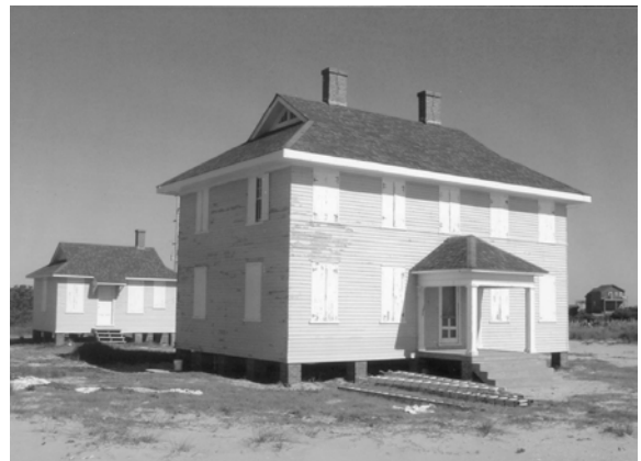
Figure B-2 Privately owned Chatham Type station at Creed's Hill, Frisco, now a residence (© Stephen Wilmoth, October 2004)
