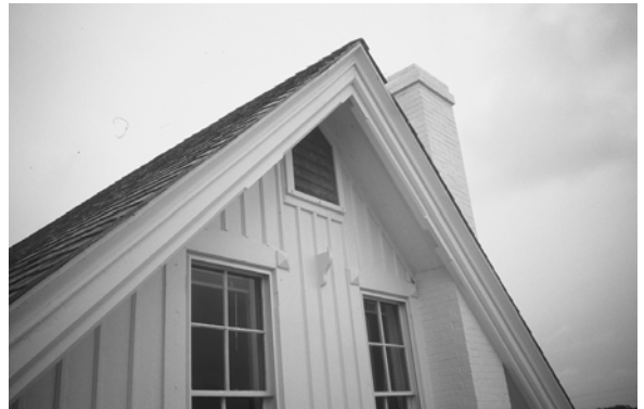
Figure C-6 Detail of north gable end and chimney
