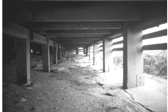
Figure C-22 Foundation and floor structure of the boat house, looking west
