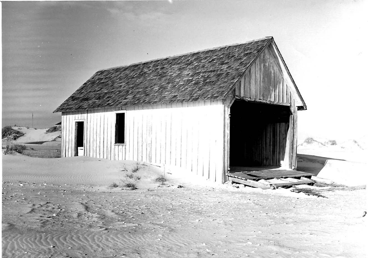
I.17 1916 boat house from the southeast, Jan. 31, 1955. Label – “Neg. No: 55-18, Date: 1/31/55, Print File: St/M, General Description, Location, Other pertinent Data: Old Bodie Island C. G. boat house prior to being moved into location for Supt’s garage. Negative by: Albert Dillahunty Large print? Yes”. Shows south and east elevations.
