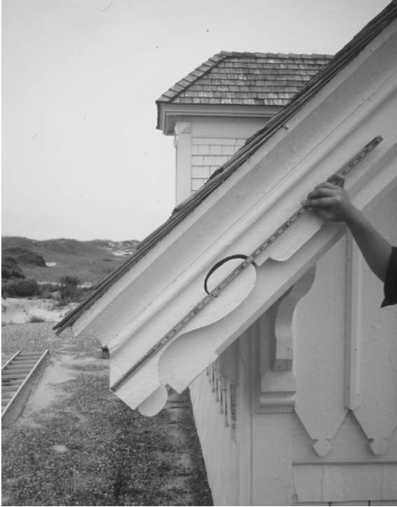
Figure C-7 Detail of fascia and rake boards
