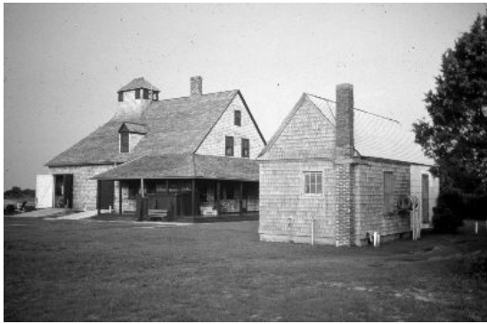
Figure B-4 Quonochontaug Type Station at Portsmouth Village (Portsmouth Village website, CALO)
