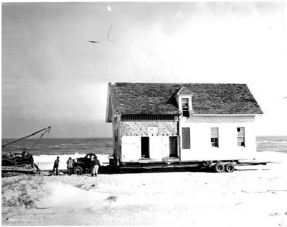
Figure B-5 Moving the Station, January 31, 1955, photo by Albert Dillahunt, NPS archives, Outer Banks Group, negative number 55-20
