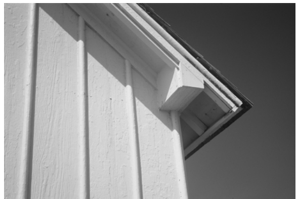
Figure C-24 Fascia and wall of boat house
