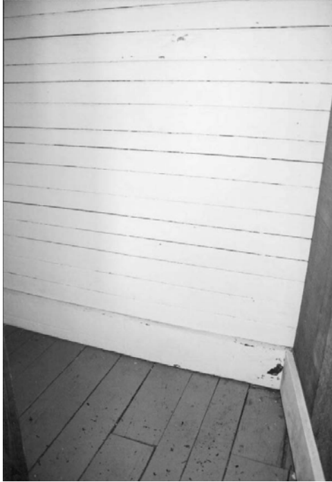
Figure C-18 Closet in Room 204A, showing early flooring and beaded wall board
