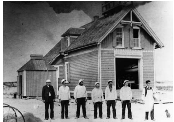
Figure B-7 c. 1885 appearance of Bodie Island Life-Saving Station, unknown date (Outer Banks History Center)
