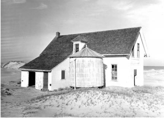
Figure B-7 Bodie Island Station, January 10, 1955, photographer Albert Dillahunt, NPS archives, Outer Banks Group, negative no. 55-17
