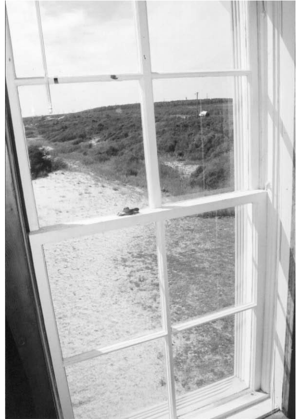
Figure C-19 Window muntins in Room 204A
