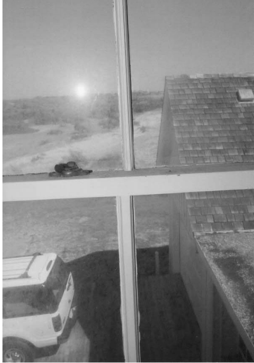
Figure C-16 Window muntins in Room 201
