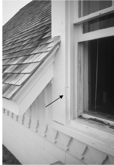
Figure C-9 Detail of dormer window with shutter hinge mark
