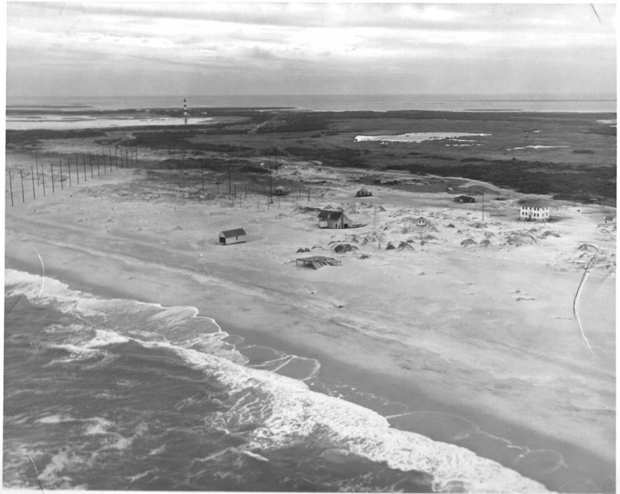
I.9 Aerial view of Station, September 1948, from the northeast. Shows LORAN system in place. Water storage tanks removed from 1925 Station.
