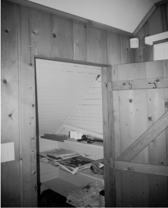
Figure C-20 View into Room 204B from Room 204A
