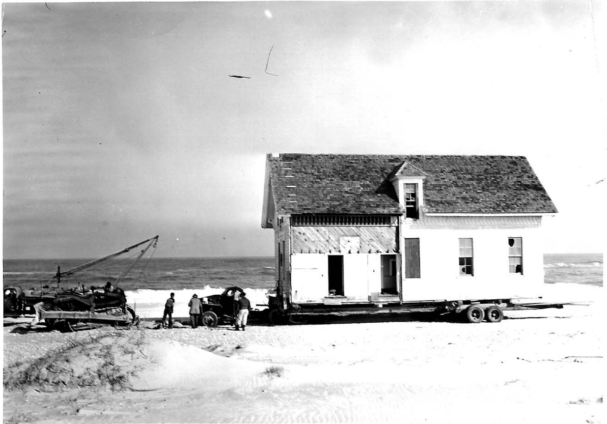
I.18 1879 Station from the east, Jan. 31, 1955. Label – “Neg. No: 55-20, Date: 1/31/55, Print File: St/M, General Description, Location, Other pertinent Data: Supt. Residence being moved. Negative by: A.D.” [Albert Dillahunty]. Shows lean-to removed and evidence of an earlier door location.
