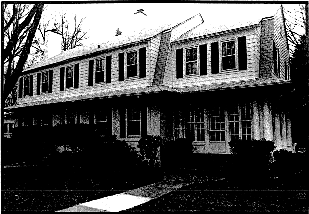
Figure III-154. 1925 Officers housing (Building M-5, Marine Corps Recruit Depot, San Diego, California), above . 1920 Officers housing (Quarters 12, Marine Corps Development and Education Command, Quantico, Virginia), below . (Official U.S. Marine Corps Photograph)
