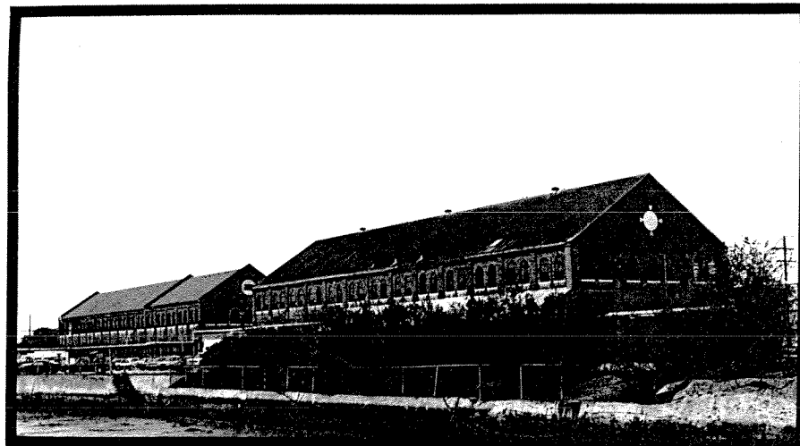
Figure III-57. 1882 Foundry (Building 26, Naval Complex Pensacola, Florida), above . 1882 Machine shop (Building 38, Naval Complex Pensacola, Florida), middle . 1897 Shop buildings (Buildings 10 and 11, Marine Corps Recruit Depot, Parris Island [formerly Port Royal Navy Yard], South Carolina), below .
