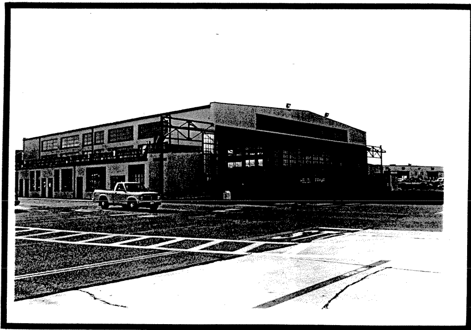
Figure III-166. 1935 Seaplane hangar (Building NS-53, Naval Base Charleston, South Carolina), above. 1930s Land plane hangar (Building 308, Naval Air Station, North Island, California), below.
