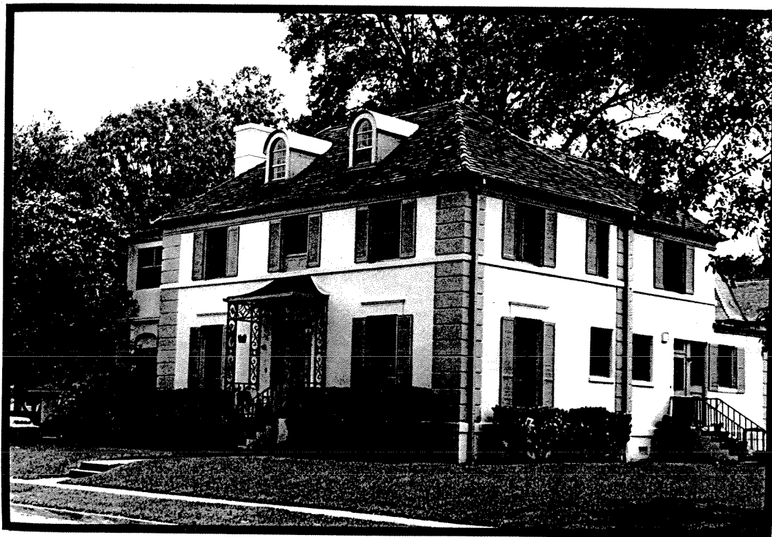
Figure III-140. 1935 Tudor Revival officers housing duplex (Building 318, Wright-Patterson AFB, Ohio), above . French Provincial officers quarters constructed during the early 1930s at Barksdale AFB, below . (Courtesy Louisiana Division of Historic Preservation)
