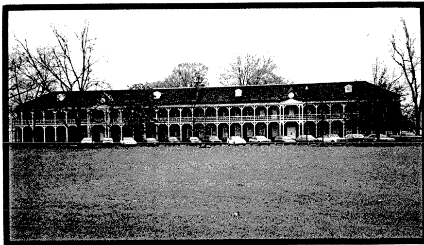
Figure III-109. 1883 Wood-frame barracks (Building 22208, Ft. Huachuca, Arizona), above . 1893 Multiple-company barracks (Building 111, Ft. Bliss, Texas), middle . 1891 Barracks with simplified Queen Anne and Stick style detailing (Building 58, Ft. McPherson, Georgia), below
