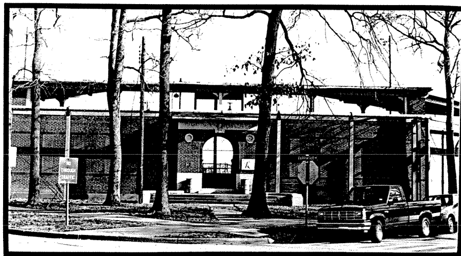
Figure III-83. Doughboy Stadium at Ft. Benning, Georgia, constructed in 1925 under Recreational Center Board, above . Jamestown Tricentennial Exhibition Building, constructed in 1907, converted for use as gymnasium (Building N24, Naval Base Norfolk, Virginia), middle . 1918 Playing field grandstand (Building M050, Naval Base Norfolk, Virginia), below .
