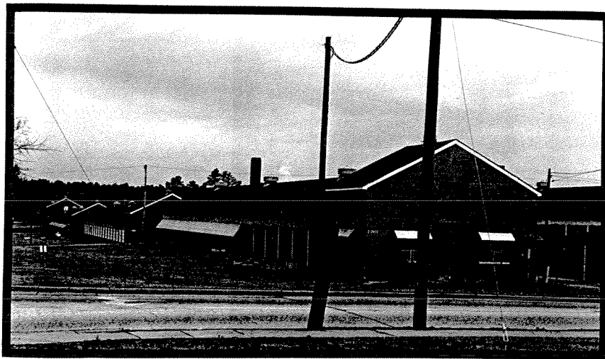
Figure III-174. 1935 Artillery stables (Buildings 22404, 22405, 22205, Ft. Bragg, North Carolina), above . 1935 Stable guard house (Building 22205, Ft. Bragg), middle . 1935 Gun sheds (Buildings 22402 and 22802, Ft. Bragg), below .
