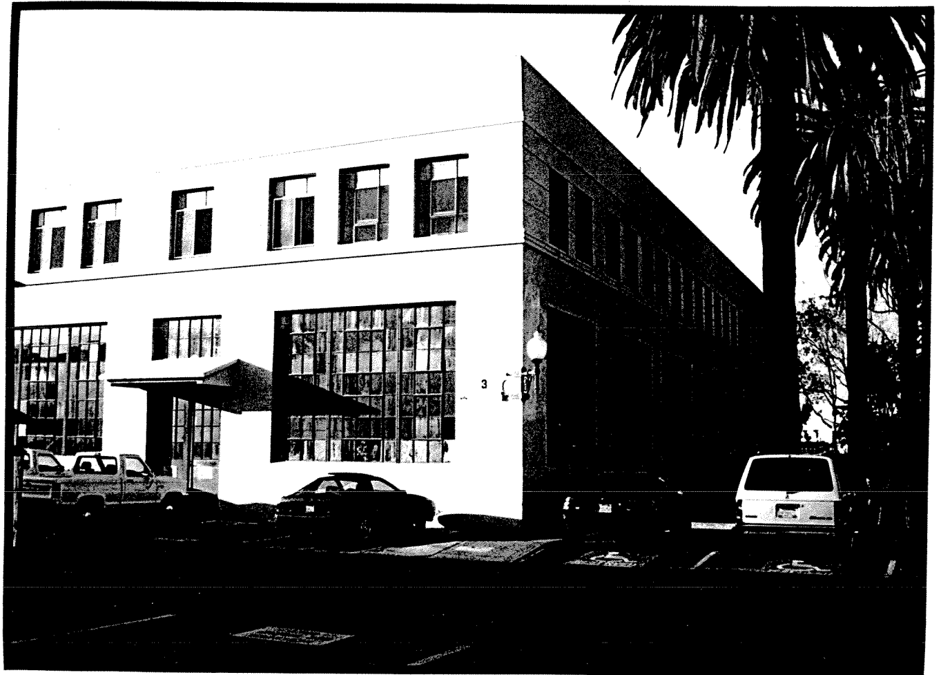
Figure III-52. ca. 1935 Final Engine Overhaul and Assembly Shop (Building 94, Naval Air Station North Island, California), above . 1919 Shops and Tool Room (Building 3, Naval Air Station North Island, California), below .
