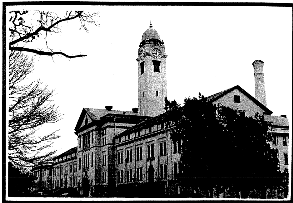
Figure III-24. 1881 Post Headquarters, also served as School of Application for Infantry and Cavalry (Building 44, Ft. Leavenworth). The building originally had a two-story veranda on the east elevation, as well as the existing veranda on the south elevation, above . Grant, Sheridan, Sherman, and Wagner Halls, comprised of two former Ordnance storehouses constructed in 1859 with clock tower added in 1904 (Building 52, Ft. Leavenworth, Kansas), below .
