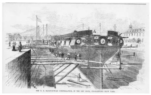
Figure 3.5: Engraving from c. 1859 of Dry Dock 1, which was completed in 1833. Staging installed in the dry dock allowed workers to work on the hull of USS Constellation at two levels from Gleason's Pictorial Drawing-Room Companion (BOSTS 10721).
