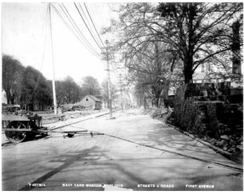
Figure 5.4: Brick paving of First Avenue in 1903 looking east. The sidewalk slabs to the left cover the newly completed Conduit (Structure 280). Note the flagpole and the gun park to the left and the mature trees to the right. Utility lines and poles marked the road (BOSTS-8654).
