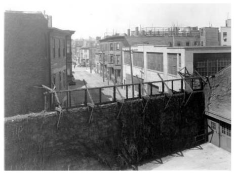
Figure 6.16: Looking west down Henley Street in 1937, showing the Transportation Office (Building 204) outside the wall and the original Building 1 inside the wall, lower right. This section of wall was removed to create Gate 2, and the original Building 1 was replaced by a gatehouse addition to the WPA Garage and Chauffeur's Quarters (new Building 1). Riordan Stables on the left was demolished during World War II (BOSTS-9155).
