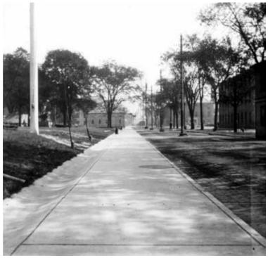
Figure 5.5: First Avenue after paving c. 1903. The concrete sidewalk covers the new Conduit (Structure 280). Note the gutter to the left and the flagpole in the former gun park. Utility poles and lines run down the middle of the avenue, and elm trees still line the south side of the street (BOSTS-8654).
