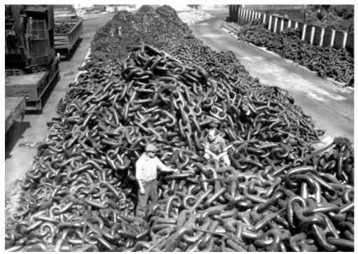
Figure 7.1: Yard-manufactured dielock chain stored in piles, 1943 (BOSTS-9669).
