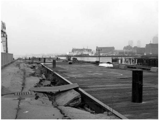
Figure 9.15: This image of Pier 3 shows its deteriorated condition. Pilings are all that remain of the end of Pier 2 (right) (OCLP, 2003).
