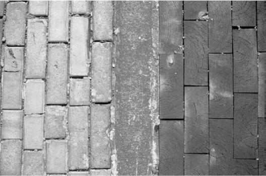
Figure 8.10: Fourth Street paving with yellow bricks on the southern half of the street separated from the wood blocks on the northern half of the street by a strip of granite (OCLP, 2002)
