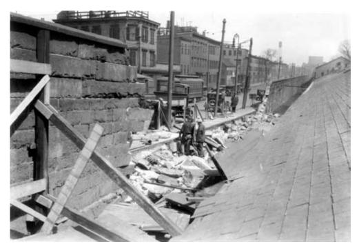
Figure 5.48: Removal of the rubble-filled granite boundary wall between the Ropewalk (Building 58) and Chelsea Street in 1929 (BOSTS-8951).
