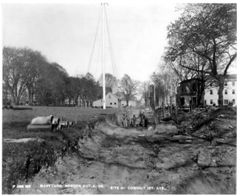
Figure 5.3: Construction of the Conduit (Structure 280) and repaving of First Avenue in 1902. Note the flagpole in the gun park (left center). Trees along the north side of First Avenue have been removed for the project (BOSTS-8654-3).
