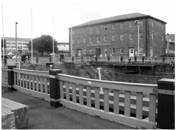
Figures 9.39: Synthetic material is used to create a post-and-pale fence around Dry Dock 1. The pipe-and-chain railing that also surrounds the dock is just inside this fence (OCLP, 2002).
