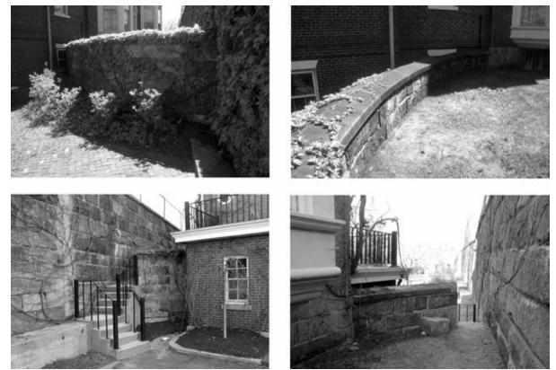
Figure 9.2: The change in grade between the inside (left images) and outside (right images) of the eastern (top images) and western (bottom images) portions of the old boundary wall where it curves toward the former front (north) door of the Commandant's House (Quarters G) forming a semicircle. A staircase negotiates the western portion, bottom left (OCLP, 2002 and 2005).
