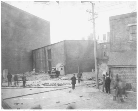
Figure 5.9: Resurfacing Lincoln Avenue and First Street between Hoosac Stores (left) and the Storehouse (Building 4) (right) in 1902 with either Belgian block or brick. An additional Storehouse (Building 3), demolished in 1906, is in the center (BOSTS-9251).
