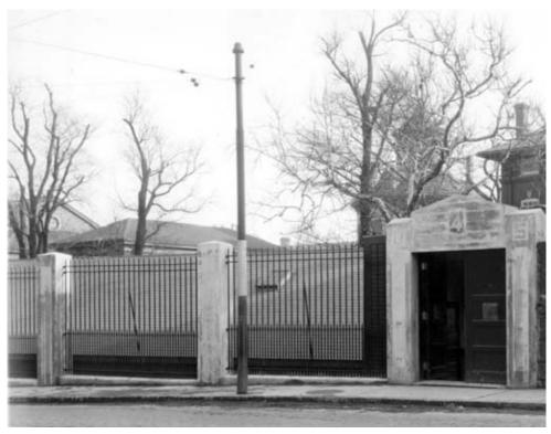
Figure 5.49: Gate 4 after the Navy replaced the granite boundary wall along the Ropewalk (Building 58) with concrete posts and wrought iron fence in 1929 (BOSTS-8951).
