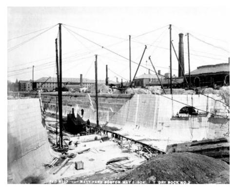
Figure 5.13: Dry Dock 2 under construction in 1904, showing the dramatic transformation of this portion of the yard (BOSTS-8808).
