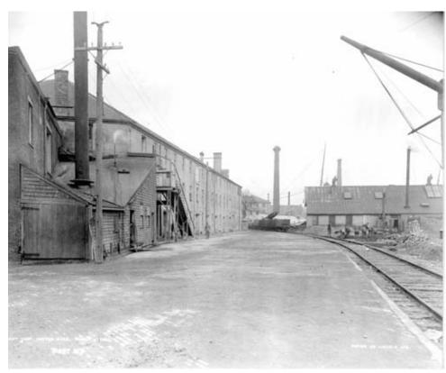
Figures 5.10: Granite Belgian block paving between the Storehouse and Navy Store (Buildings 4 and 5) on the left and the railway in 1903 looking east (BOSTS-9256).
