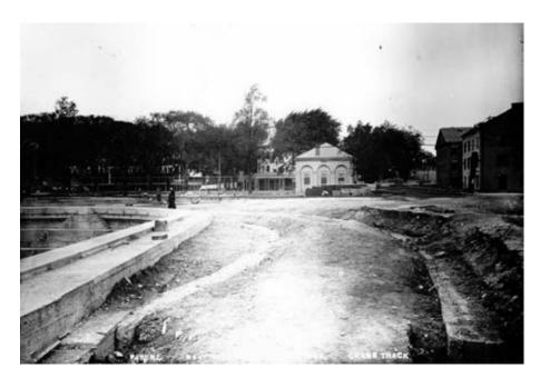
Figure 5.14: Improvements to the yard in 1904 included installing additional crane and rail tracks as seen from the northeast corner of Dry Dock 2. In the distance are the tennis courts, Muster House (Building 31), and Commandant's Office (Building 32), while trees obscure the Marine Barracks (Quarters H-I-K) (BOSTS-8656).
