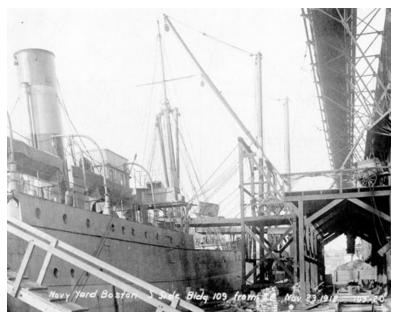
Figure 5.20: 1912 view of the Coaling Plant (Building 109) in operation with a rail line and one of the yard's thirteen dump cars for coal in the foreground (BOSTS-9807,9808).
