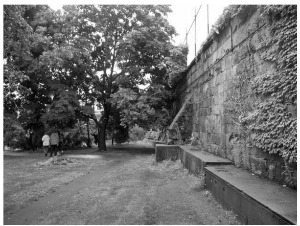
Figure 9.35: The yard's granite block boundary wall northwest of the Commandant's House (Quarters G). The concrete footings were poured during the relocation of the wall in 1981-82 (OCLP, 2003).
