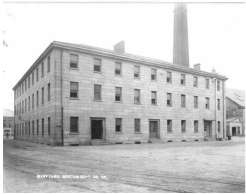
Figure 5.8: Dry Dock Engine House (Building 22) showing granite block paving and rail lines in September 1902 (BOSTS-9288).
