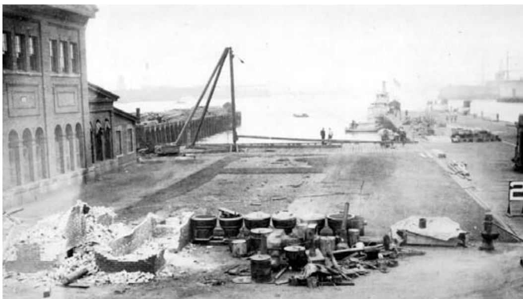
Figure 15: Pier west of Building 125 prior to start of construction on the marine railway. In the foreground are remnants of Building 110, the former Pitch House. Note the two windows to the substation in the west wall the south wing, identifiable by the newly mortared masonry surrounding them. (1918)
