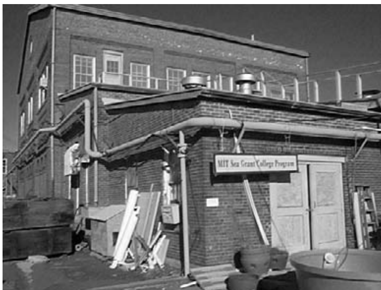
Figure 31: View of the building's southwest corner. The opening now with the pair of doors was constructed for an electrical substation in this location shortly after the building was completed. The two windows in the west wall were added at the same time. (1/15/03)
