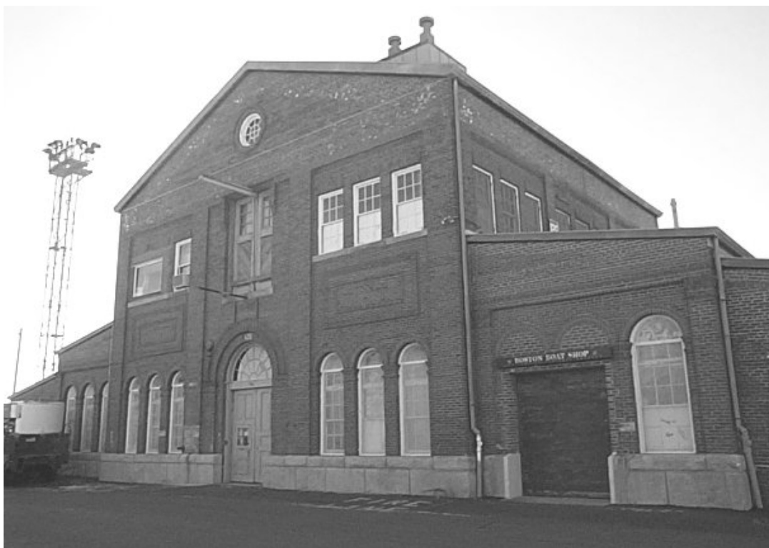
Figure 23: View of east façade. Corbelled brick cornices delineating the pediment and roof eaves were removed in the 1960's. (1/15/03)
