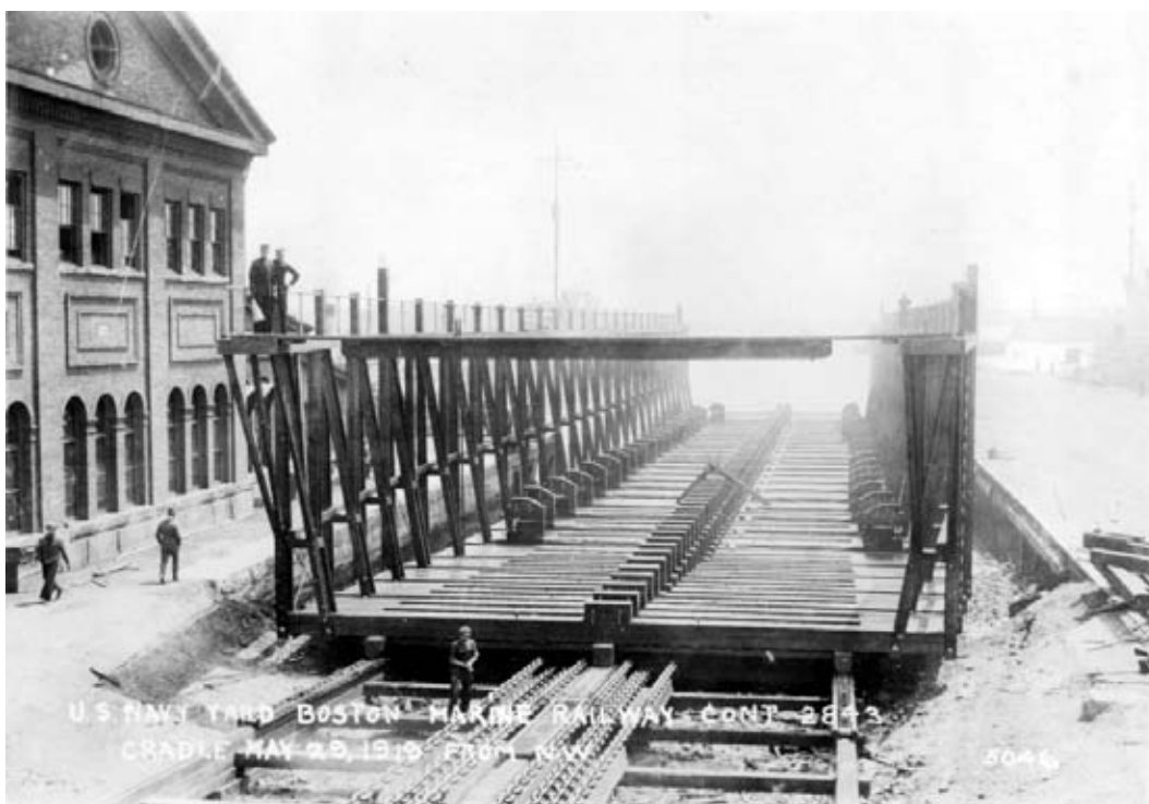
Figure 16: Completed marine railway with its wooden cradle raised (May 1919).
