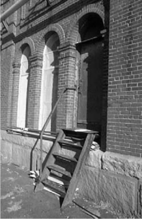
Figure 32: Fire door and stair through an original window opening in the west wall of the main space. (1/15/03)
