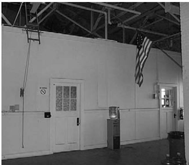
Figure 43: View of second floor corridor. The existing offices were constructed in the 1950's, enclosed by 12' high GWB partitions with suspended ceilings. The corridor is open to the steel trusses of the roof structure above the offices. (1/15/03)
