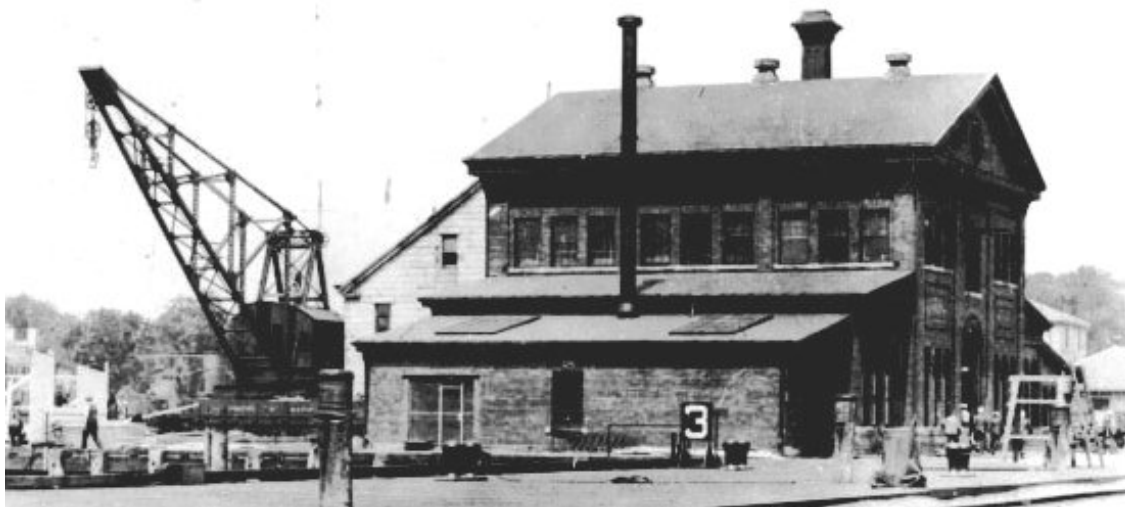
Figure 14: View from the south in an undated photograph taken between spring 1917 (when the north wing was finished) and summer 1918 (when the marine railway construction began). Note the new substation door in the west side of the south wall. The opening at the center of this wall is the original wood window, which exists today.
