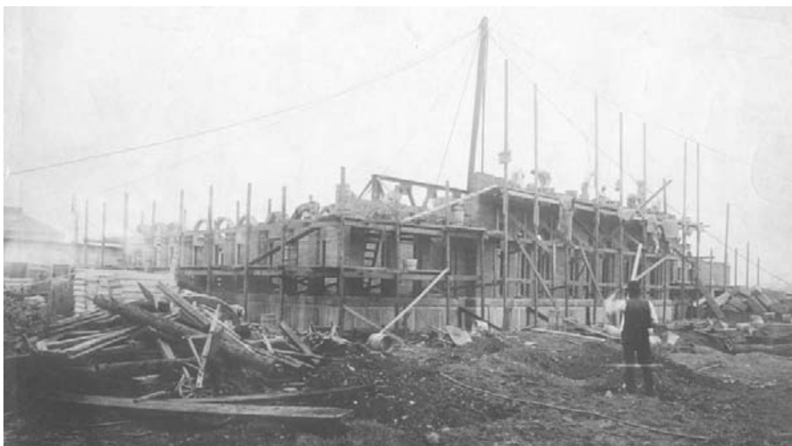
Figure 8: View from the northwest of walls rising (September 1905). One of the two steel warren trusses that will support the second floor is visible above the walls. This is the last construction progress photograph in the NPS archives, though undoubtedly regular photographs documenting the work were made.
