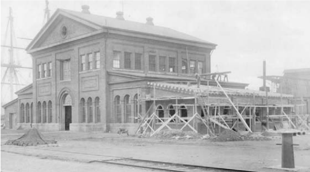
Figure 12: North wing extension under construction (December 1916). Note the wood rafters. The original building's roofs were all constructed of concrete on steel rafters.
