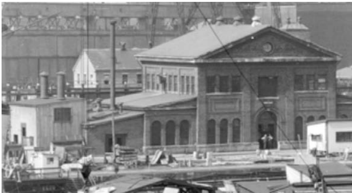
Figure 17: Temporary shed attached to south wing (Sept. 1939). The new elevator penthouse is visible on the north side of the main roof.
