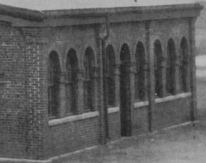
Figure 27: This ca. 1917 photograph of the north wall shows the original exterior single door opening within a typical brick arch.
