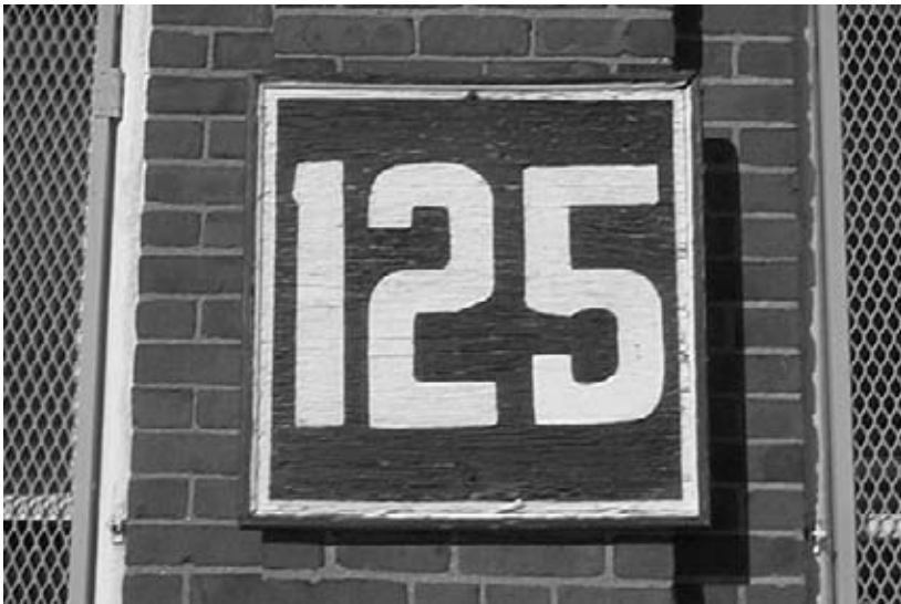
Figure 34: Building number sign. Two (probably original) signs are on the building, attached to the north and south facades. (1/15/03)
