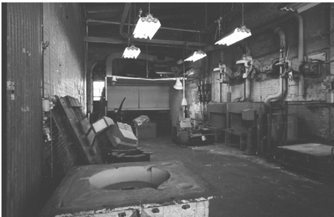
Figure 37: View of Room 103 from east, as abandoned by the Navy. Note the paint mixers along the north wall that remain in the same location today. They could be preserved as an exhibit of primary paint shop equipment. (1/15/03)
