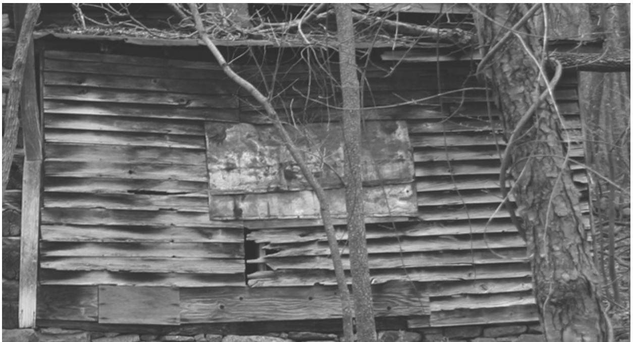
FIGURE 55. View of exterior of enclosed porch, showing two generations of siding. (NPS, 2005)
