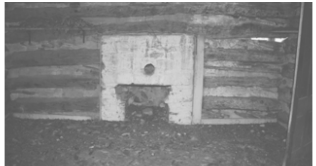
FIGURE 42. View of north wall of Room 100. (NPS, 2005)
