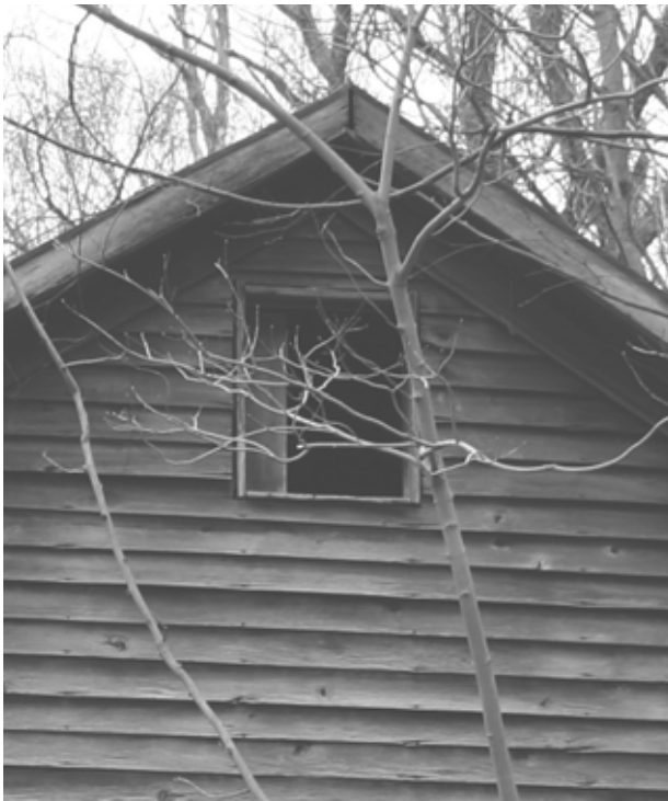
FIGURE 35. View of east gable. (NPS, 2005)
