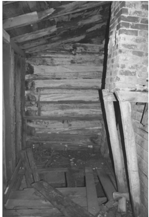
FIGURE 56. View west in Room 102. (NPS, 2005)
