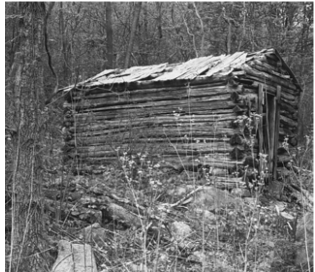
FIGURE 16. View northeast of chicken house in 1977. (NPS, BLRI Coll.)
