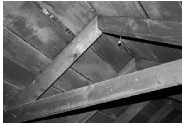
FIGURE 32. View of typical rafters and collar beam. (NPS, 2005)
