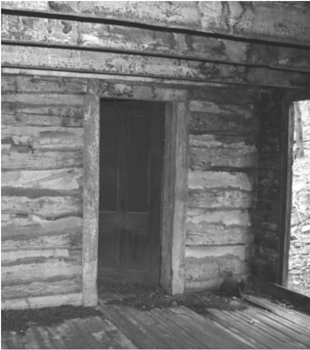
FIGURE 53. View of west wall of Kitchen. (NPS, 2005)
