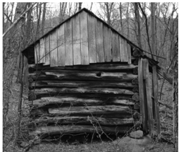
FIGURE 60. View of south end of meat house. (NPS, 2005)
