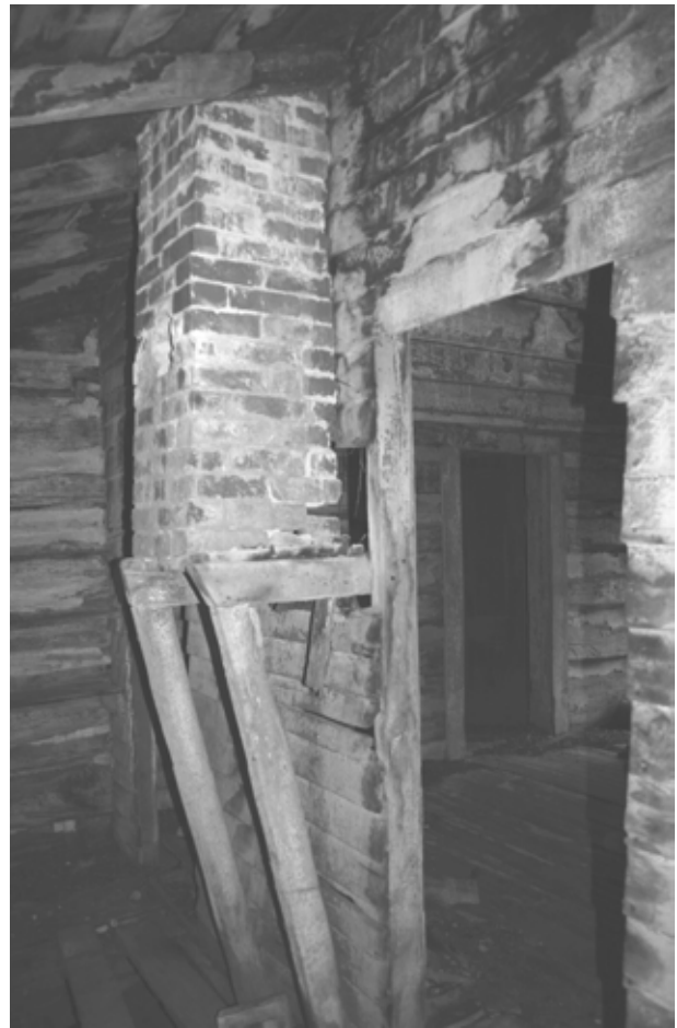
FIGURE 27. View of kitchen chimney. (NPS, 2005)
