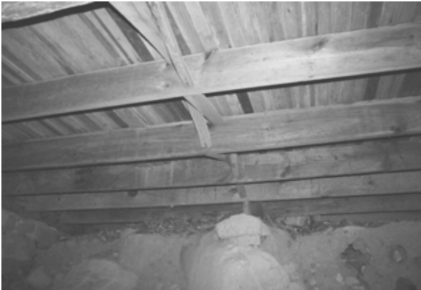
FIGURE 30. View of floor framing in log pen. (NPS, 2005)
