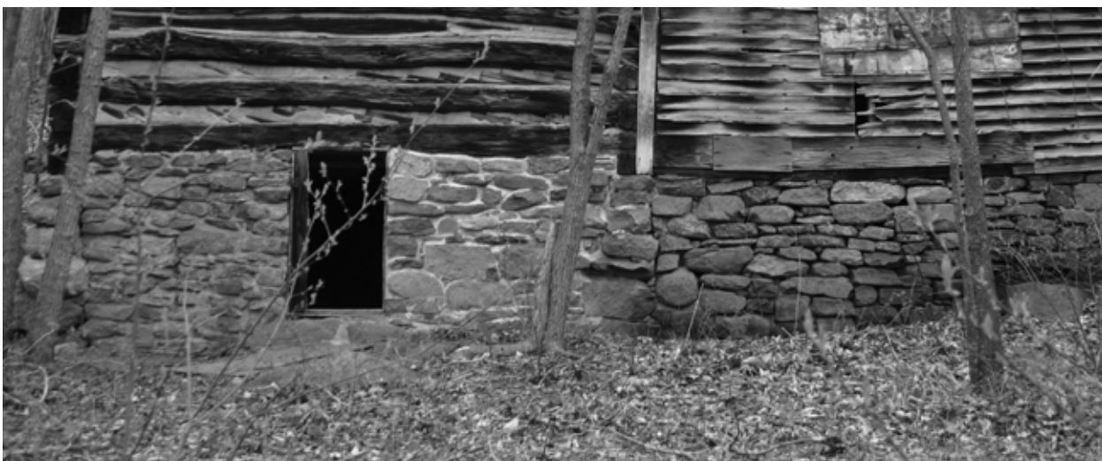
FIGURE 22. View of foundation at south end of house, showing cellar doorway.
