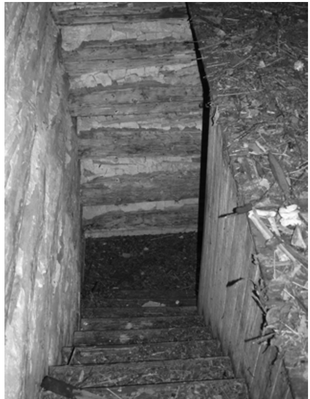
FIGURE 46. View of stairway from Room 200 to Room 100. (NPS, 2005)
