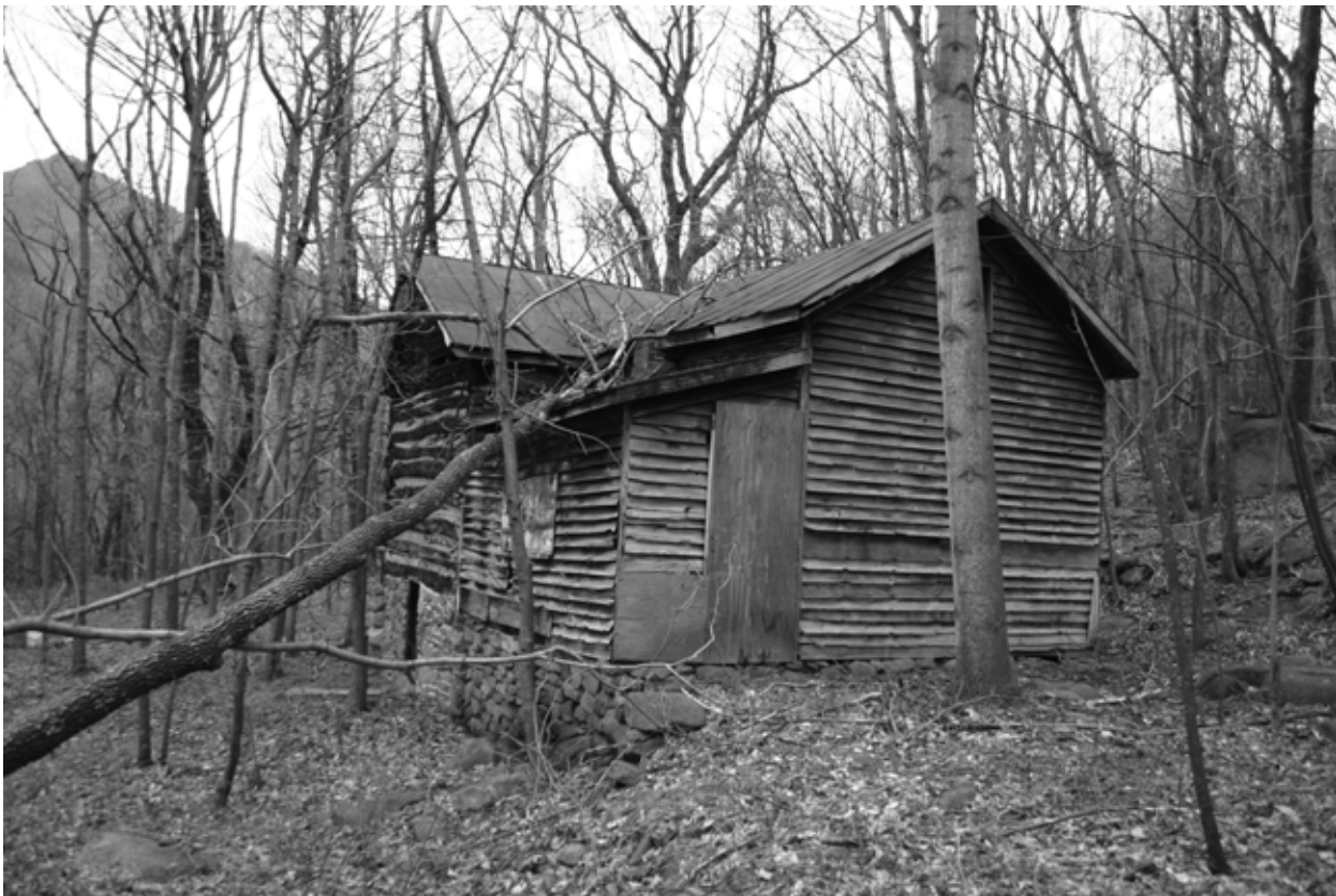
FIGURE 40. View west-northwest of rear and south sides. (NPS, 2005)
