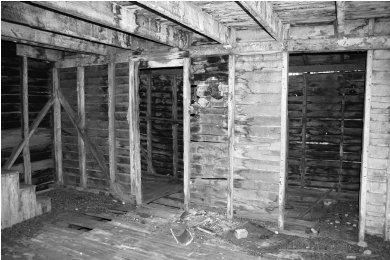
FIGURE 54. View southeast in Room 101. (NPS, 2005)
