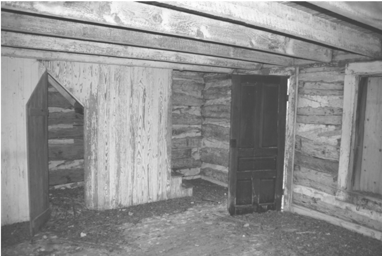
FIGURE 45. View to southwest in Room 100. (NPS, 2005)
