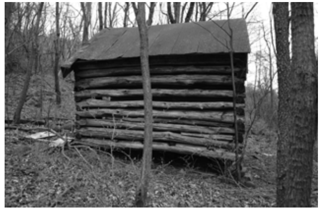
FIGURE 58. View of west side of meat house. (NPS, 2005)
