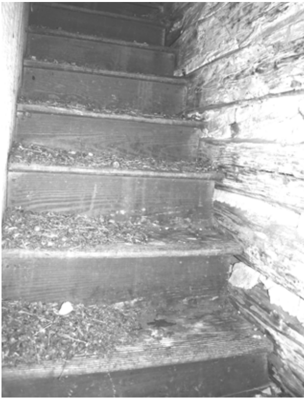
FIGURE 44. View of stairs to second floor of log pen. (NPS, 2005)
