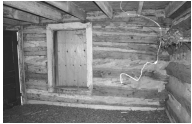
FIGURE 41. View west in Room 100. (NPS, 2005)
