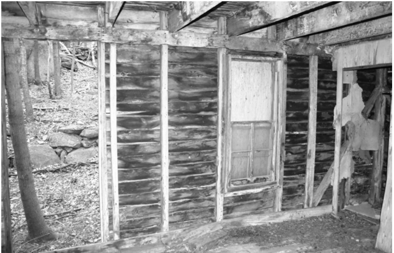
FIGURE 51. View northeast in Kitchen. (NPS, 2005)
