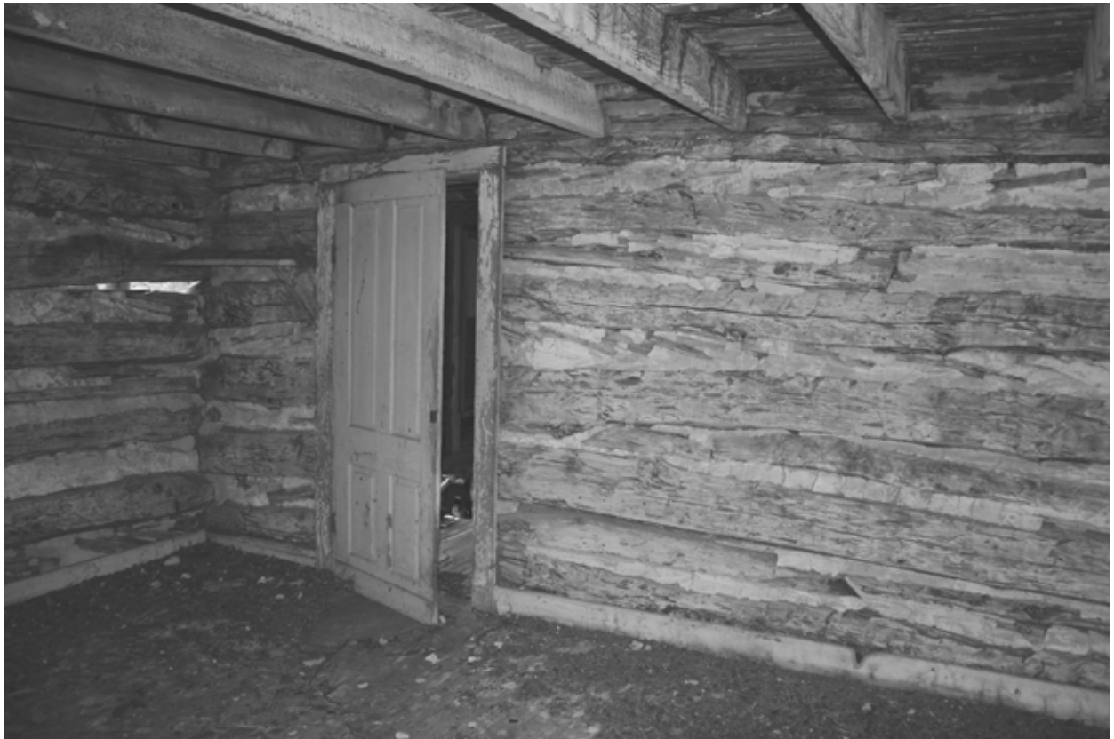
FIGURE 43. View northeast in Room 100. (NPS, 2005)
