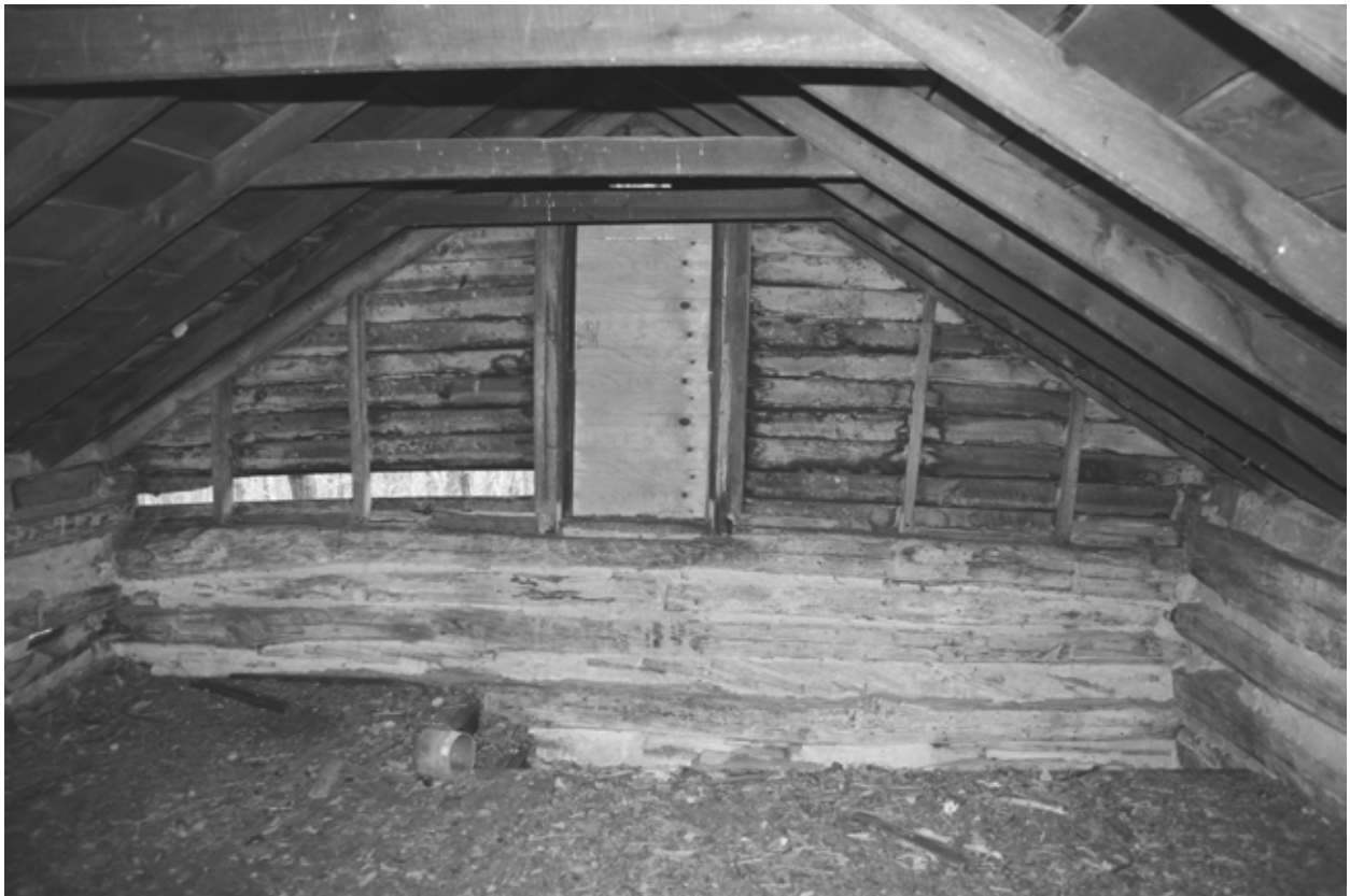
FIGURE 47. View south on second floor of log pen. (NPS, 2005)
