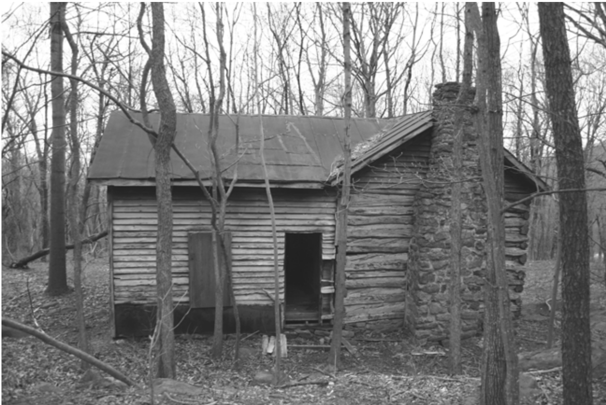
FIGURE 36. View of north side of house. (NPS, 2005)
