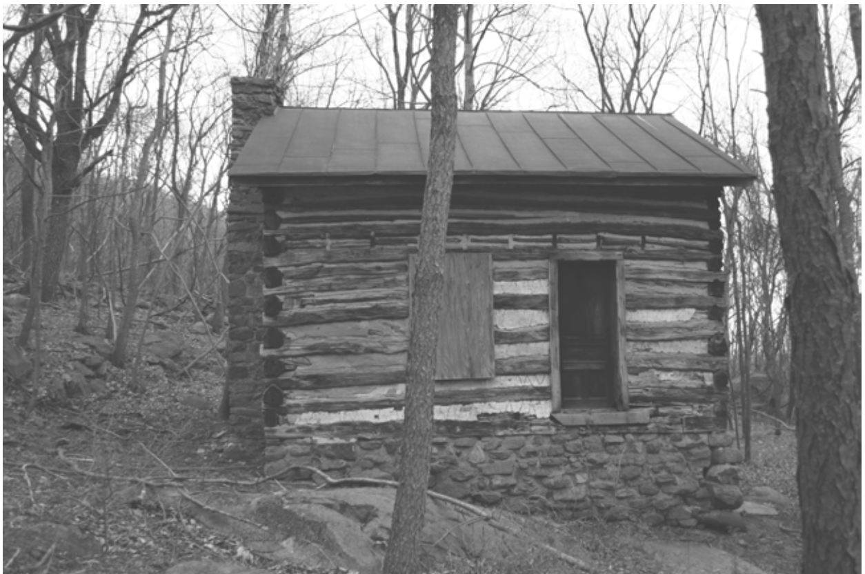
FIGURE 37. View of front of house. (NPS, 2005)
