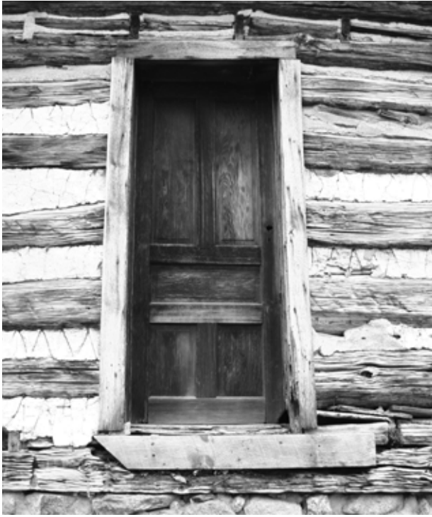
FIGURE 39. View of front door. (NPS, 2005)
