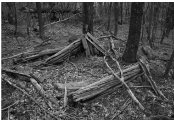
FIGURE 63. View southeast of ruins of hog house. (NPS, 2005)
