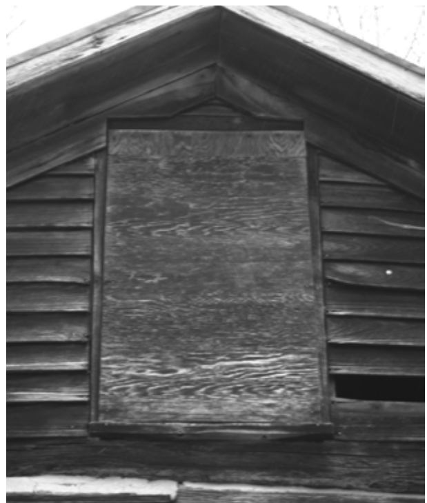
FIGURE 38. View of window in south gable. (NPS, 2005)
