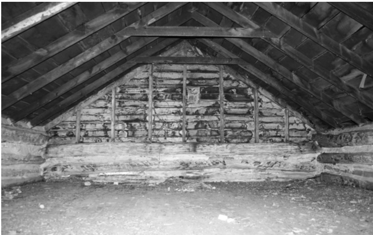
FIGURE 50. View south in Room 200. (NPS, 2005)
