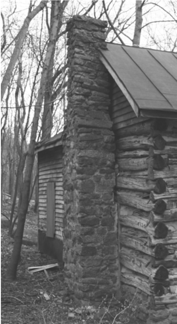
FIGURE 25. View of chimney. (NPS, 2005)
