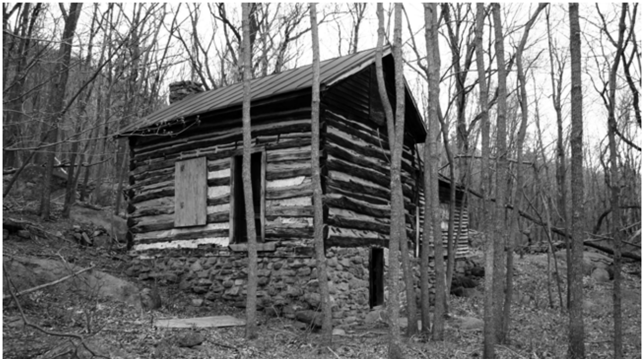
FIGURE 19. View to northeast of Saunders House. (NPS, 2004)
