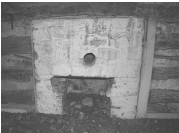
FIGURE 26. View of fireplace. (NPS, 2005)
