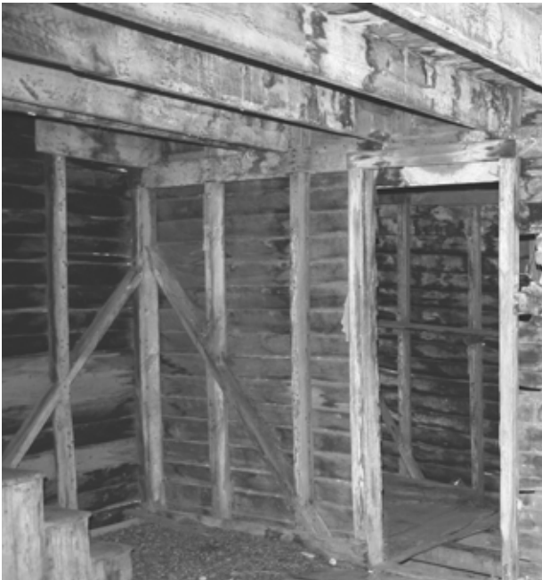
FIGURE 31. View of framing at southeast corner of the kitchen. (NPS, 2005)
