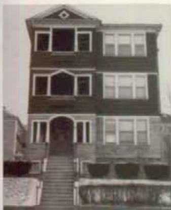
With sensitive maintenance, mill housing will remain a strong part of our identity.
