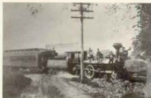
The Providence & Worcester Railroad is the oldest American railroad in continuous ownership and operation. Its opening in 1847 greatly expanded the markets for Valley textiles.
