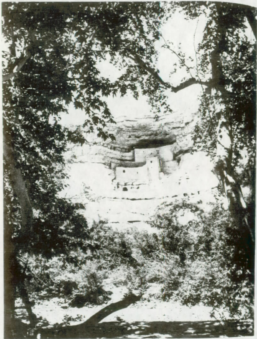
Montezuma Castle National Monument, Camp Verde, Arizona. The structure was built and occupied during the period A.D. 1100-1400 by a people of Puebloan ancestry. Only a few breaks in the upper parapet wall and the roof of the square tower room have been repaired with original materials. By 1957, increasingly heavy visitor impact began to weaken the structure noticeably, at which time it was closed to public viewing. The ruin is seen today by visitors from the trail below where a cutaway scale model enhances the interpretive story.
