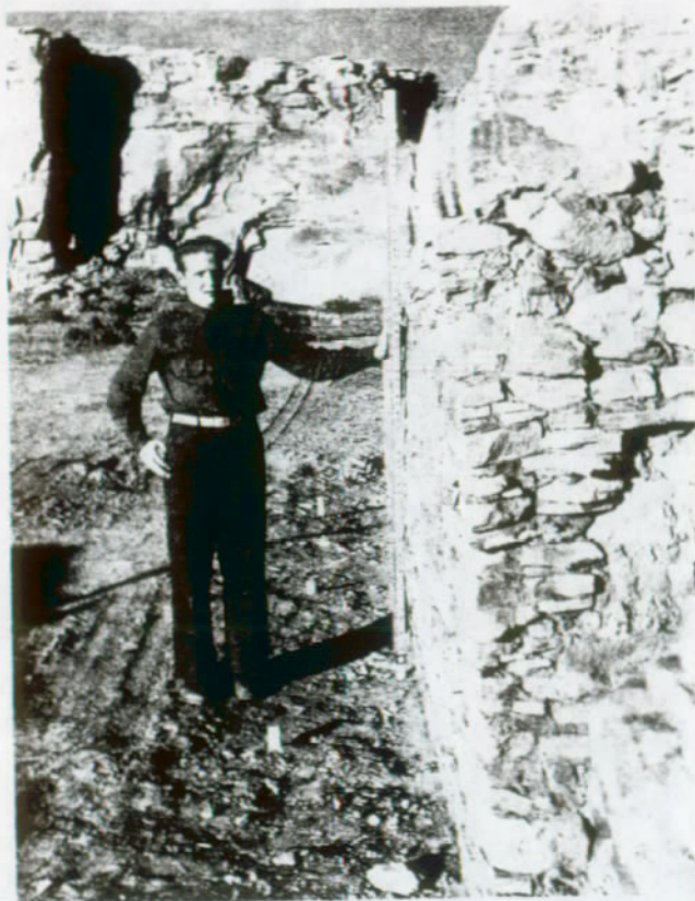
FIGURE 35. The wall depicted in figures 33 and 34 after pressure had been applied for three weeks by means of jacks in sleeves.
