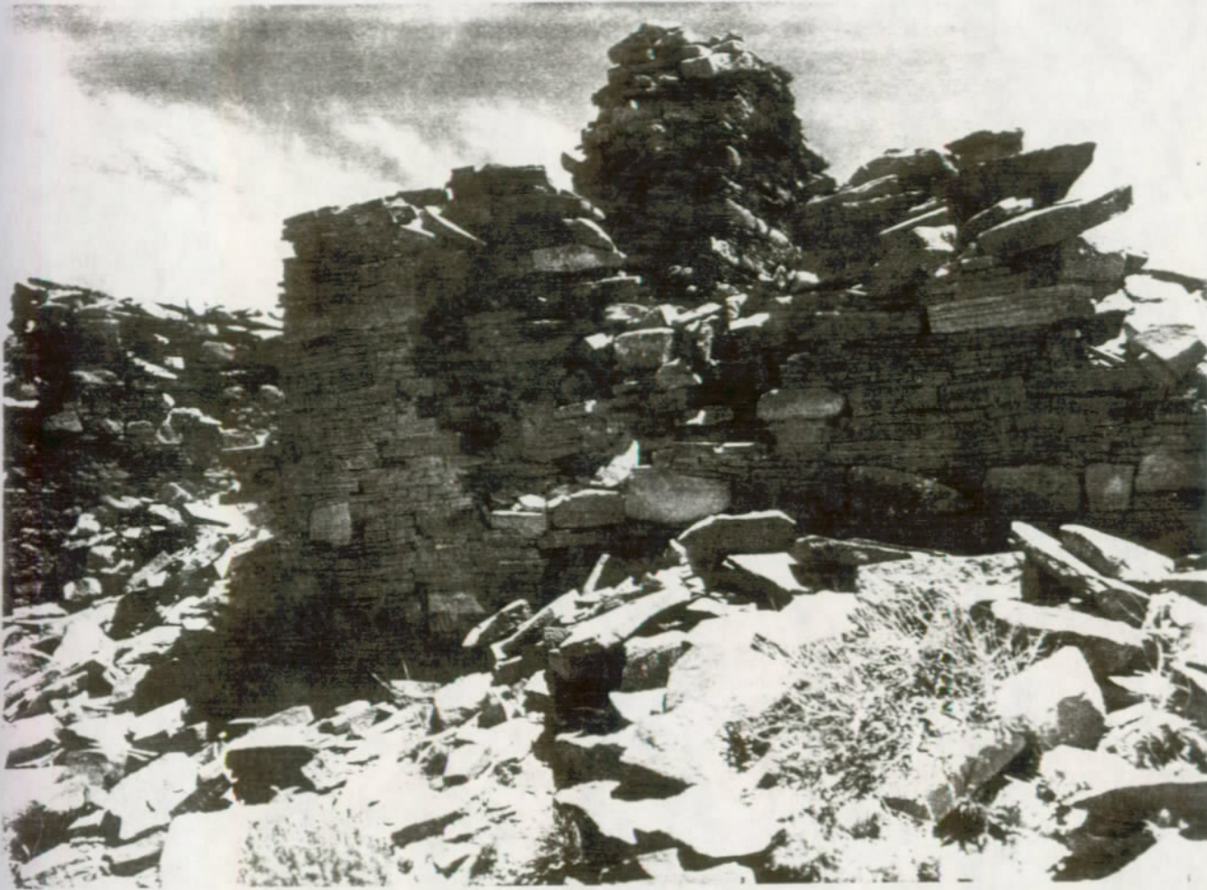
FIGURE 23. An example of soft, pecked and dimpled stone in random areas over wall surface. Replacement of the stone requires extreme care if the character of the wall is not to be changed. (Peñasco Blanco Ruin, Pecos Canyon National Monument, N. M.)
