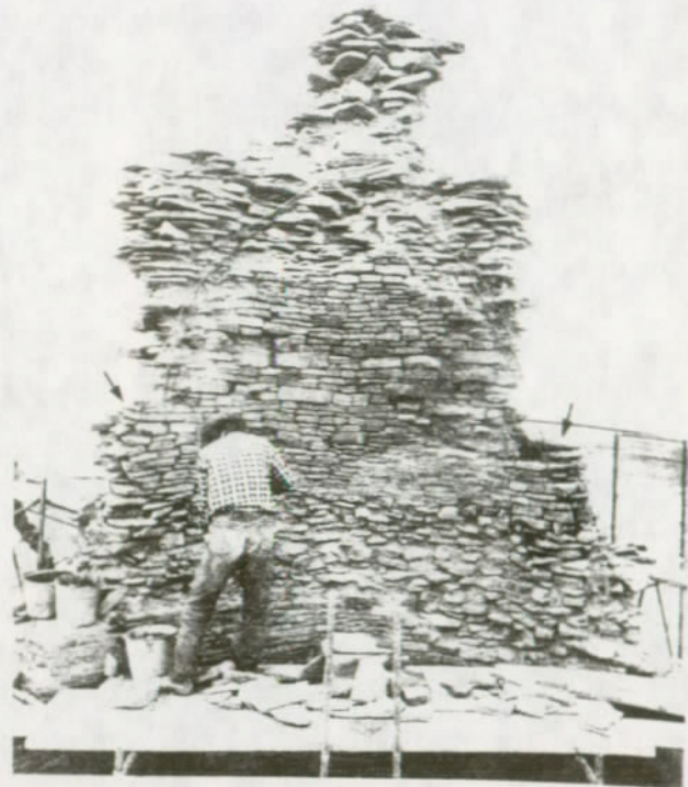
FIGURE 109. Beginning the vertical, reinforced capping (arrows).
