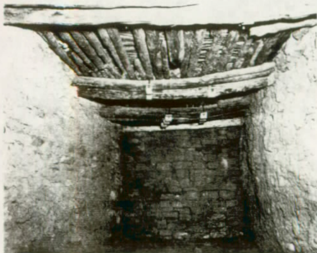
FIGURE 48. The ceiling shown in figure 47 after removal of the overburden and construction of a slab roof which protected the ceiling and permitted support of broken beams. The bolts are fastened in the slab above, and were taken up enough to transfer most of the weight from the old ceiling beams to the new roof.
