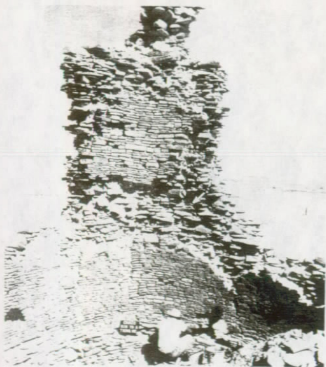
FIGURE 103. General view of northeast interior of Tower Kiva at start of project. The circular wall is stepped back or inset at two points: (1) at narrow ledge or bench where workman is beginning repairs, and (2) where facing is gone, exposing core (arrow).
