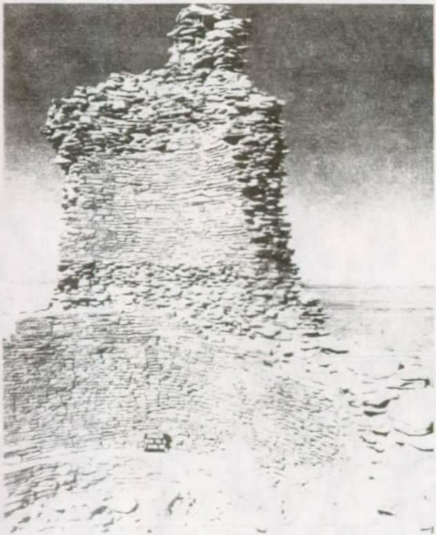
FIGURE 111 The wall at completion of stabilization. The wall is considerably strengthened and tightened, without a serious or objectionable alteration of the original profile.
