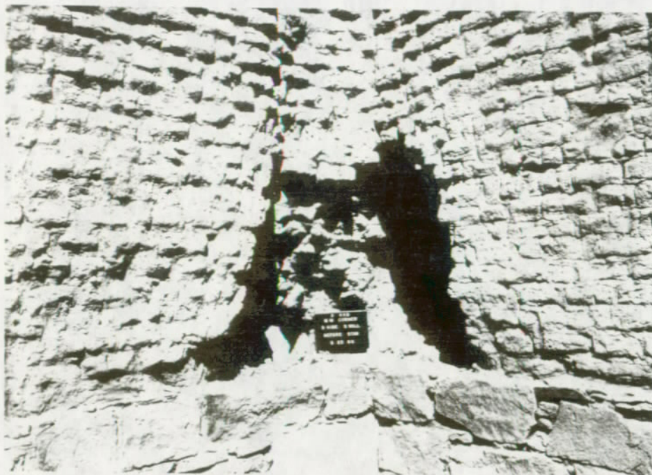
FIGURE 75. Building 3-440, southwest corner, before stabilization. Fort Union National Monument.
