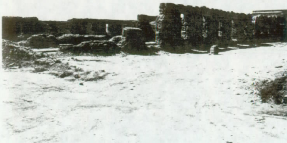
FIGURE 74. Building 3-440, from the northeast, after stabilization. Fort Union National Monument.
