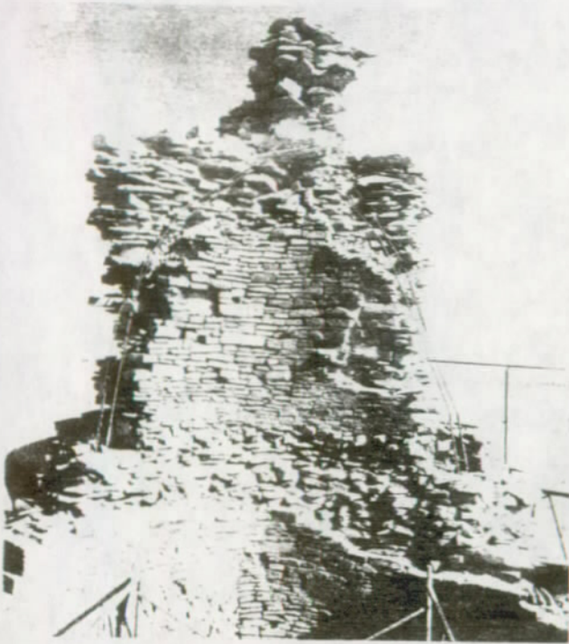
FIGURE 108. Upper portion of Tower Kiva, northeast corner interior, after the integral members were anchored in masonry.
