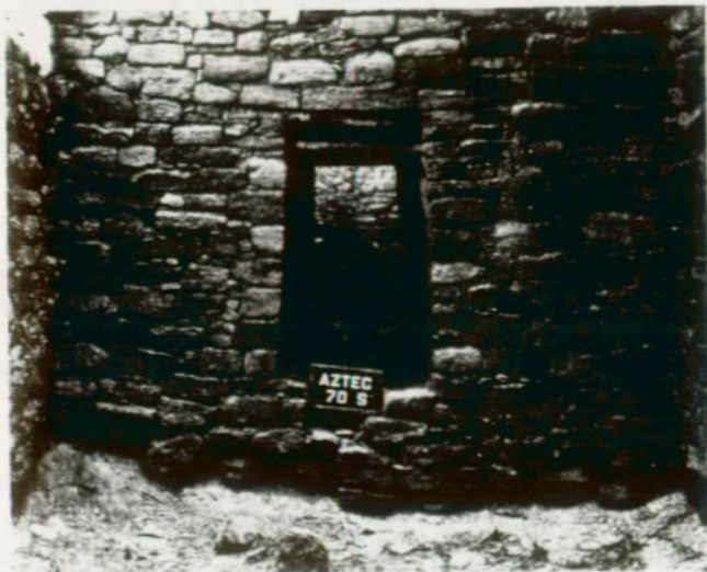
FIGURE 17. Basal erosion from capillary moisture is particularly damaging in the interiors of excavated sites where drainage is poor. (West Ruin, Aztec Ruins National Monument, Ariz.)
