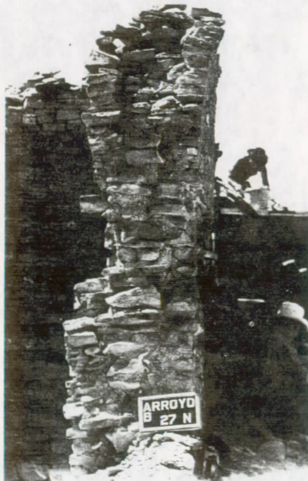
FIGURE 2. Aboriginal construction often left narrow strips at ceiling line. This wall is much wider at the top than in the center. (Room 27, north wall, Pueblo del Arroyo Ruin, Chaco Canyon National Monument, N. M.)
