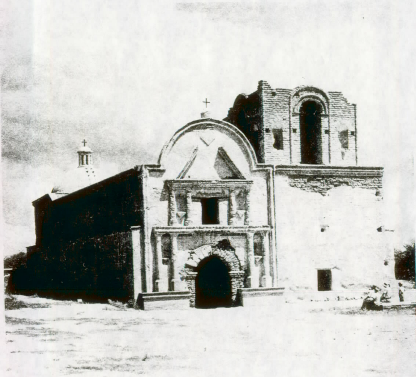
The Mission Church, Tumacacori National Monument, Tumacacori, Arizona. Comprehensive stabilization, repair, and partial restoration of the Mission Church was performed in 1921 by Frank Pinkley. Lower portions of the columns and bases of the facade were restored in 1945. Since that time, all efforts by the National Park Service have been directed to preserving existing original construction. Replacement plaster, where required to cover eroded original lime plaster and adobe brick surfaces, consists of a tinted cement-lime-sand mortar employed with a bonding agent.
