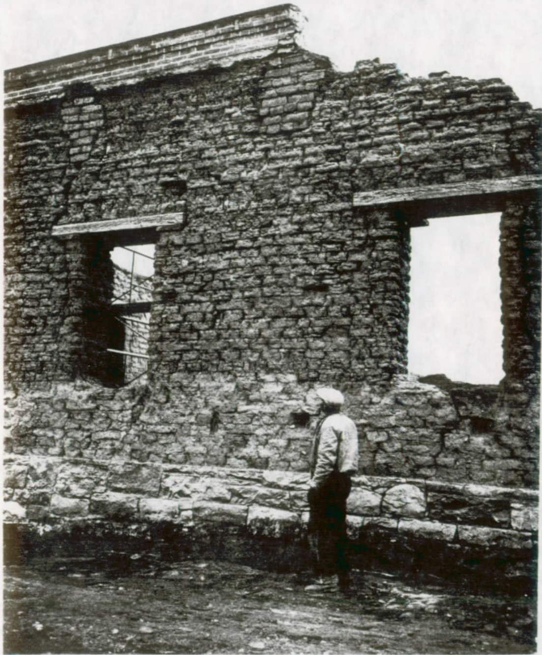
FIGURE 69. Building 3-440, west wall and coping, during stabilization. Fort Union National Monument.
