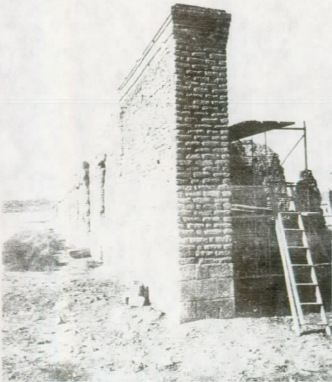
↖ BUILDING 3-330, ROOM 331, WING WALL, AFTER STABILIZATION
