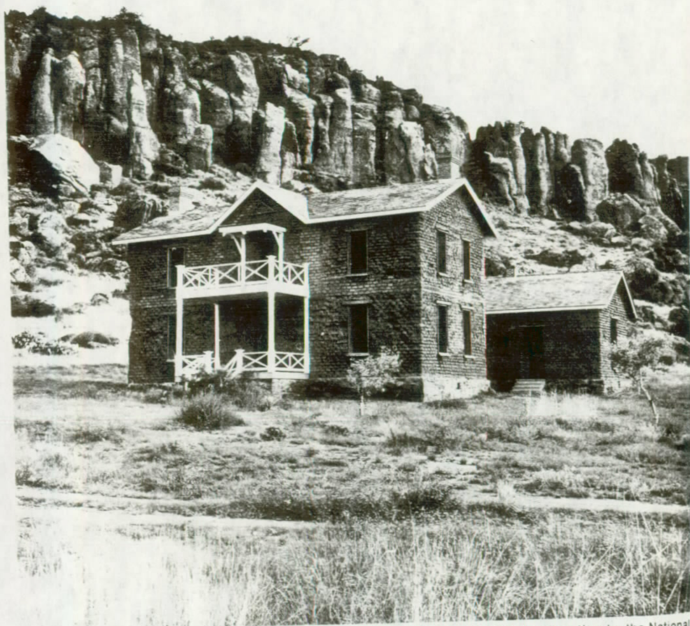
FIGURE 59. Building HB-15 and its outbuilding, a kitchen, following modified restoration by the National Park Service. Soil-cement adobes simulating original adobes were used as modular units of repair. Compare with figure 58.
