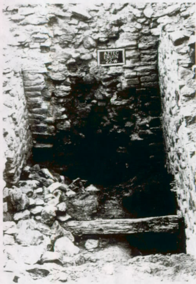
FIGURE 24. Wall break in a partially excavated site. A patch must be designed to prevent further flow of water and fill at the top, and some excavation will be required to base patch on sound masonry. (East Ruin, Aztec Ruins National Monument, N. M.)
