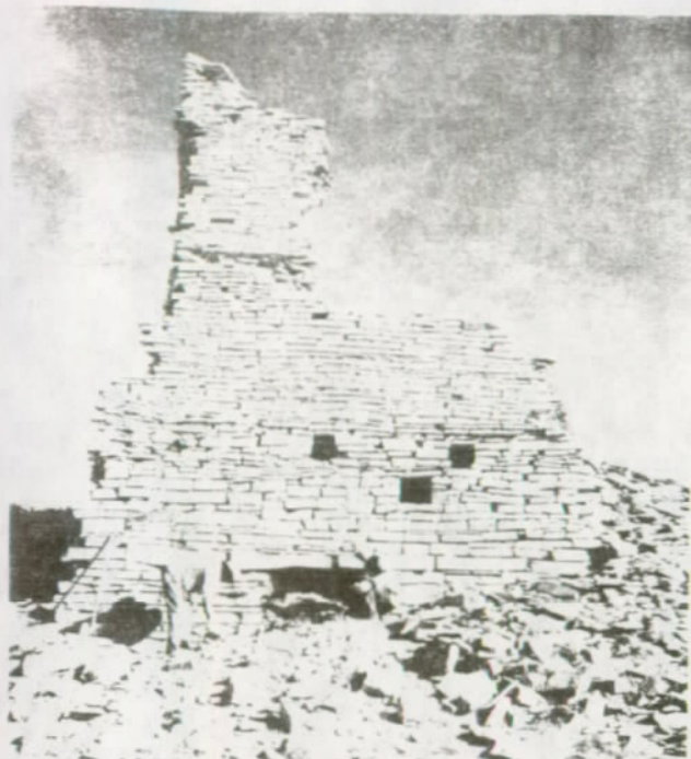
FIGURE 100. Close-up of north wall, Tower Kiva.
