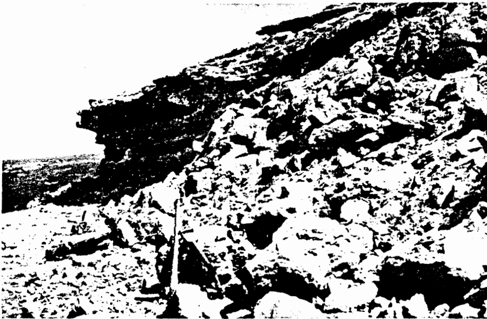
Fig. 3.31. (A) Drilling the rock overburden in University Quarry prior to blasting in 1908, looking north. A 2-horse team and scraper similar to the one shown here were used in all quarries to remove rock after blasting. When the scraper approached the bone bed, the men turned to hand tools to avoid damage to the bones; (B) Rock rubble resulting from blasting in University Quarry in July 1908.
