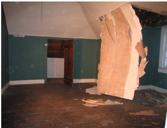
Figure C-56 Room 203, looking southeast
