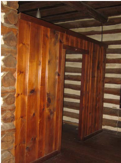
Figure C-35 Added paneled wall in Room 102
