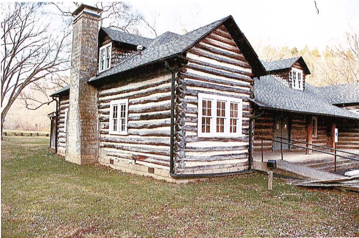
Figure 3 The log walls rest on a cast-in-place concrete perimeter wall with two eight inch courses of block.
