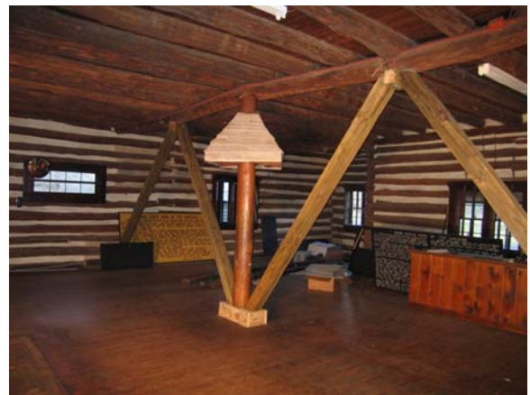
Figure C-33 Room 102, looking northeast
