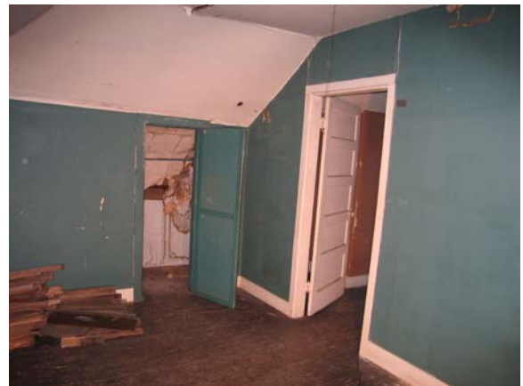
Figure C-57 Room 203, looking northwest
