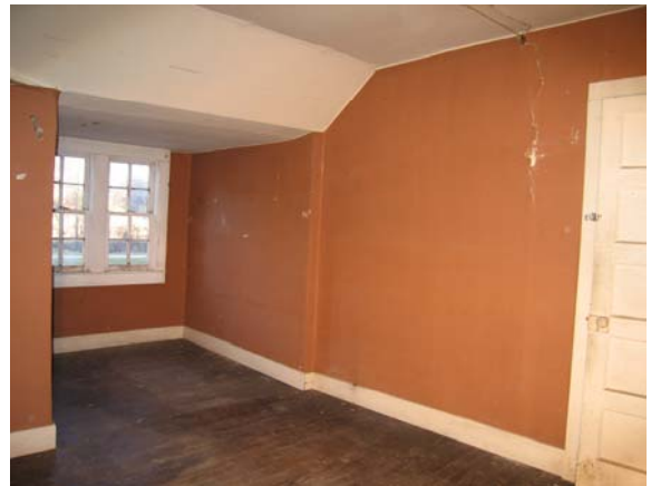
Figure C-60 Room 204, looking southeast
