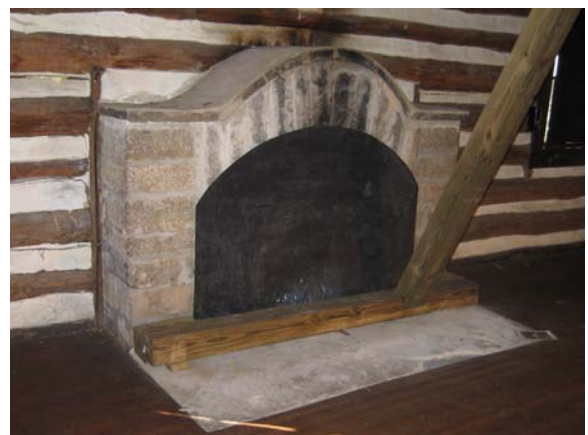
Figure C-39 Fireplace in Room 102
