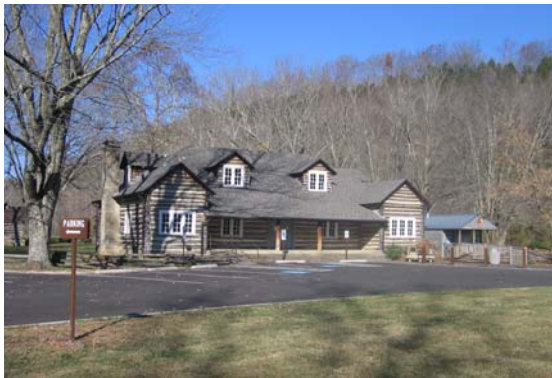
Figure C-1 Tavern from the southeast
