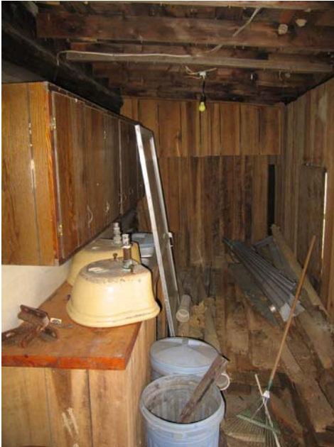
Figure C-48 Room 105 looking south
