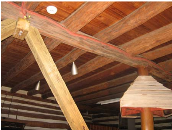
Figure C-9 Log joists, beams, and posts, with modern temporary supports
