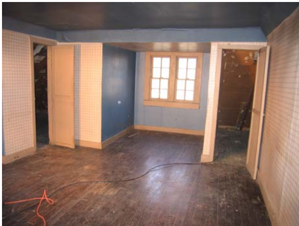
Figure C-63 Room 205, looking northwest
