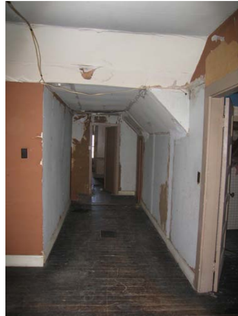
Figure C-53 Room 202, looking west
