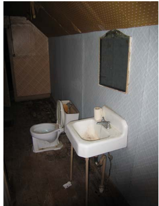
Figure C-51 Room 201, looking southeast
