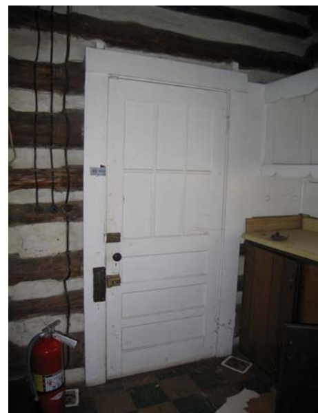
Figure C-16 Original rear doorway in kitchen
