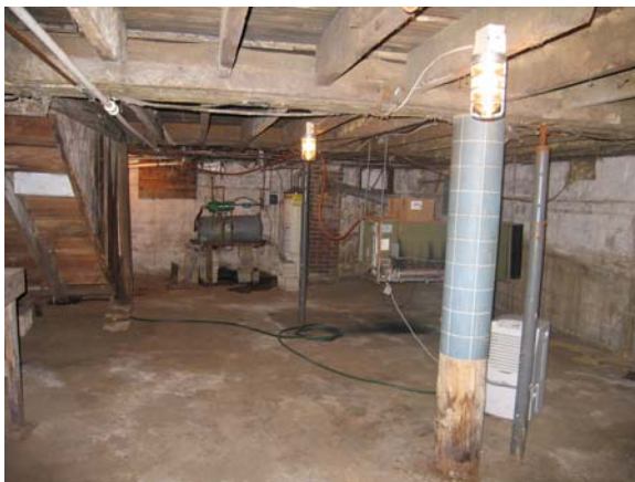
Figure C-23 Room 001, looking northwest
