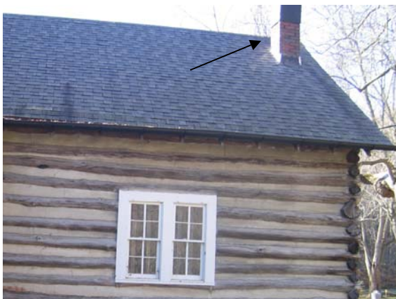
Figure C-12 Brick chimney at kitchen
