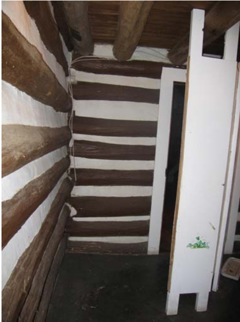
Figure C-46 Room 104 looking east
