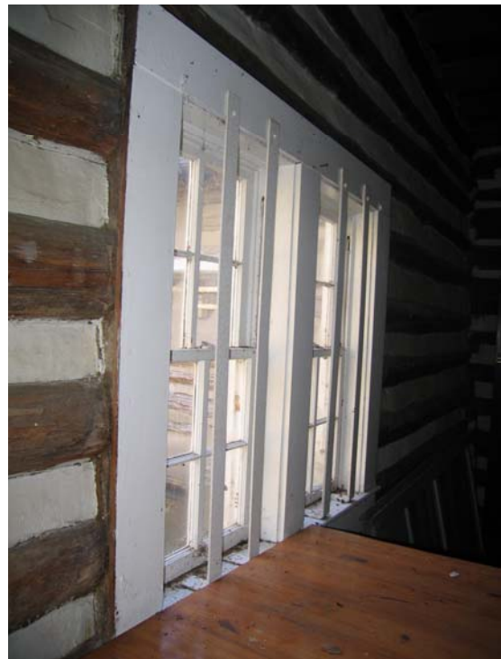
Figure C-29 Window on north wall of kitchen
