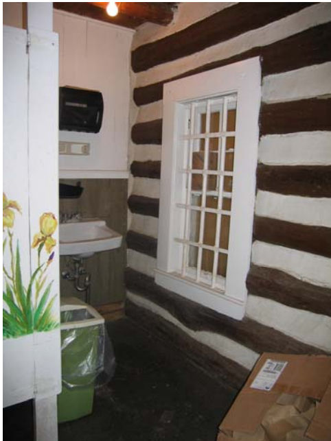
Figure C-45 Room 104, looking southwest
