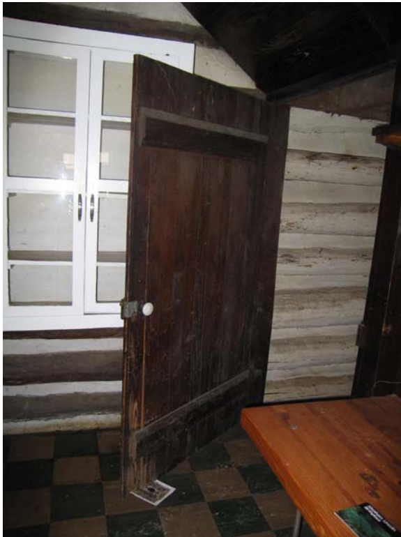
Figure C-28 Door to basement, with original box lock
