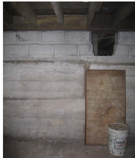
Figure C-4 Basement interior showing cast-in-place concrete and concrete masonry units
