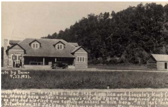
Figure B-1 Cabin and tavern looking west, September 23, 1933 (photo by Beuer)
