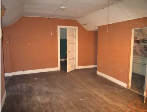
Figure C-59 Room 204, looking southwest
