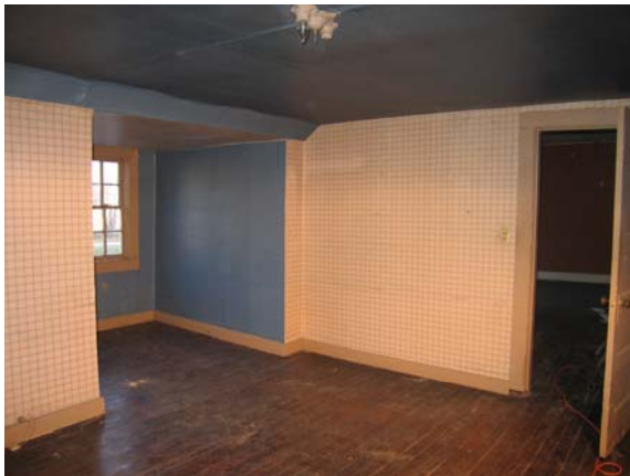
Figure C-64 Room 203, looking southeast
