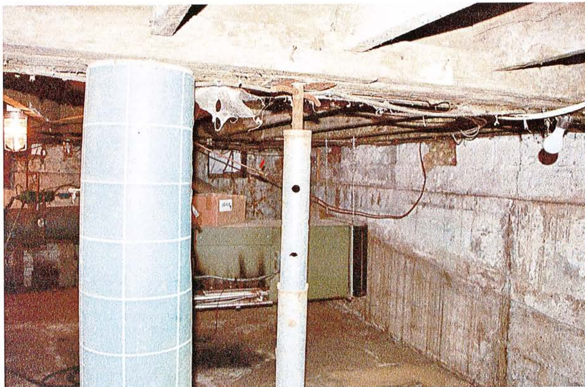
Figure 8 The screw jack was added to supplement the original support.
