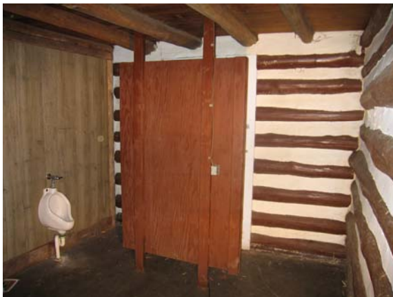
Figure C-43 Room 103, looking northeast
