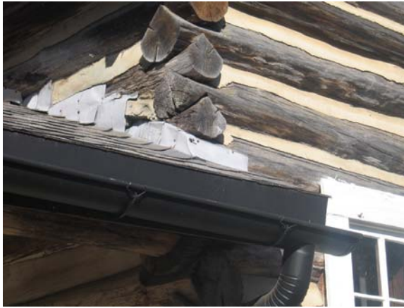
Figure C-11 Composition shingle roofing and galvanized steel gutters and downspouts
