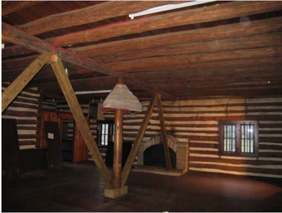
Figure B-6 View of added bracing inside hall, 2005
