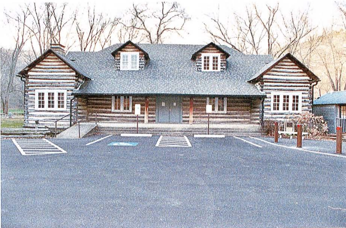
Figure 1 The Tavern is a story and a half log structure with two dormers and two gable endwalls facing the road.
