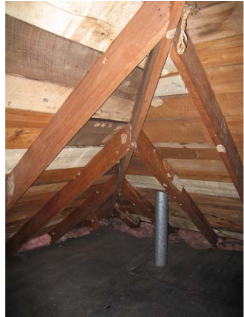
Figure C-10 Rafters and sheathing visible in attic
