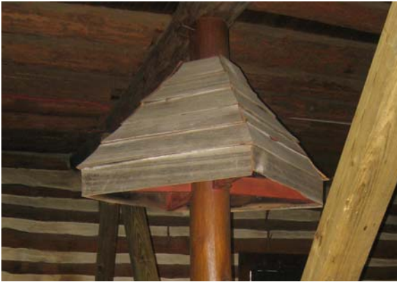
Figure C-40 Display canopy in Room 102
