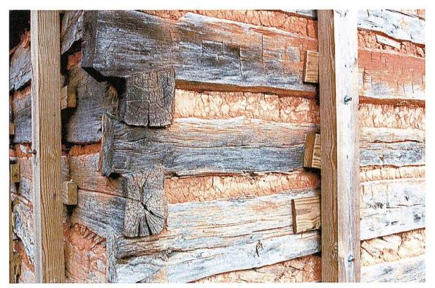
Figure 2 The cabin is constructed using chamfer and notch method.
