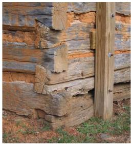
Figure C-2 Half dovetail (chamfer-and-notch) corner
