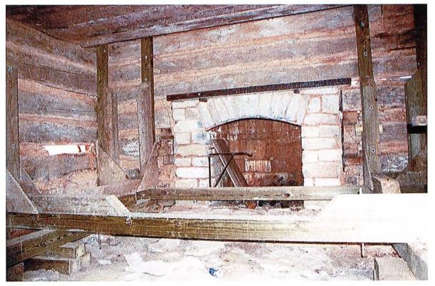
Figure 6 The stone fireplace appears to have been constructed at a later time.
