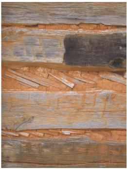
Figure C-5 Detail of logs and chinking
