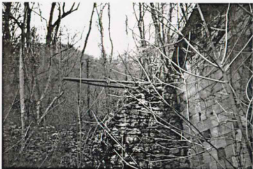
Figure 27 Powerhouse Existing Condition Photo: Structural detail. View from interior of boiler room. Notice lack of roof, missing sections of back wall, and vegetation growing inside the building. Nov. 1996. NPS photo.
