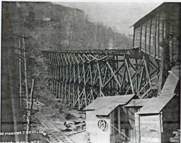
Figure 12 The monitor trestle supported the tracks that ran 1,000 feet from the headhouse (upper left) to the tippie in the right foreground. 1920. Photo by Clyde J. Simpson.
