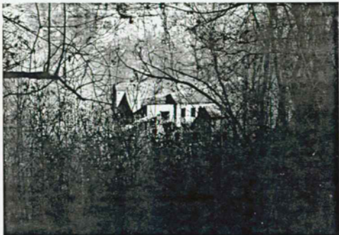
Figure 17 Coal Tipple west elevation. View from uphill on the haulage route.
