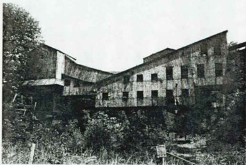
Figure 19 Coal Tipple Existing Condition Photograph: North elevation. July 1996. NPS photo.
