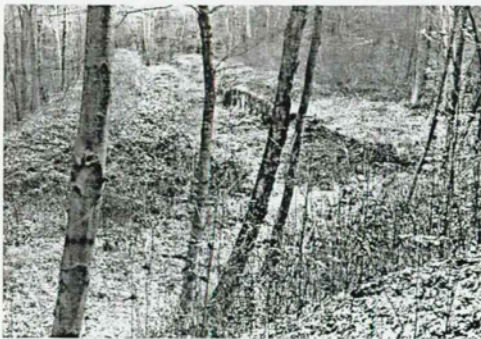
Figure 30 Coke Ovens Existing Condition Photo: Double battery of coke ovens. Vegetation partially cleared in between. July 1996. NPS photo.
