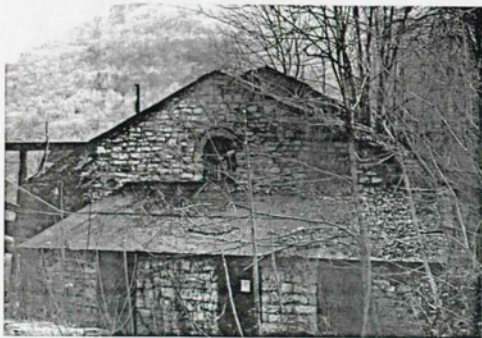
Figure 24 Powerhouse Existing Condition Photo: North elevation. Roof over generator room in the foreground. Nov. 1996. NPS photo.
