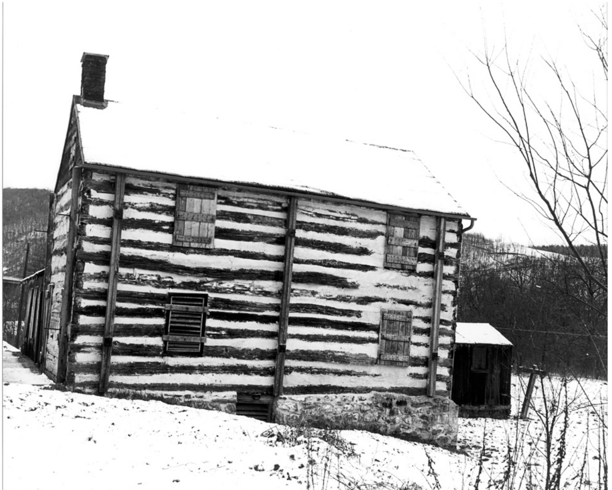
Illustration 2 Lockhouse of log construction, 1967 photograph. From National Park Service Files, Department of the Interior
