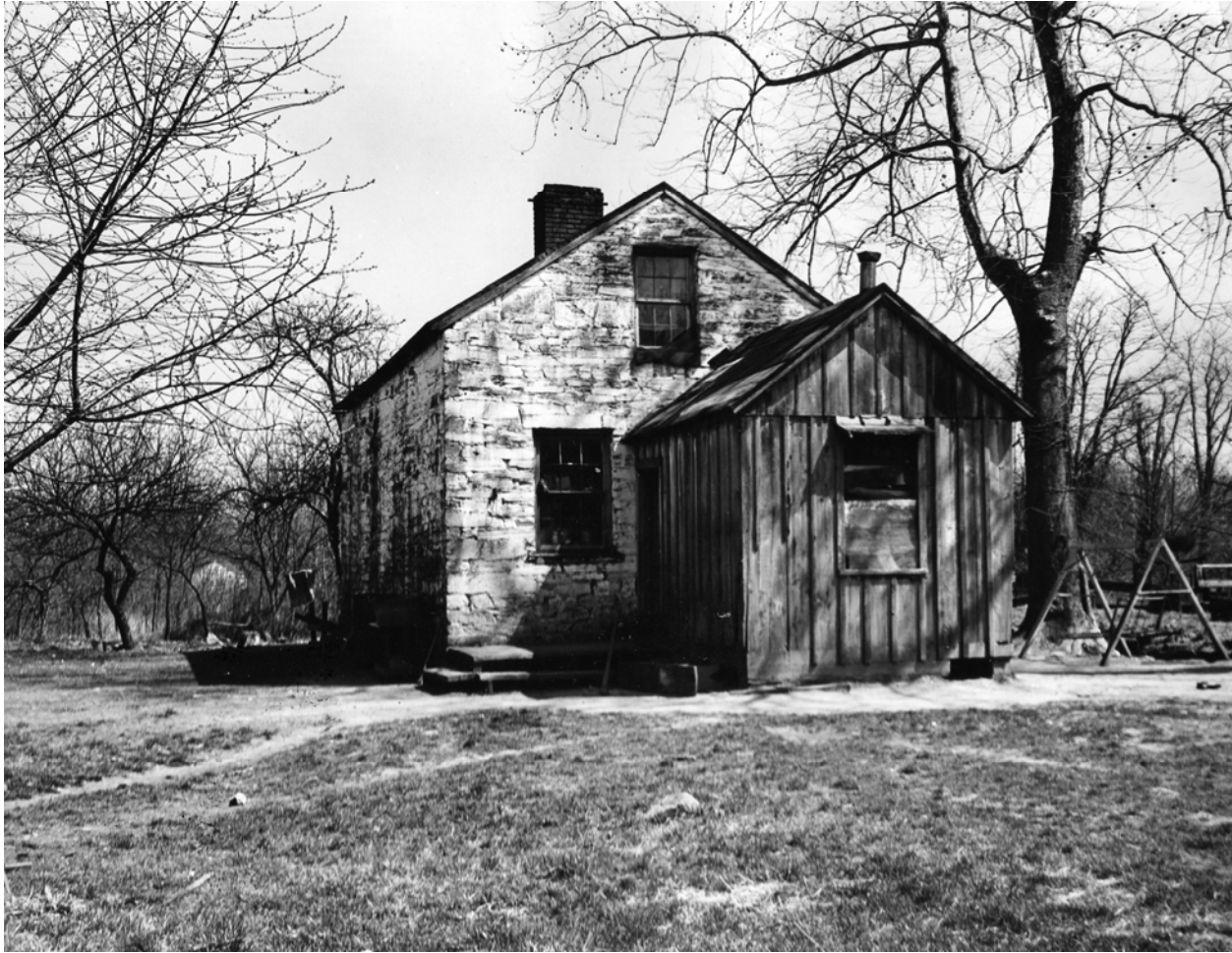
Illustration 5 House at Lock No. 13, ca. 1936 photograph. From C & O Canal NHP Files.
