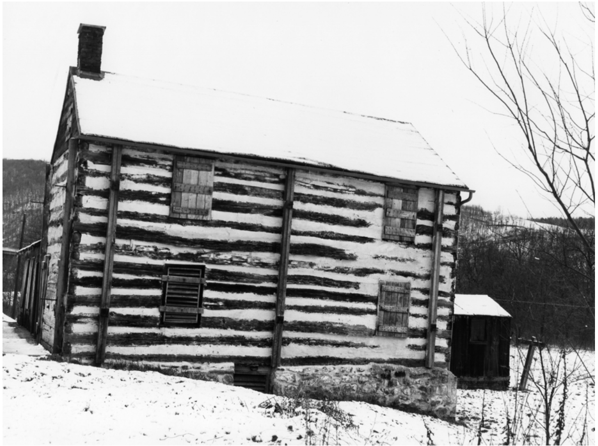
Illustration 26 House at Lock No. 75, right side view. Note 3 vertical braces, Prior to 1978 restoration.
