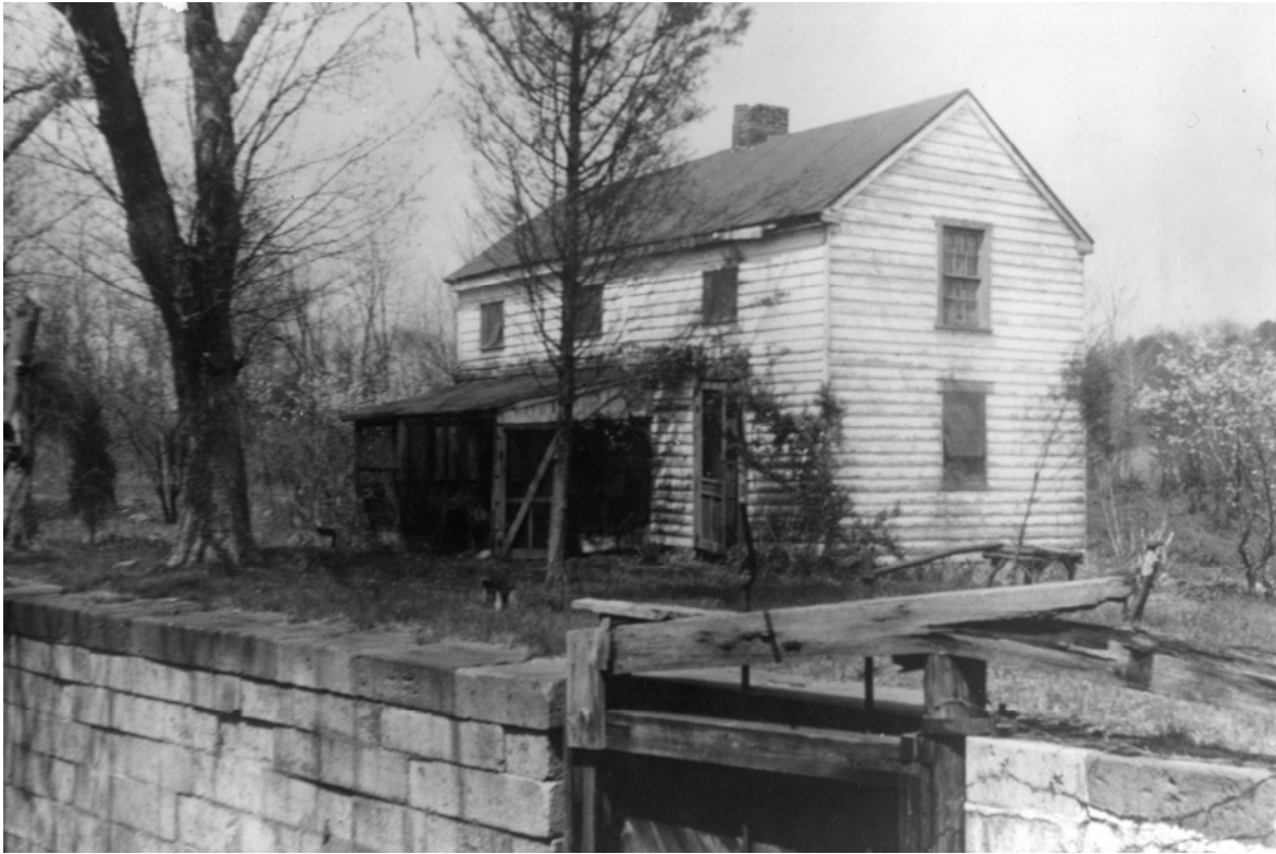
Illustration 4 House at Lock No. 12, ca. 1936 photograph. From C & O Canal NHP Files.
