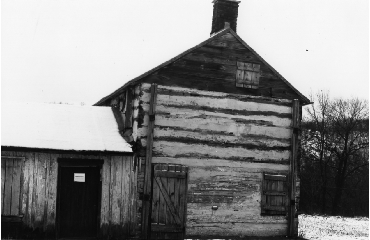
Illustration 25 House at Lock No. 75, 1967 photograph. Photograph by Hugo Skrastins. From National Park Service Files, Department of the Interior.
