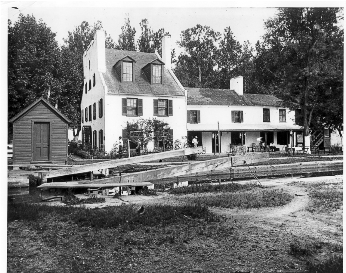
Illustration 6 Great Falls Tavern (Crommelin House), ca. 1900 photograph. showing group of men standing on porch. From C & O Canal NHP Files.
