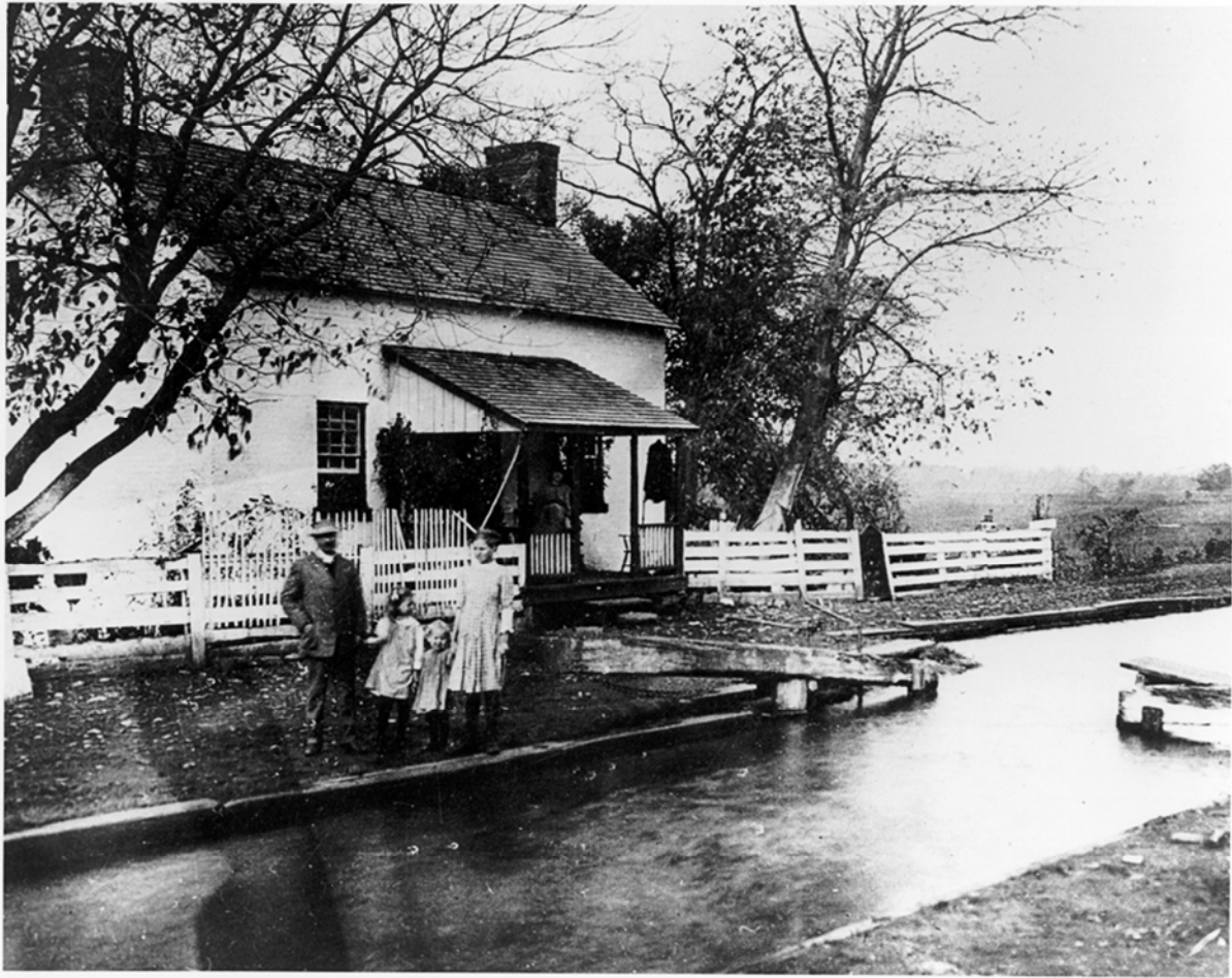
Illustration 1 Unidentified lockhouse with family standing in front, ca. 1900 photograph. National Park Service Files, National Archives.
