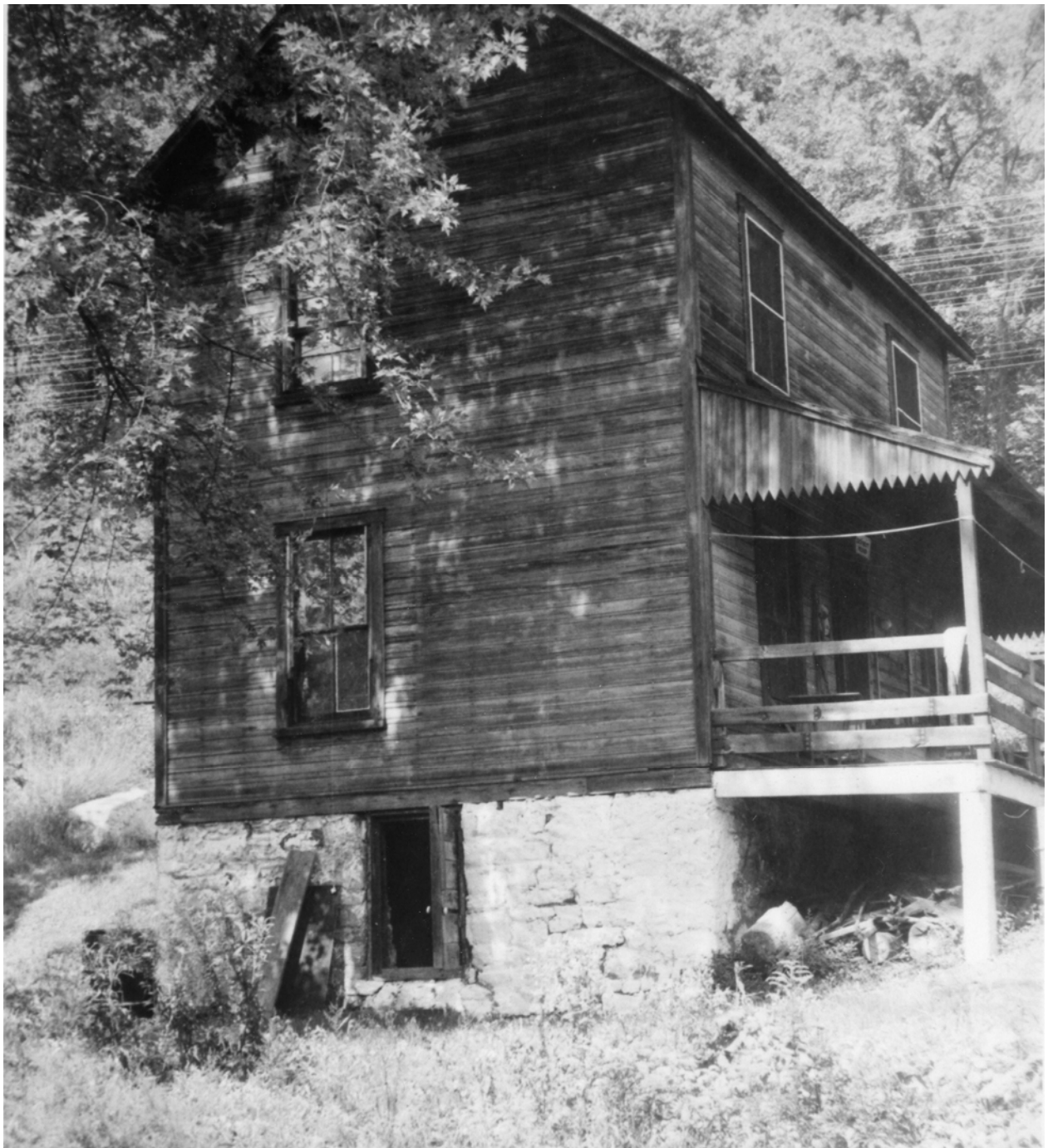
Illustration 23 House at Lock No. 54, rear and northwest elevations, Jan. 1960 photograph. Photograph by Jack E. Boucher. From Historic American Buildings Survey Files.
