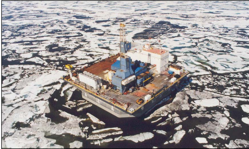
Concrete Island Drilling System (CIDS), a bottom-founded Arctic structure originally used for exploration wells in the U.S. Beaufort Sea and now serving as the base for ExxonMobil's Orlan production structure in the Sakhalin 1 development. (Photo courtesy of David Dickins, DF Dickins Associates, Ltd.)
