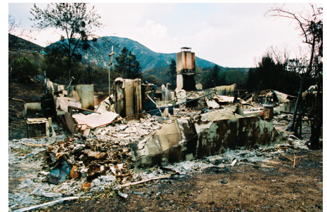
A wildfire left very little of this home near San Bernardino, Calif., in October 2003. (FEMA photo/ Kevin Galvin)
